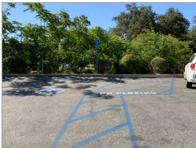
OVERVIEW OF ACCESSIBLE PARKING AREA
