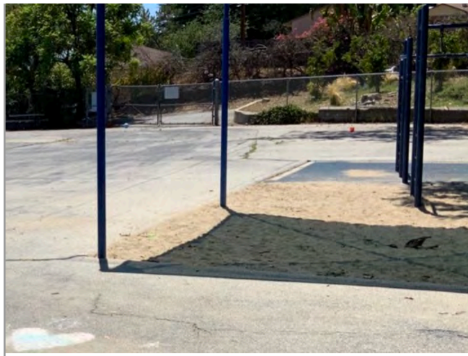
ACCESSIBLE ROUTE TO PLAYGROUND
