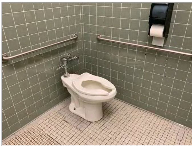
TOILET STALL OVERVIEW
