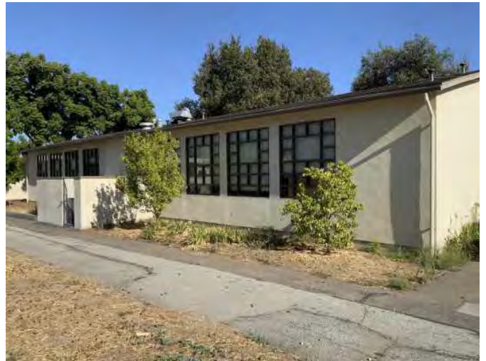
16 - BUILDING Q - LEFT/REAR ELEVATION
