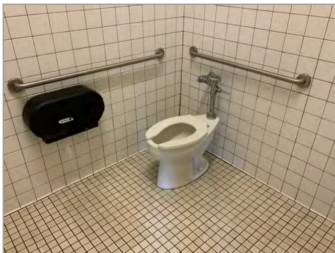
TOILET STALL OVERVIEW
