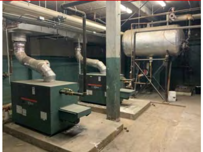
38 - BUILDING A BOILER ROOM
