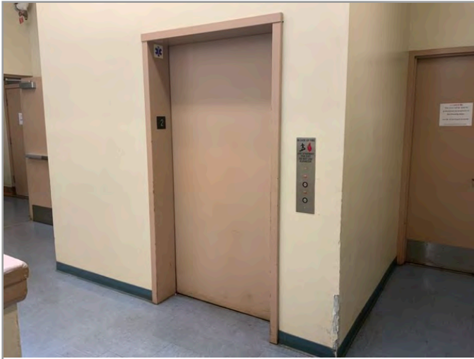
LOBBY LOOKING AT CAB BUILDING A
