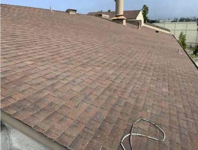
31 - ASPHALT SHINGLE ROOFING
