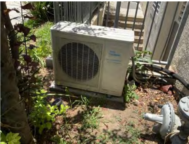
57 - DUCTLESS SPLIT SYSTEM COMPONENT
