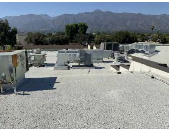
29 - MODIFIED BITUMEN ROOFING
