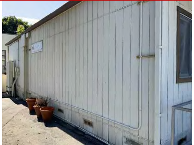
26 - EXTERIOR PAINTED WOOD PANELING
