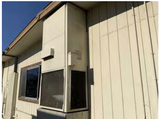
58 - WALL-MOUNTED HEAT PUMP
