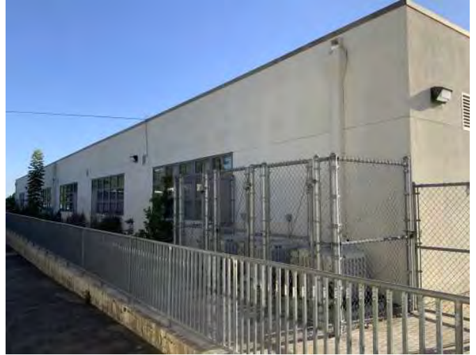
14 - BUILDING P - LEFT/REAR ELEVATION
