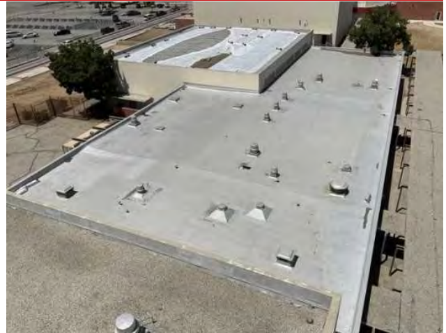
14 - PRIMARY ROOF OVERVIEW
