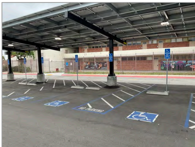
OVERVIEW OF ACCESSIBLE PARKING AREA
