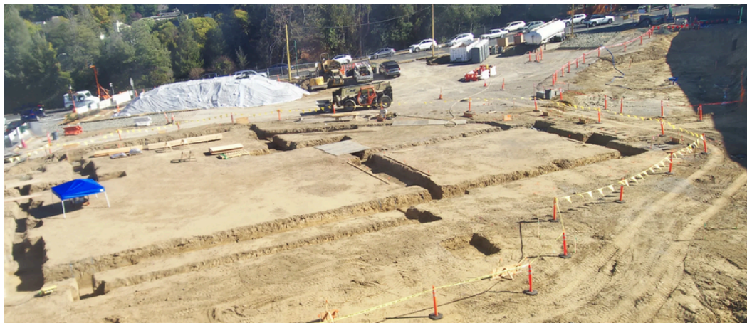
Pictured above : Grading for the building pad
