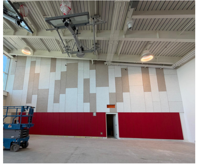
Pictured above : Acoustic Panels have been installed
