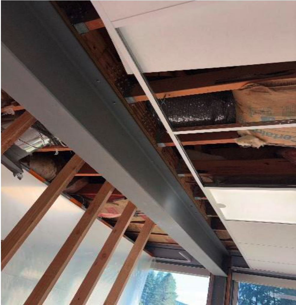
Installation of beam at Walterville
