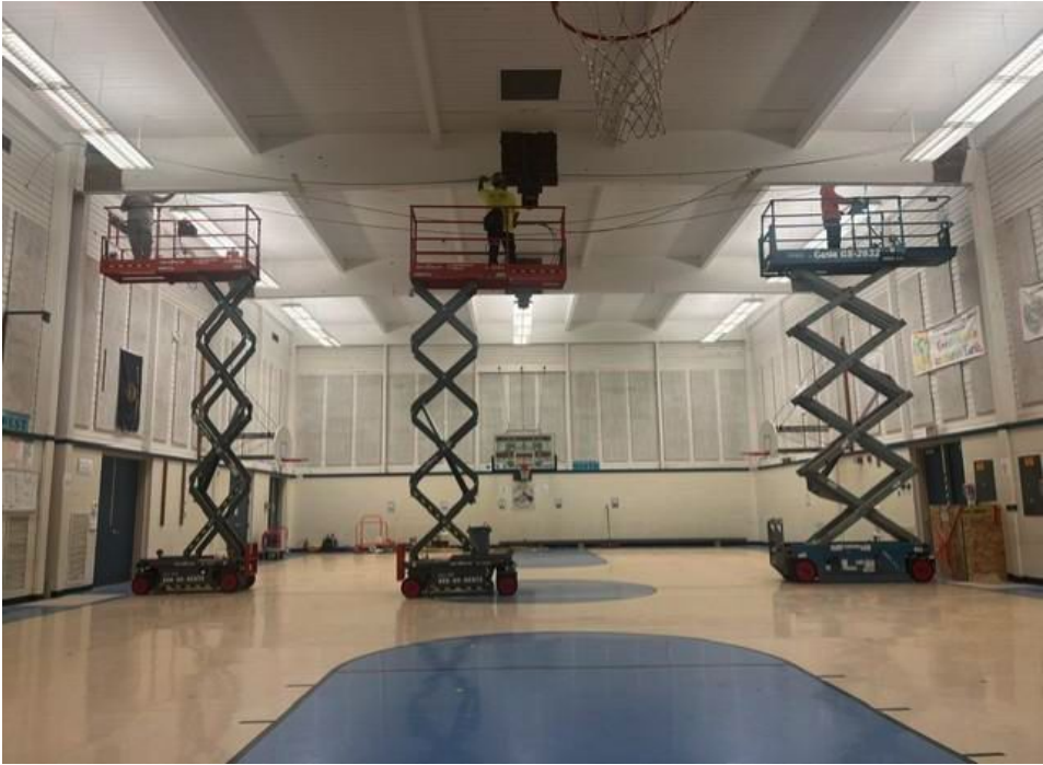
Stringing tensioning cables at Centennial
