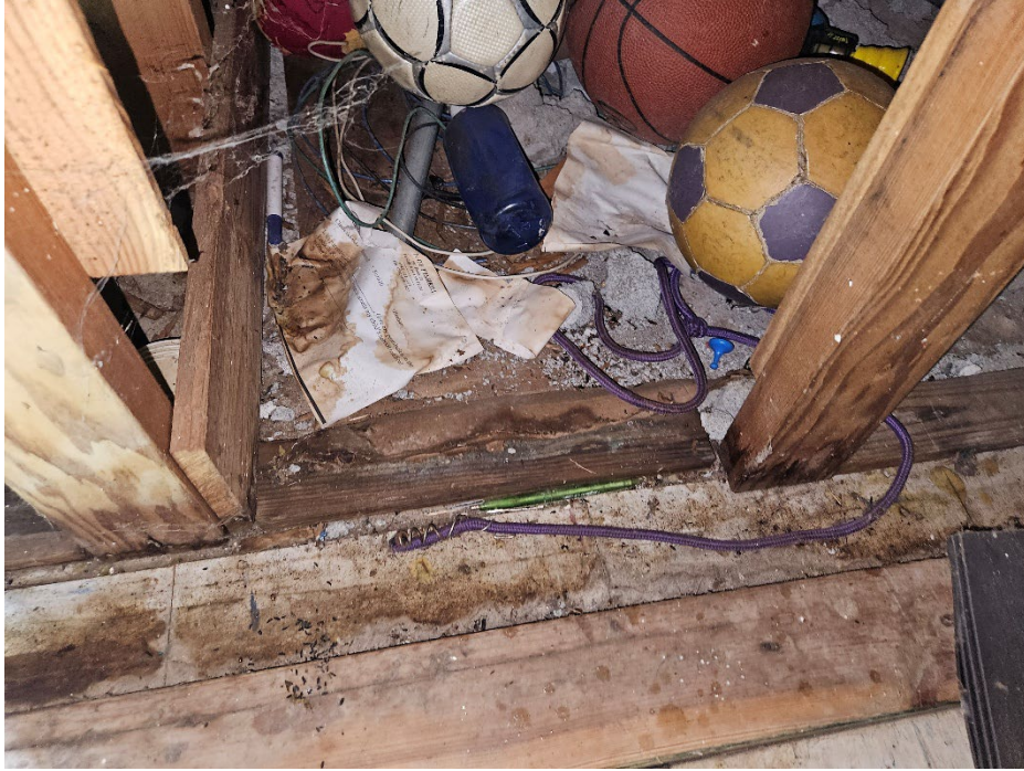
Photograph 3, Under Stage Stair
