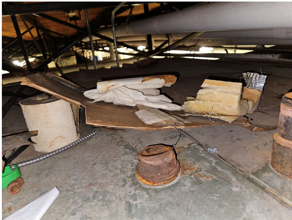
Photograph 4, Top of Second Air Handler
