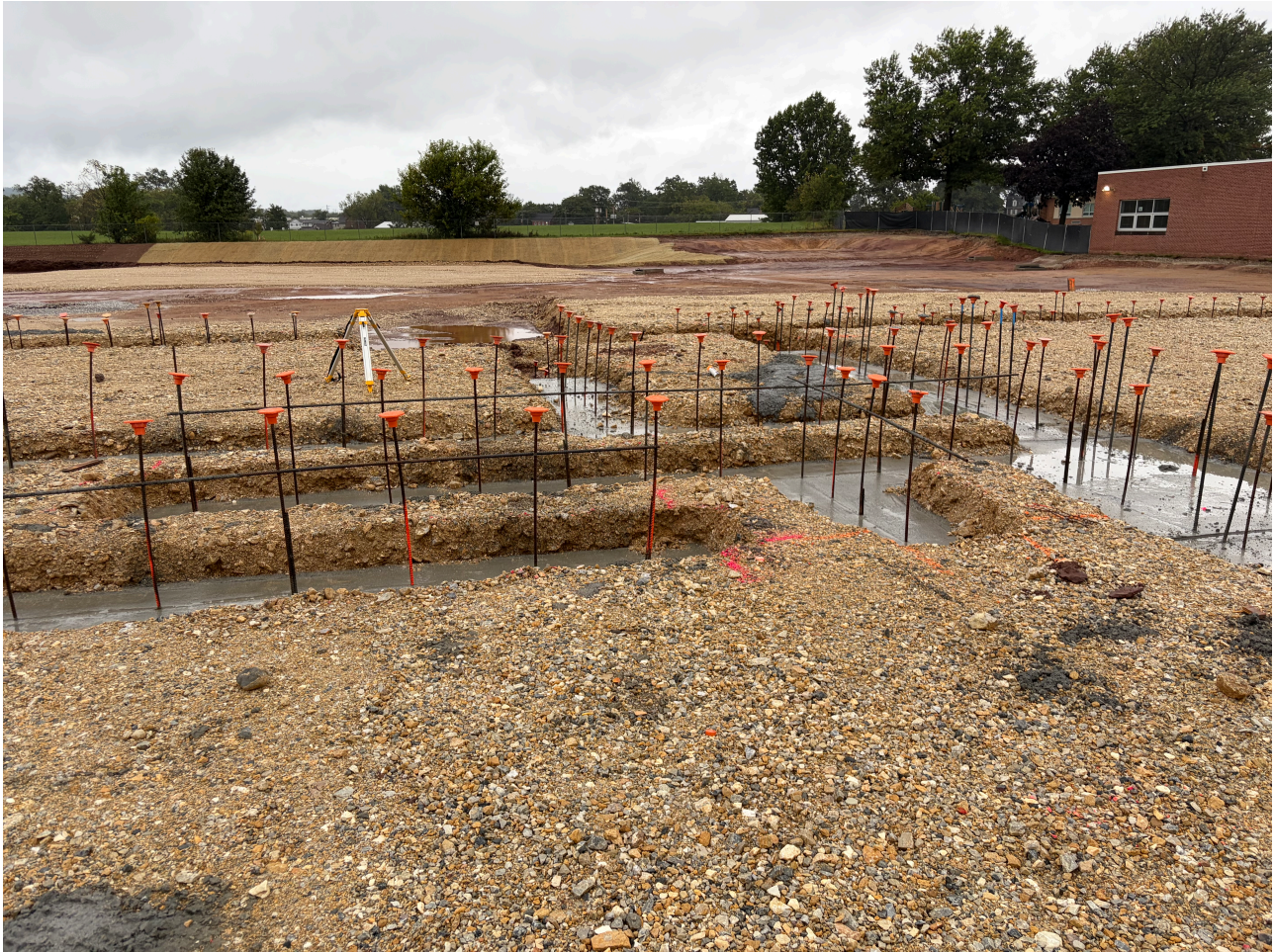
Interior Footers Area C (2)
