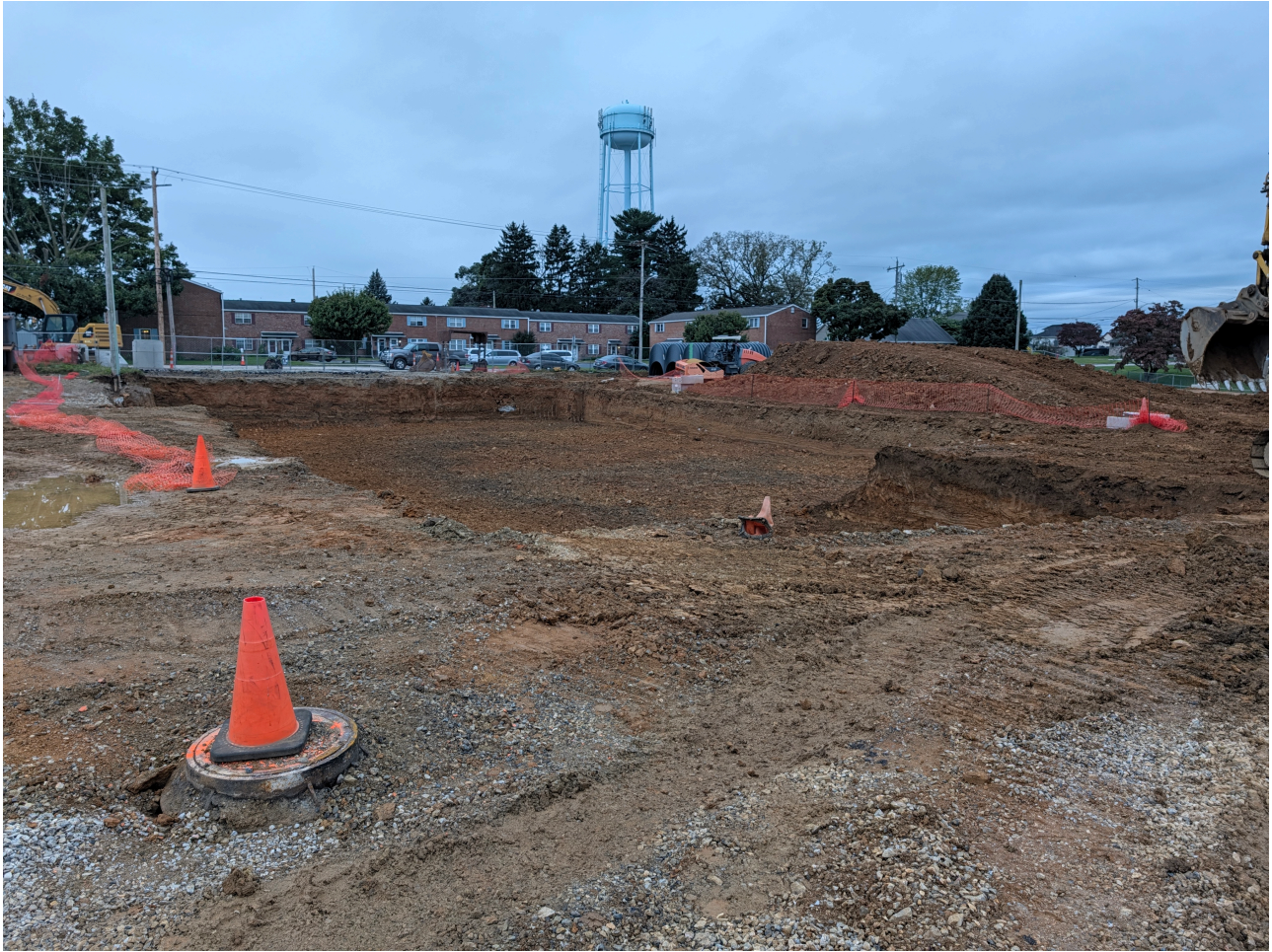
Storm Basin Excavation
