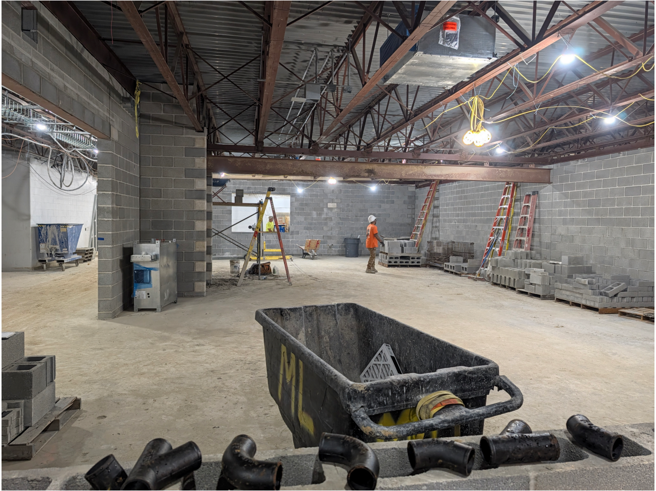
New CMU Walls Area C
