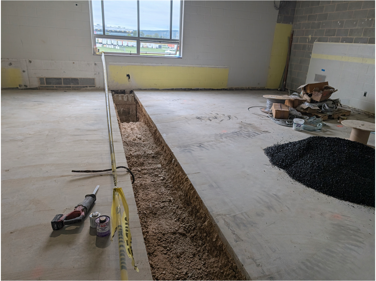
Underground Sanitary Lines in Classrooms Area C
