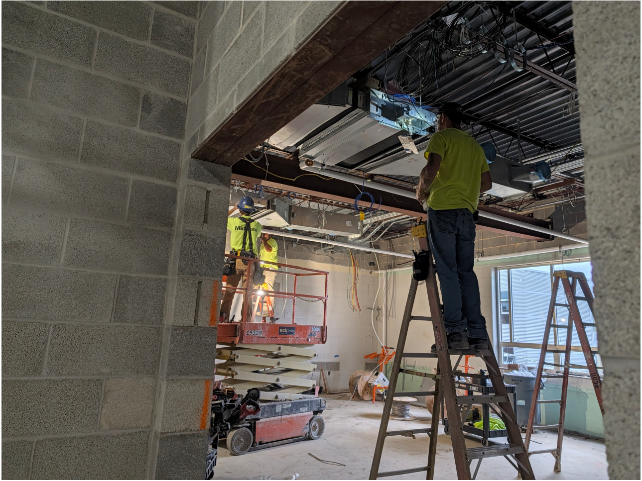
Classroom Units Installed
