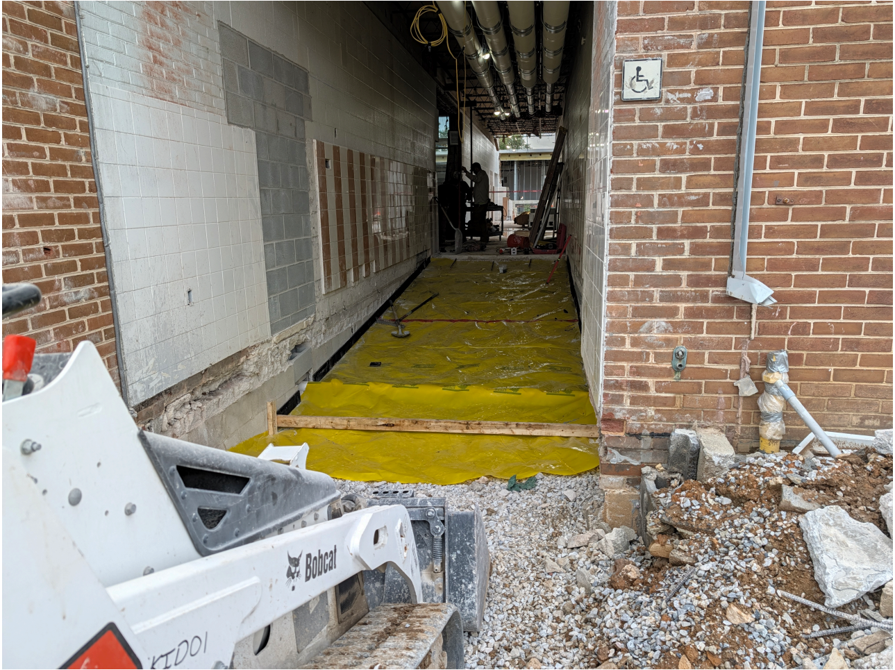
New Concrete Ramp Area A
