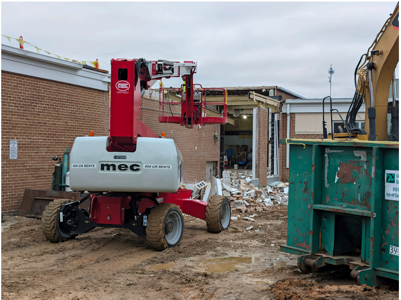
Bulk Building Demo Progress (1)
