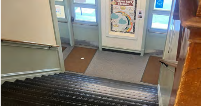
Interior stairs required to reach main office
