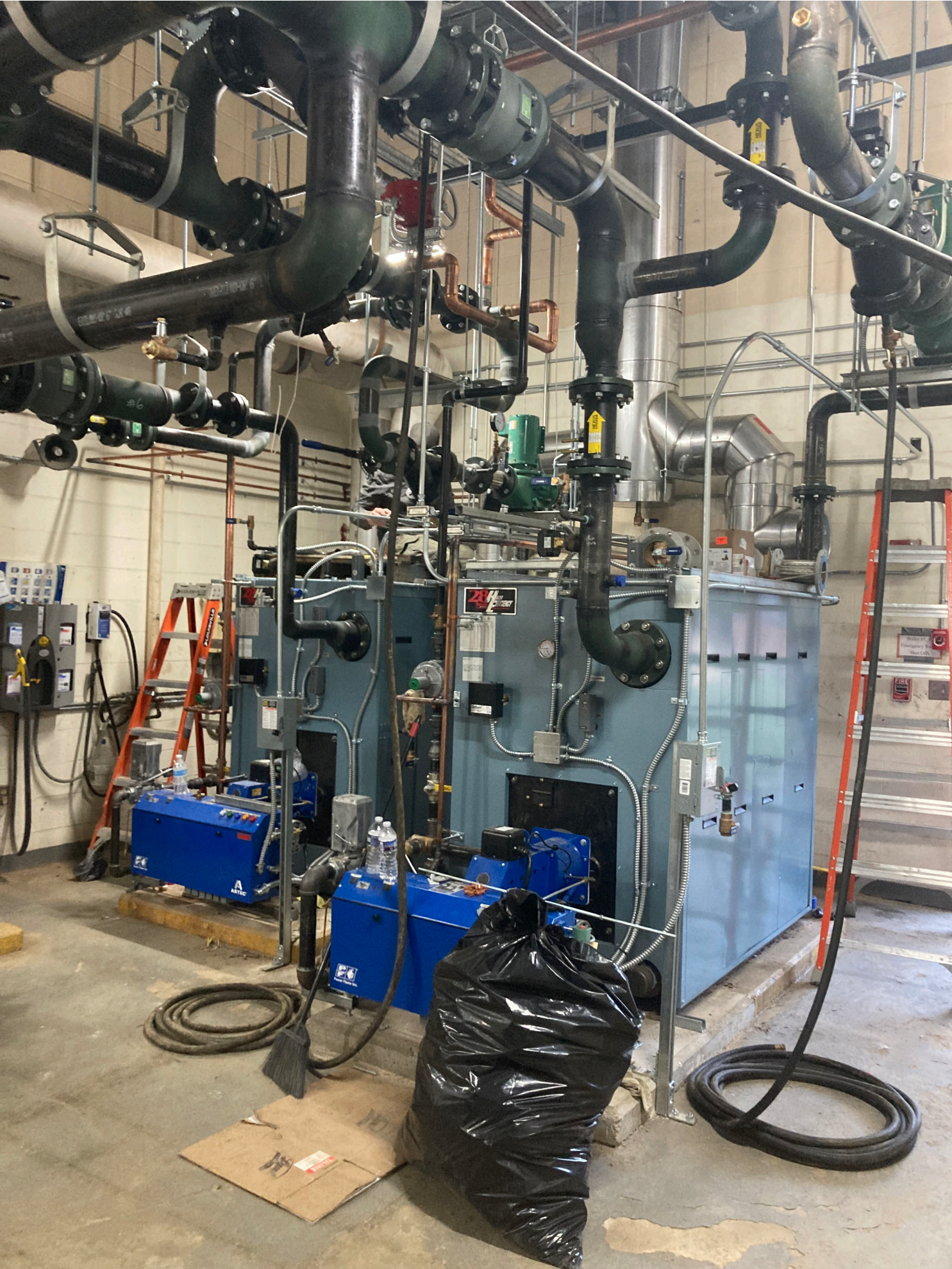
CECIL MANOR ELEMENTARY SCHOOL – HVAC REPLACEMENT
