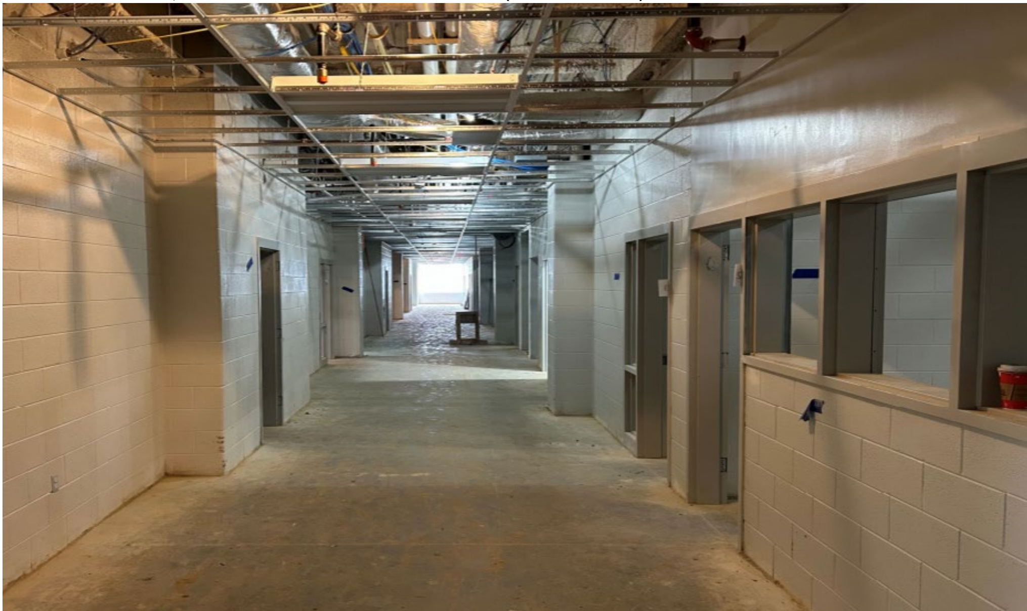
NORTH EAST MIDDLE / HIGH SCHOOL – REPLACEMENT – AREA C (MIDDLE SCHOOL) CORRIDOR
