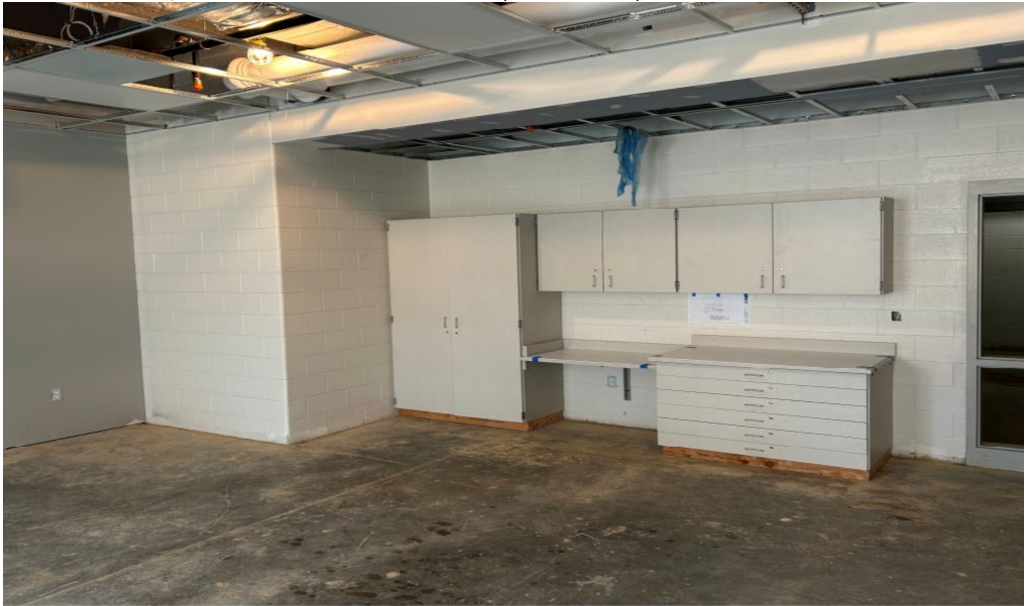
NORTH EAST MIDDLE / HIGH SCHOOL – REPLACEMENT – AREA C (MIDDLE SCHOOL) TYPICAL CLASSROOM
