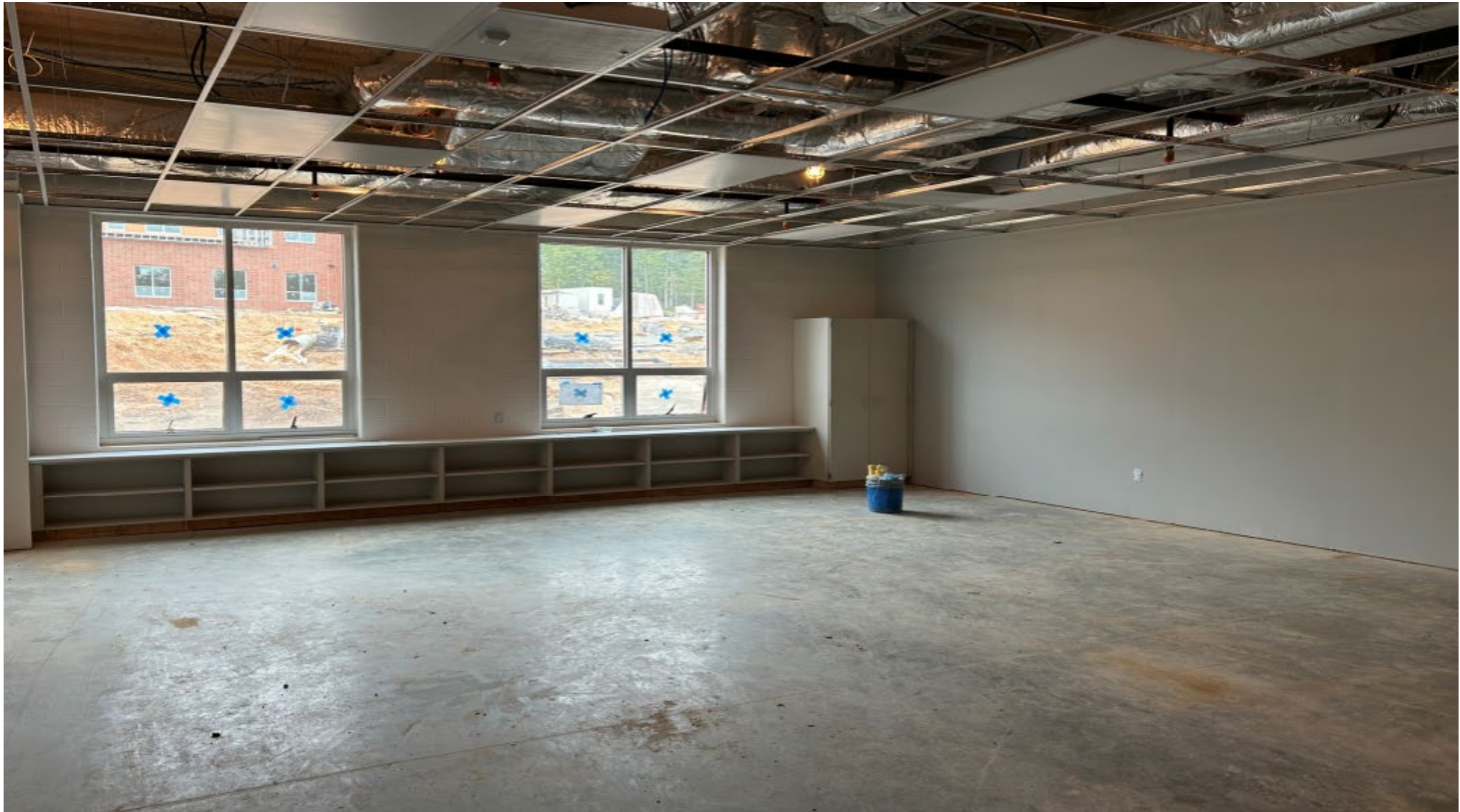
NORTH EAST MIDDLE / HIGH SCHOOL – REPLACEMENT – AREA C (MIDDLE SCHOOL) TYPICAL CLASSROOM
