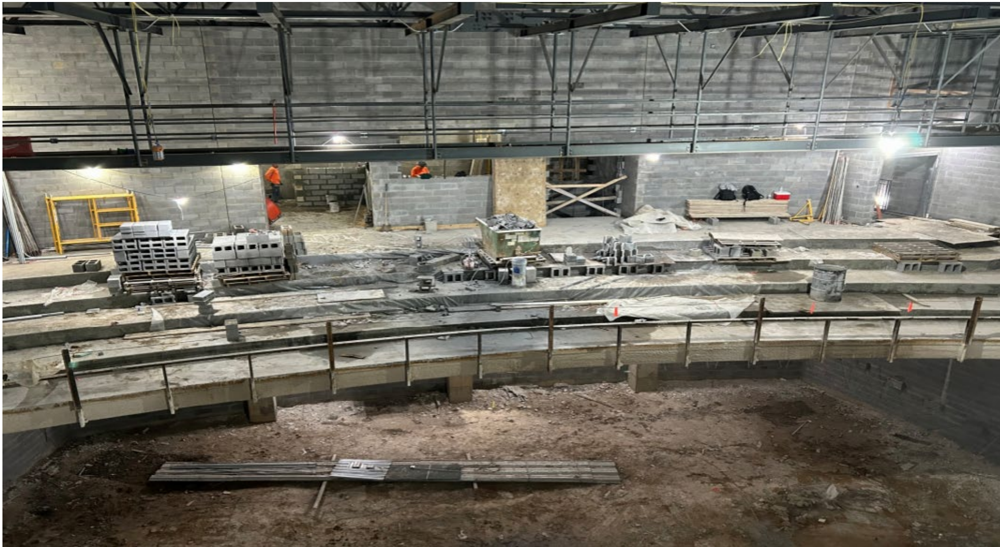
NORTH EAST MIDDLE / HIGH SCHOOL – REPLACEMENT – AUDITORIUM BALCONY
