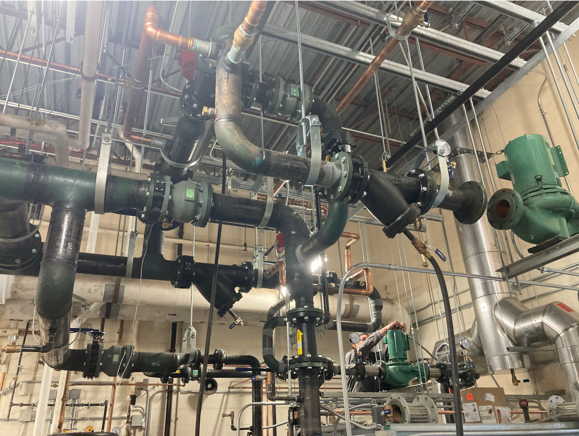
CECIL MANOR ELEMENTARY SCHOOL – HVAC REPLACEMENT
