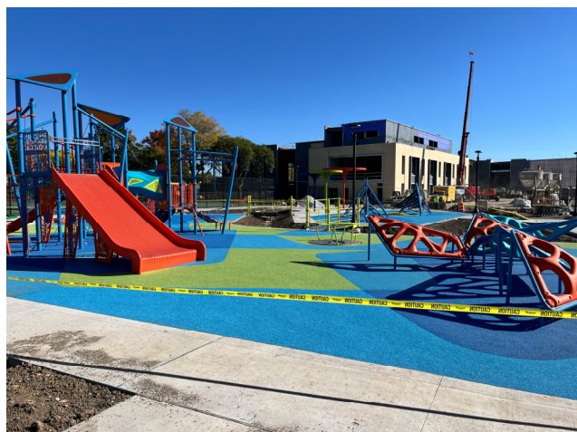
Pour In Place Surface Completed – Site Playground
