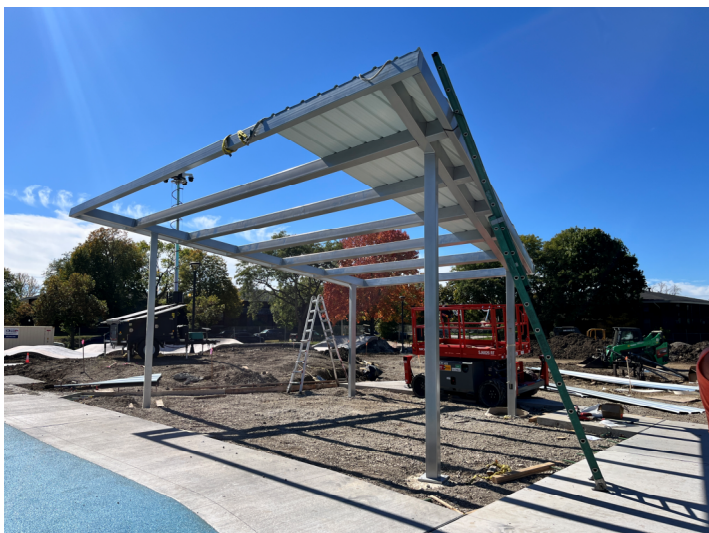
Monoslope Install Ongoing – Site West Of Playground
