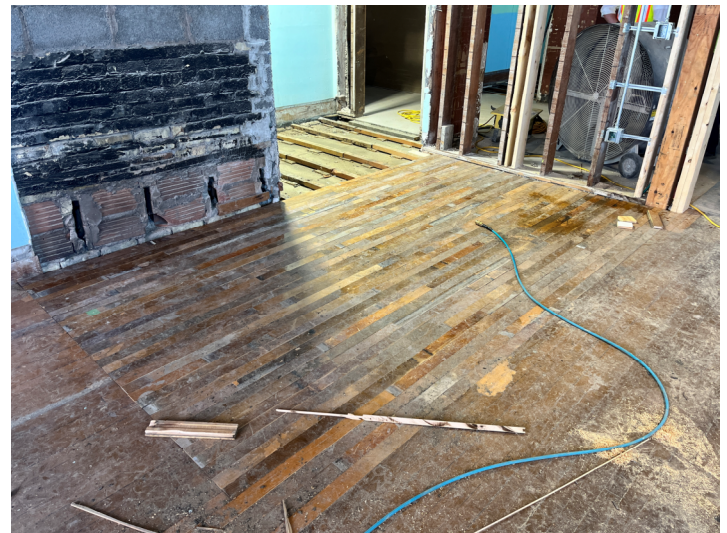
Wood Floor Patching – Area A1 3 rd Floor Classrooms
