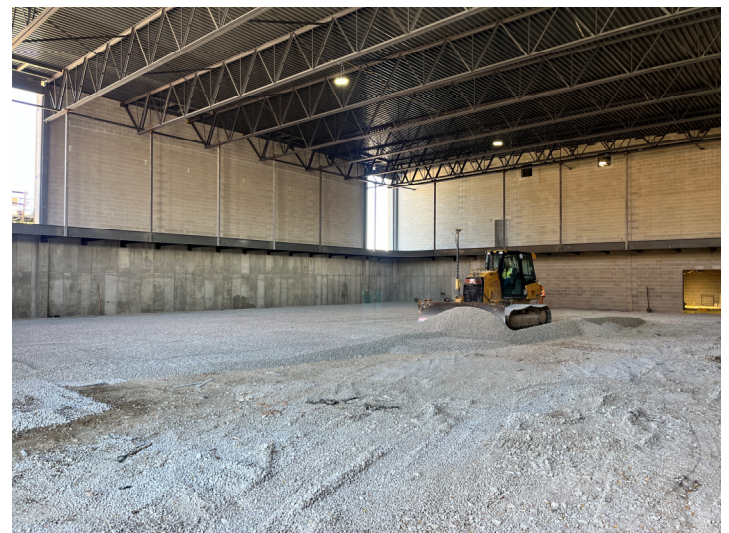
Stone/Prep Floor – Area C2 Gymnasium
