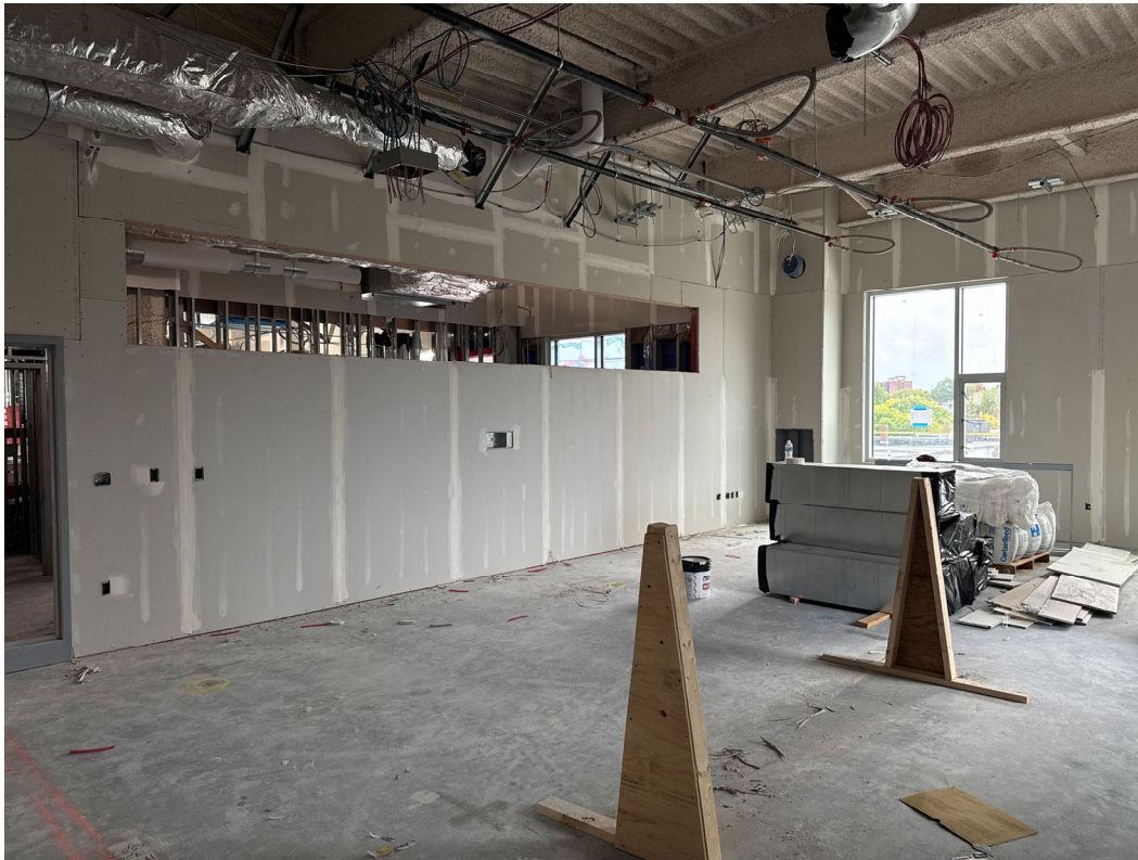
September 29: Interior walls inspected and drywalled
