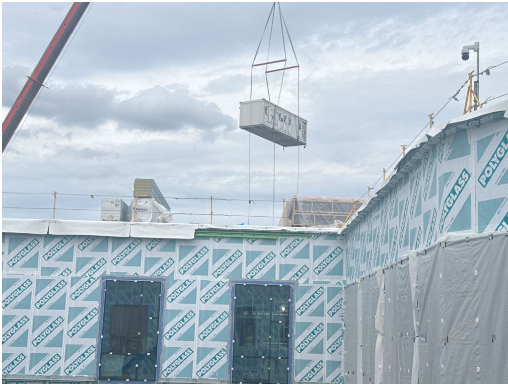
September 09: Roof top unit craned onto roof
