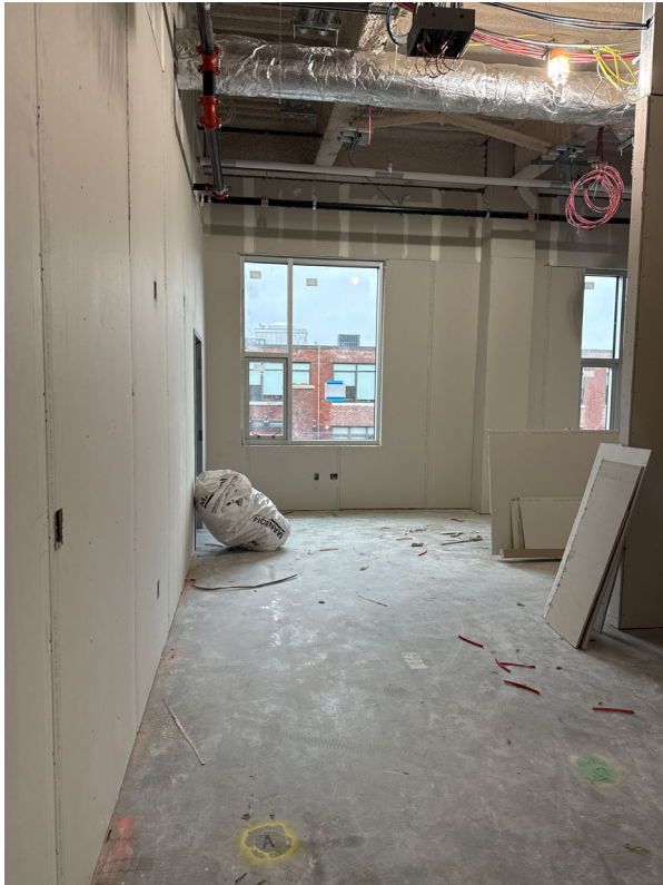
September 29: Interior walls inspected and drywalled
