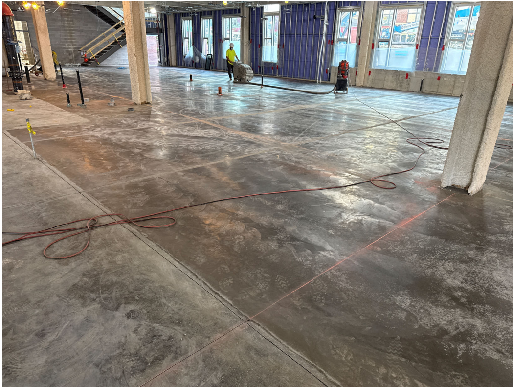
September 10: Topping slab placed, Level 1
