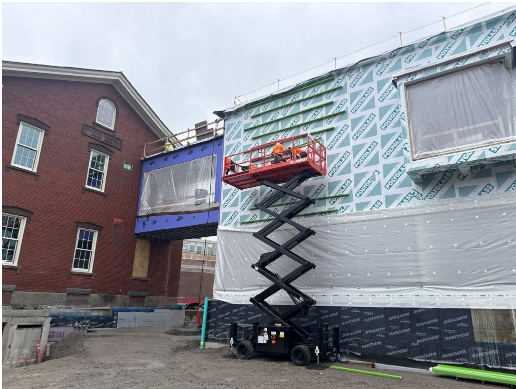
September 30: Prep for slate on Building B East; sheathing on bridge to Historic Bldg.
