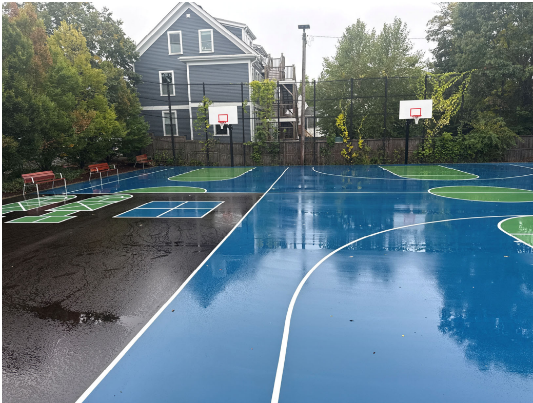
September 30: Basketball court sealed/painted/stripped
