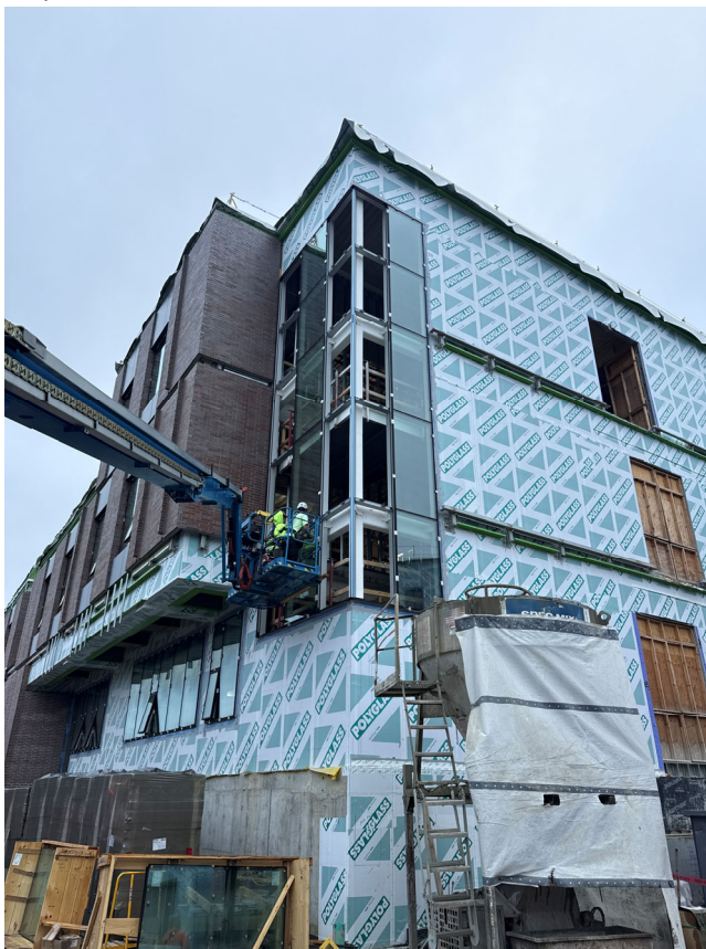
September 21: NW corner, brick, glazing
