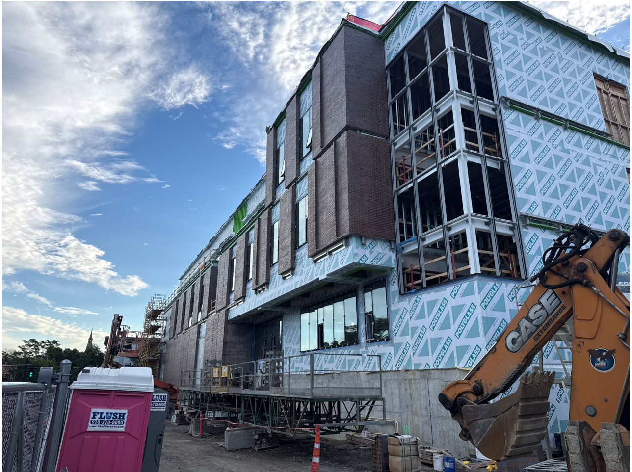
September 08: West elevation Bldg A
