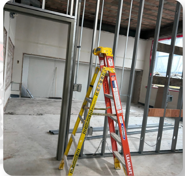
Steel stud framing for drywall partitions
