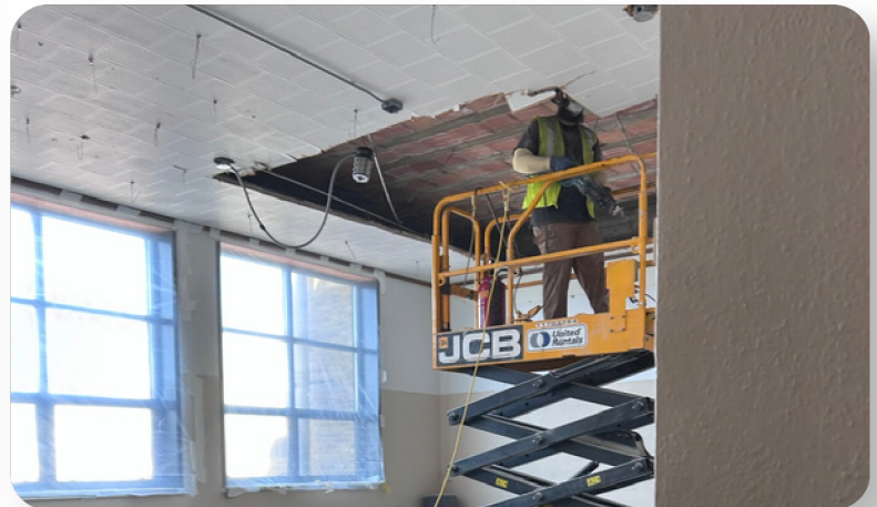
Plaster ceiling demolition
