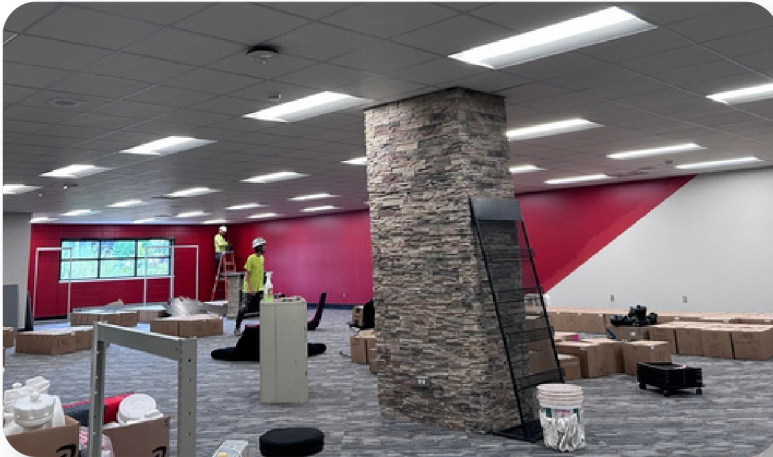
Library Media Center renovation
