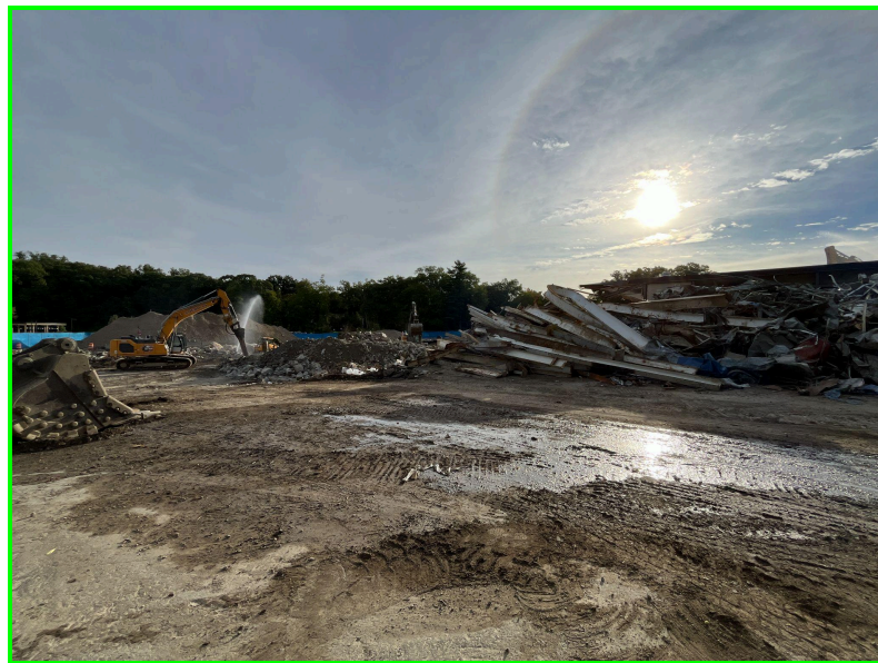
Demolition of the Existing Middle School Continues, and Crews Are Sorting and Removing Materials
