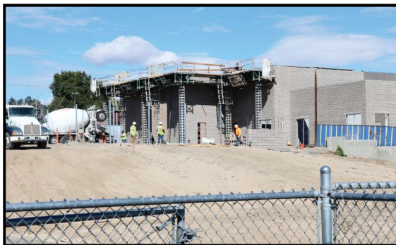
Progress continues at the Wilbur Repp CTE center on the campus of Selah High School.
