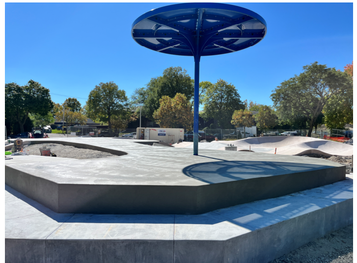
Spectating Area Concrete Poured – Site Pump Track
