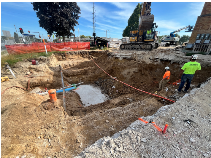
Water Meter Excavation – Site Northeast Corner
