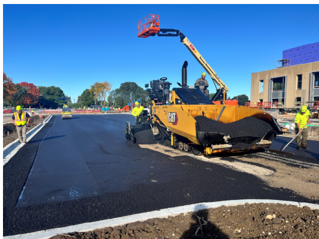
Paving – Site West Parking Lot
