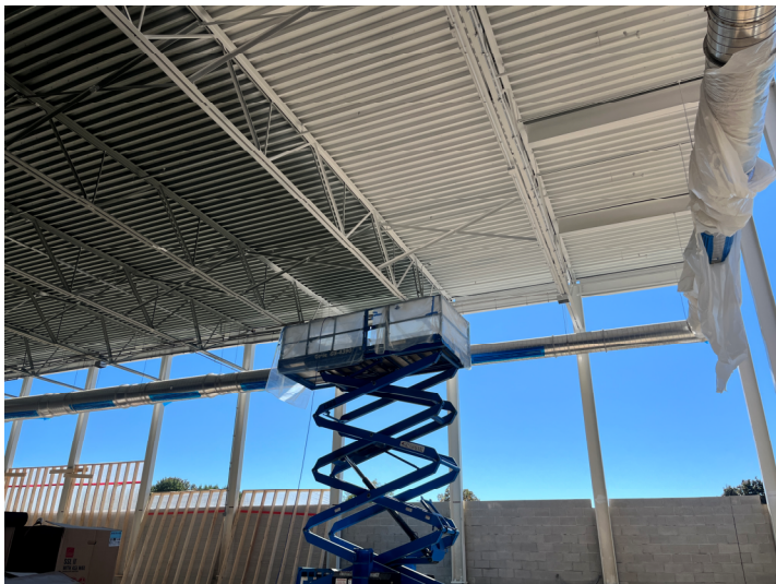
High-Performance Coating – Area B2 Natatorium
