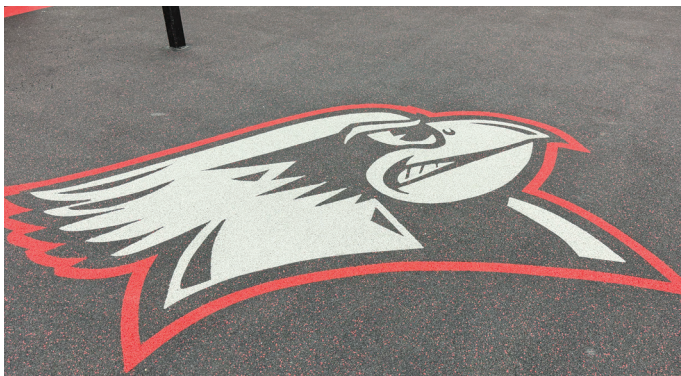
Weight Room Flooring
