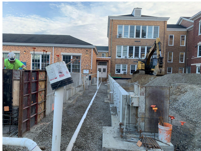
Corridor walls with sanitary line
