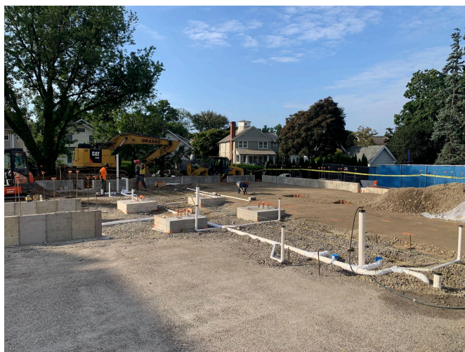
Underground plumbing installed for new addition
