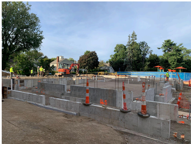
Stone installation in preparation for pouring slab
