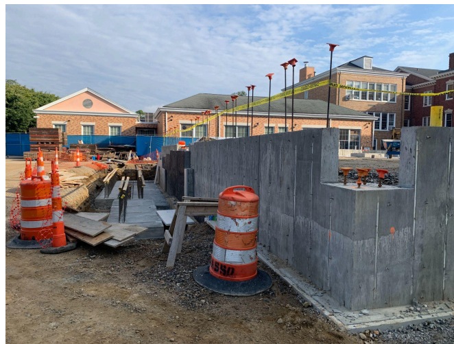
Footings for new stair/ramp out to playground and fields
