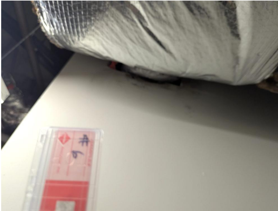
Photo 10. Mechanical/storage room. Tape sample 6 collection location, wall under the duct.
