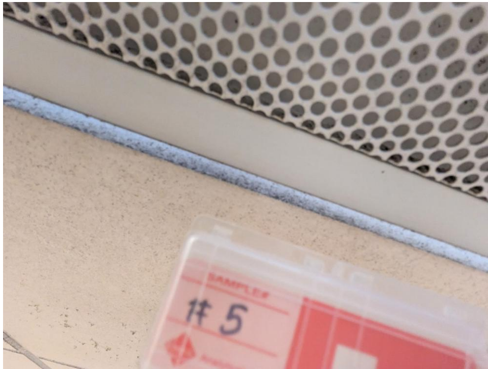
Photo 6. Room 218. Surface sample 5 collection location, ceiling tile next to the vent grille.
