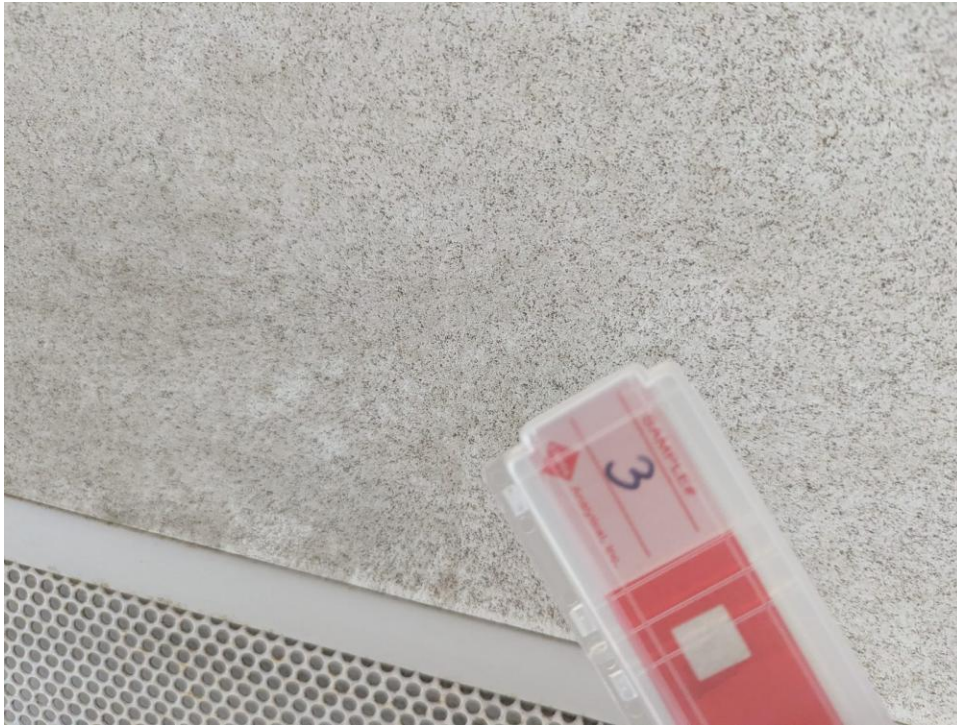
Photo 4. Room 235. Surface sample 3 collection location, ceiling tile next to the vent grille.
