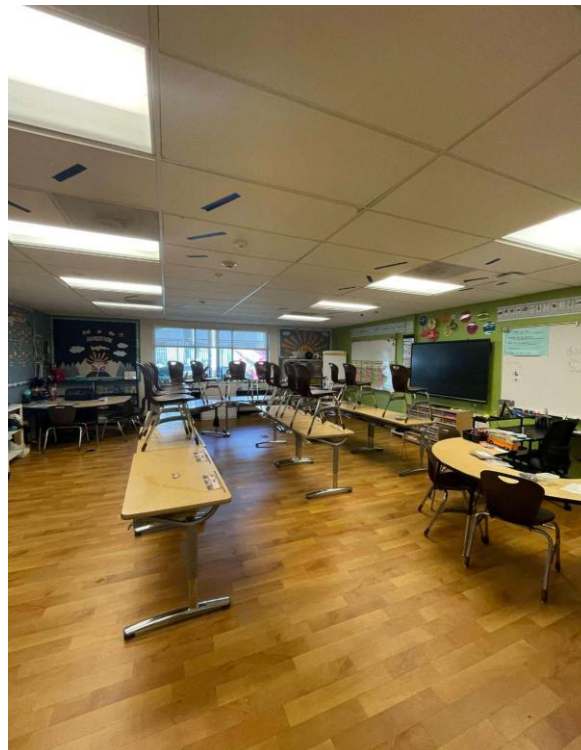
Photo 13. Classroom 131. General view.
