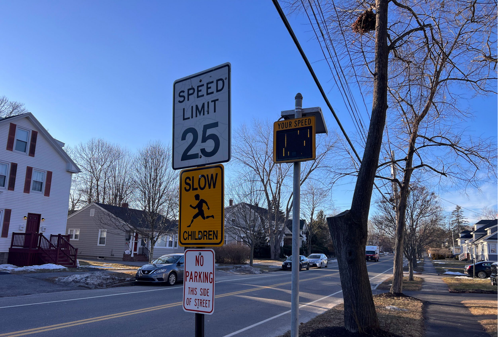
Speed feedback signs, like the one shown here on Read Street in Portland, can alert drivers to their speeds and can be useful in school zones and other areas where there are more vulnerable roadway users. Source: Neighborways Design
