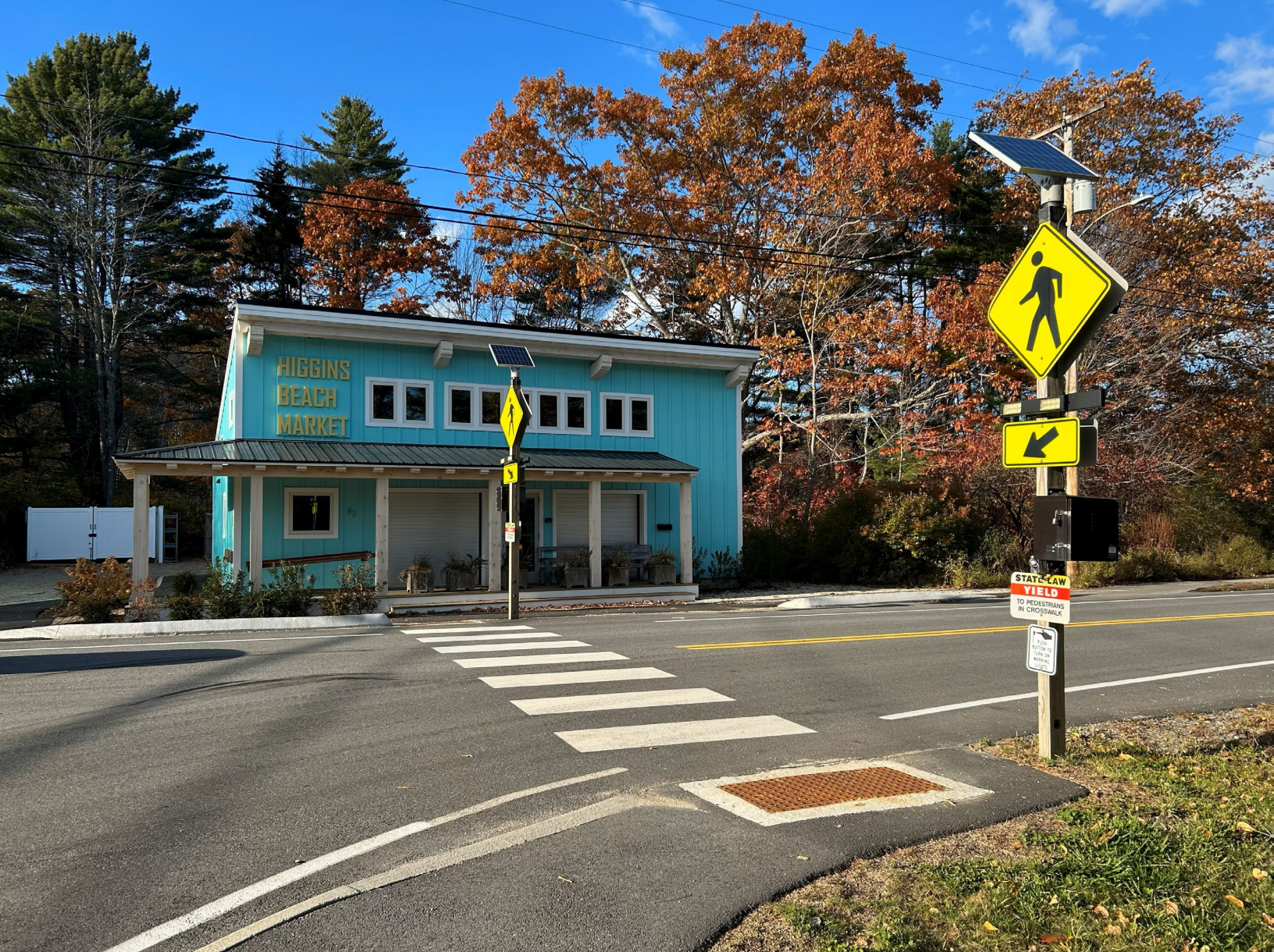
Marked crosswalk with tactile landing pad and rectangular rapid flashing beacon on Spurwink Road in Scarborough. These traffic-calming tools help improve visibility for pedestrians on rural roads where traffic volumes are higher. Source: Nelson\Nygaard
