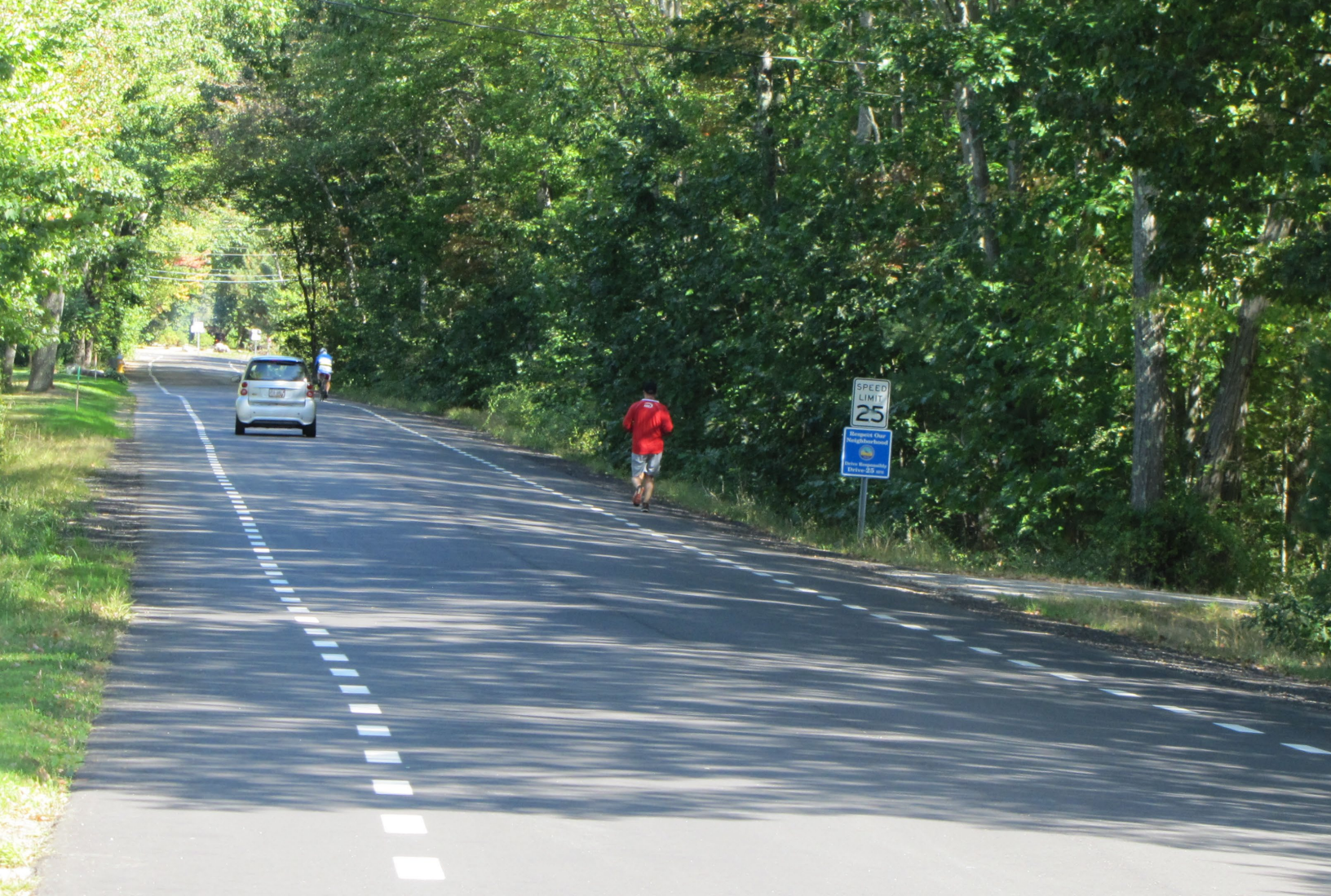
Advisory lanes like these in Scarborough can help improve safety by narrowing the traffic lanes. Source: Town of Scarborough
