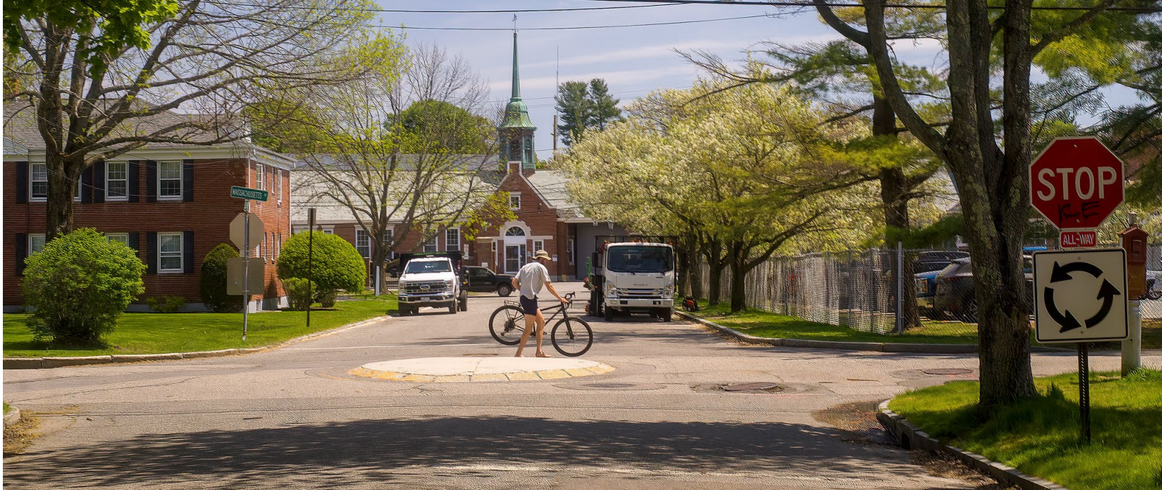
Neighborhood traffic circles, like the one shown here in Portland, ME, can provide traffic calming by encouraging slower speeds and can replace stop-controlled intersections. Source: GPCOG
