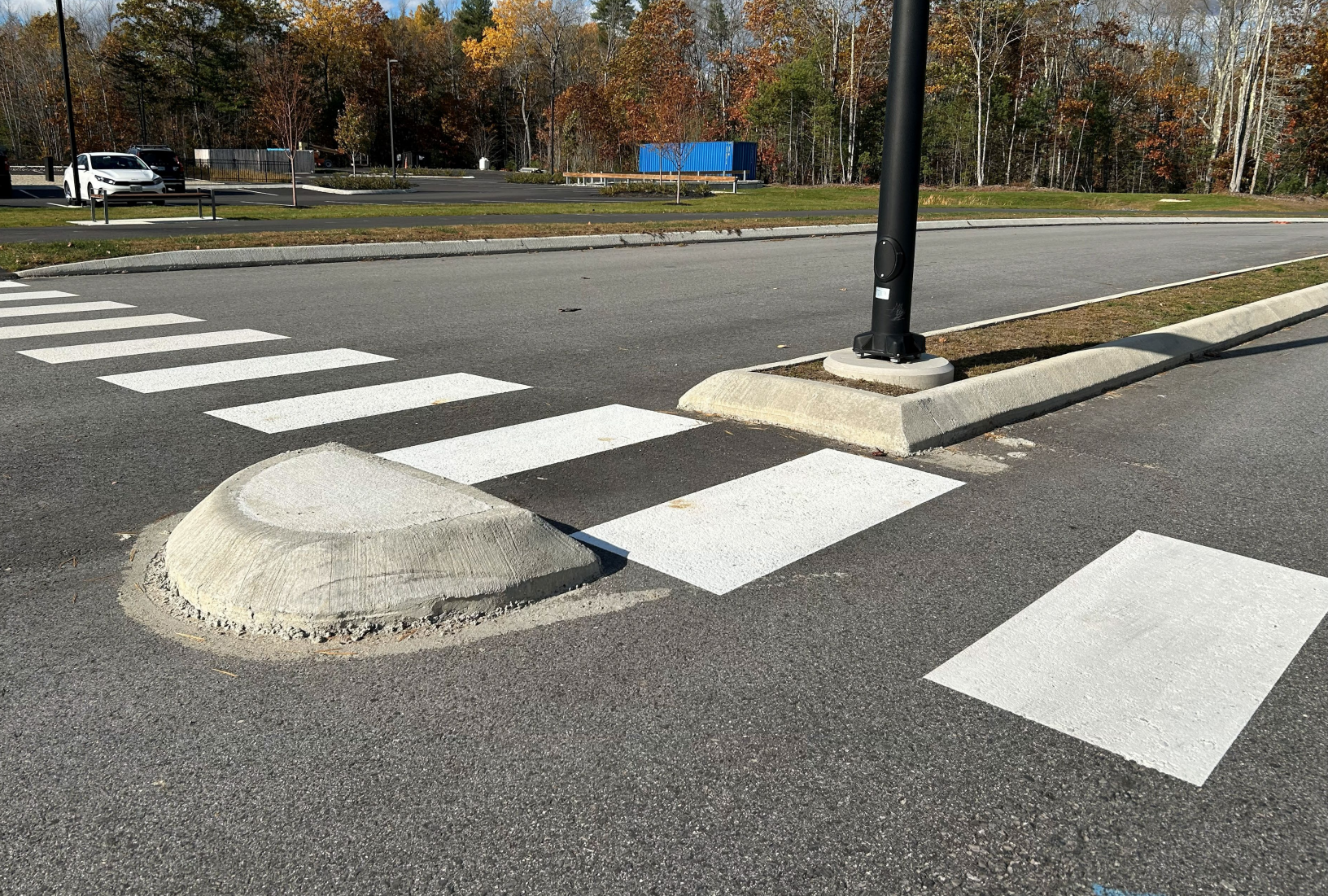
Marked crosswalks and pedestrian crossing islands, seen here on Market Street in Scarborough, provide refuge space for pedestrians while crossing. Source: Nelson\Nygaard
