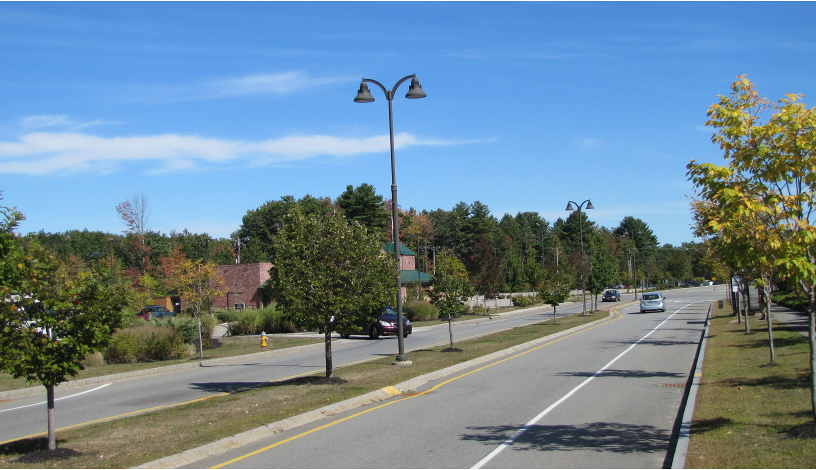
Landscaped median on Gallery Boulevard in Scarborough. This treatment can help visually narrow roadways and prevent lane departures. Source: Town of Scarborough
