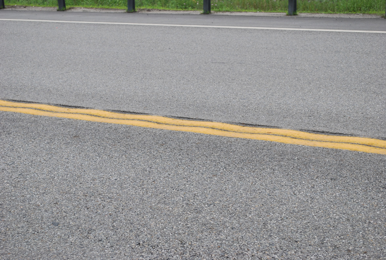
Rumble strips (shown here on Route 3 in Maine) alert drivers when they are drifting out of their lanes by creating noise and vibrations. Source: MaineDOT
