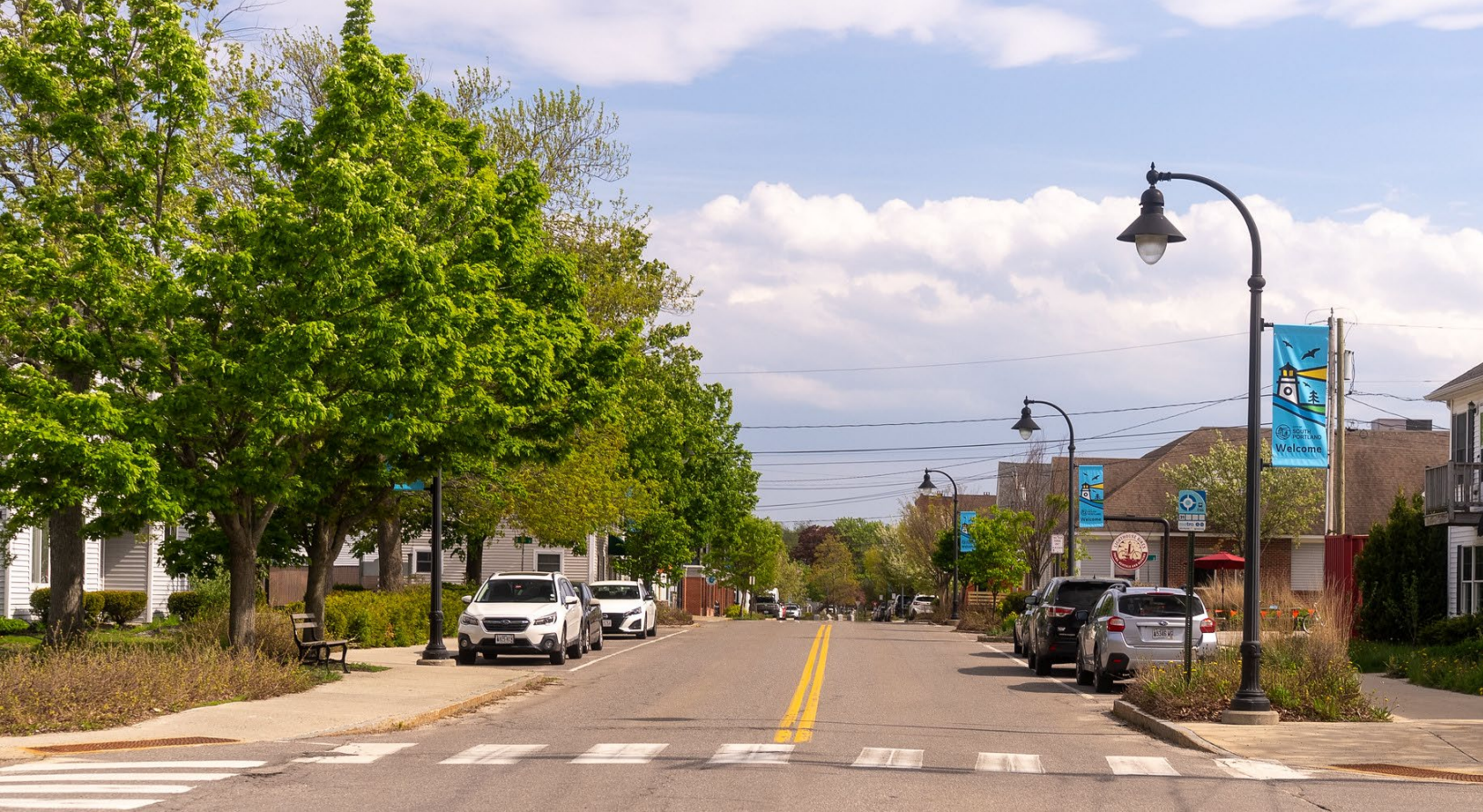
Curb extensions like these on Stevens Avenue in Portland increase visibility for pedestrians and improve safety by decreasing crossing distances. Source: GPCOG
