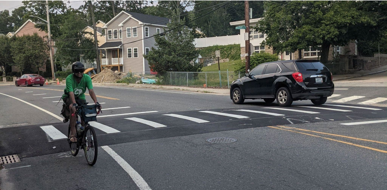
Raised crosswalk in Providence, RI. This type of treatment can slow vehicles at intersections without traffic signals. Source: Neighborways Design
