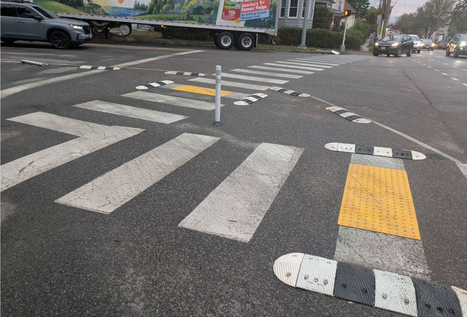
Mountable separators, shown here in Portland, help protect bike facilities and make tighter turns. Currently the Town does not install 'flex posts' due to maintenance concerns. Source: Neighborways Design
