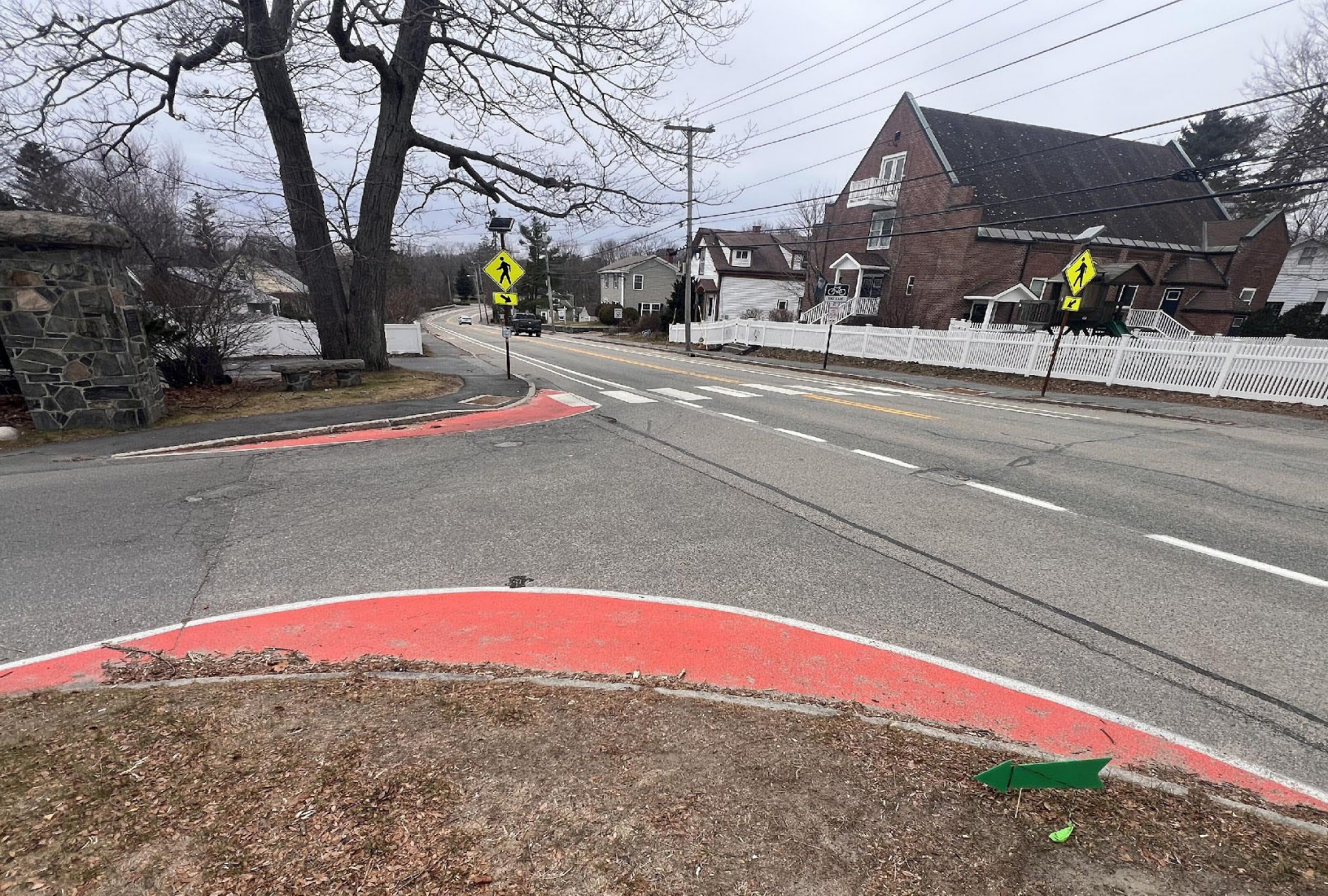
Painted bump-out, shown here in Portland, can provide a similar purpose as curb extensions on a temporary basis if permanent curb extensions are not possible. Source: Neighborways Design
