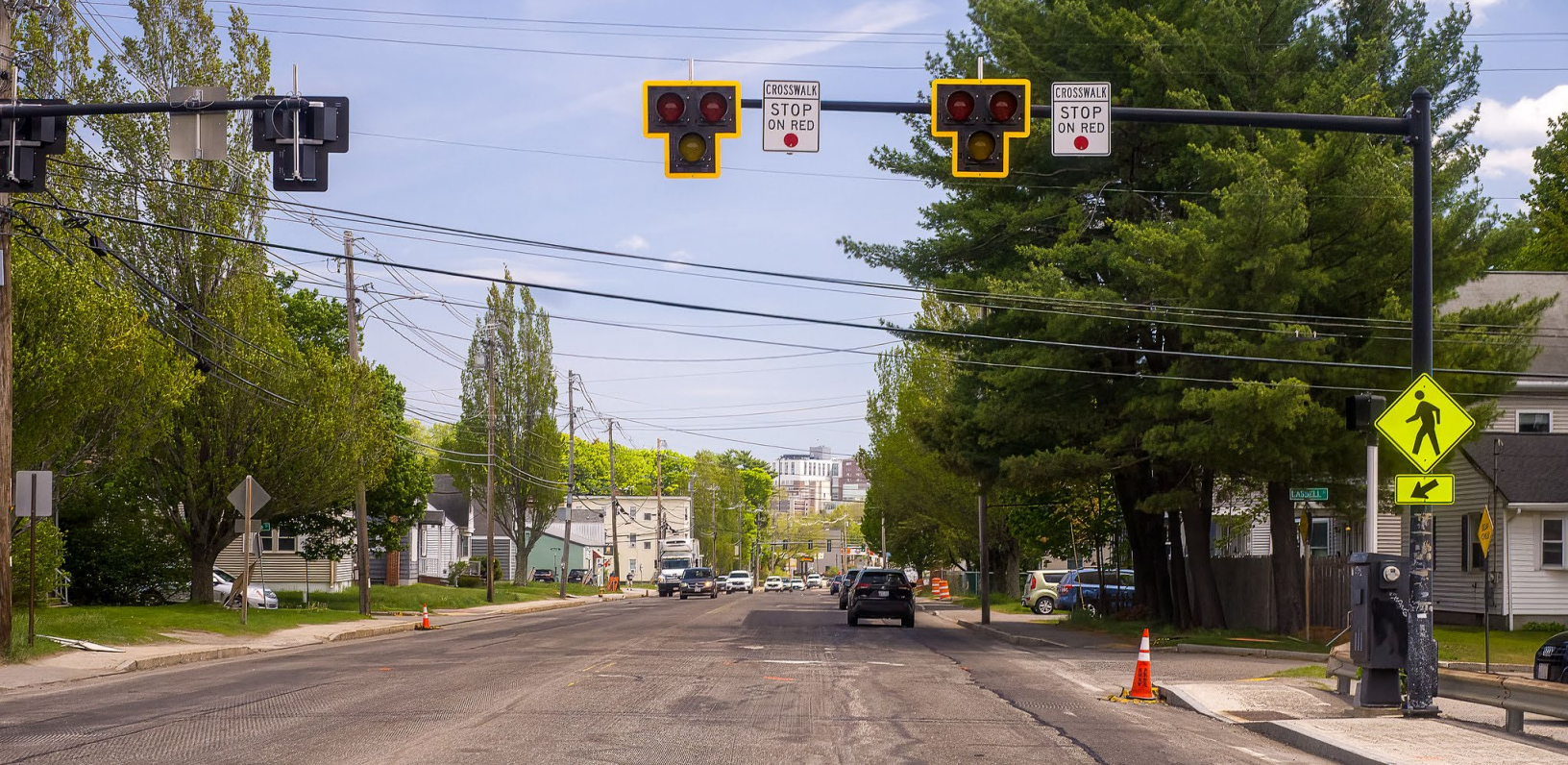
A pedestrian hybrid beacon on Congress Street in Portland, ME. Pedestrians can activate this signal to stop traffic and safely cross. Source: GPCOG
