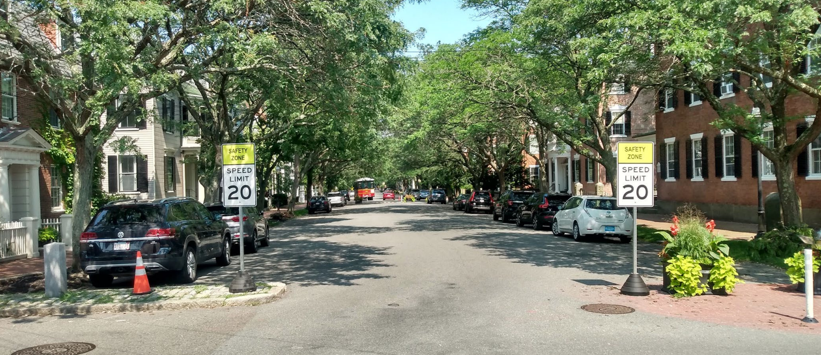
Traffic calming treatments in Salem, MA. Curb extensions, planters, speed limit signs, plastic bollards, and tree canopy provide a sense of enclosure for drivers, limiting speeds upon entry to the street. Source: Neighborways Design
