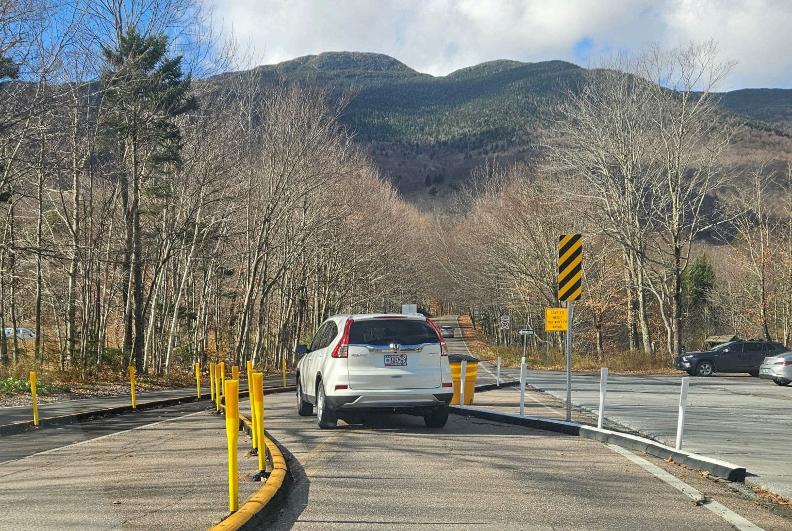
Chicanes like these in Vermont improve safety and provide traffic calming by narrowing the roadway. Currently the Town does not install 'flex posts' due to maintenance concerns. Source: Howard Stein Hudson
