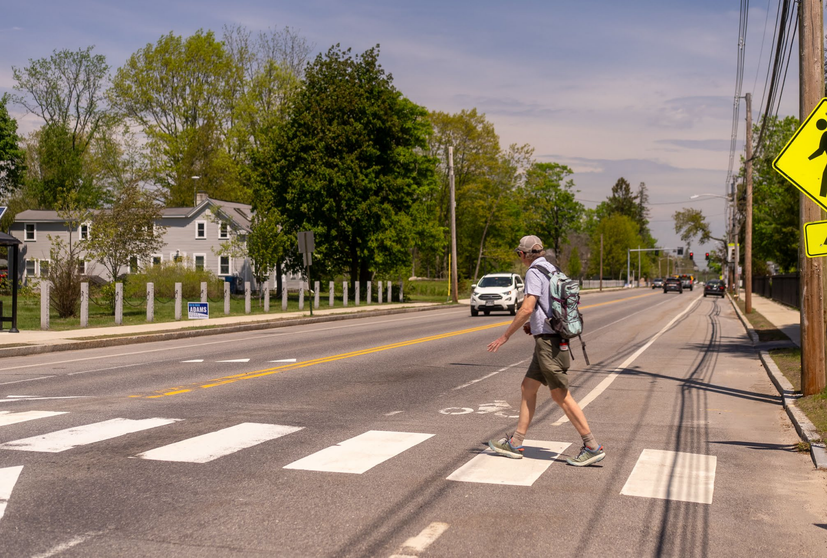
Marked crosswalk in Portland, ME. This treatment helps alert drivers of people crossing by bike or foot to encourage safe yielding. Source: GPCOG
