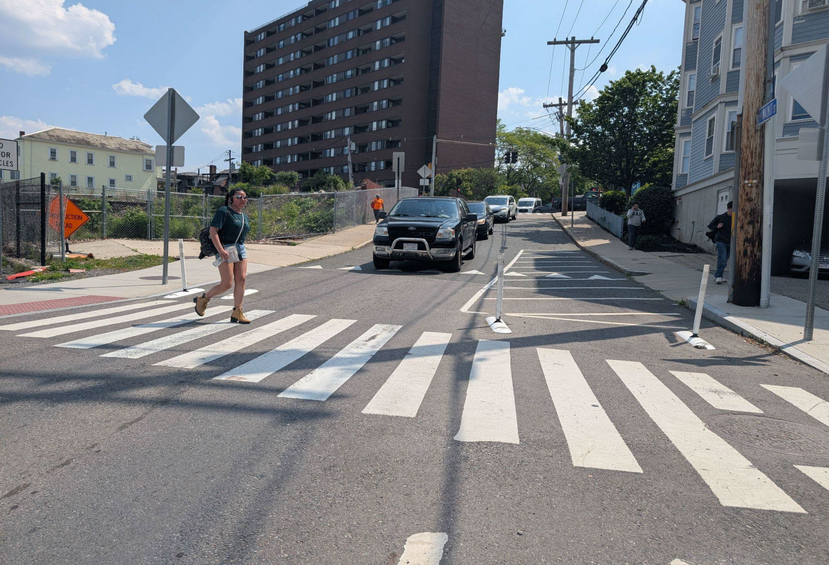
Daylighting, as seen here in Somerville, MA, helps improve sightlines for crossing pedestrians. Currently the Town does not install 'flex posts' due to maintenance concerns. Source: Neighborways Design
