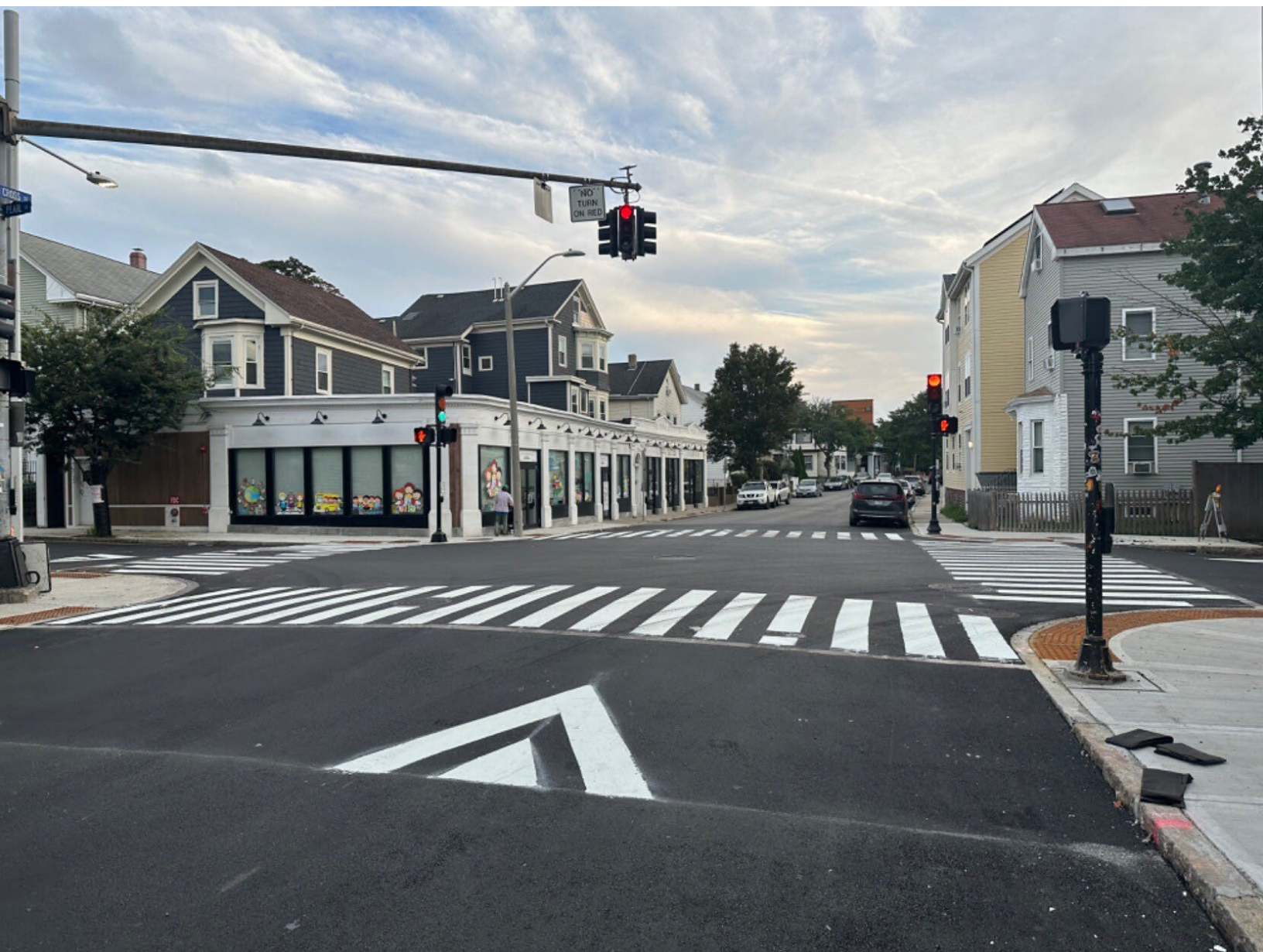
Raised intersection in Somerville, MA. This type of treatment is effective at intersections with high volumes of active transportation uses from each direction. Photo: Neighborways Design
