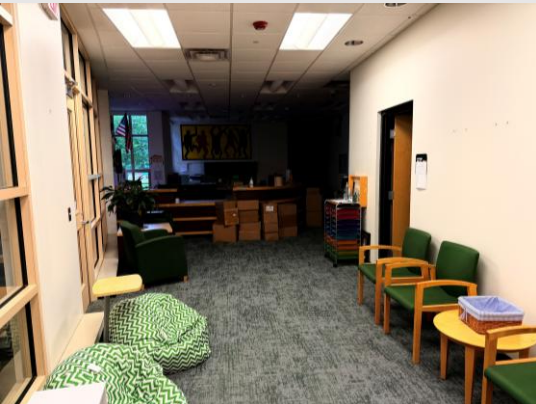
Greenfield – Main Office Flooring
