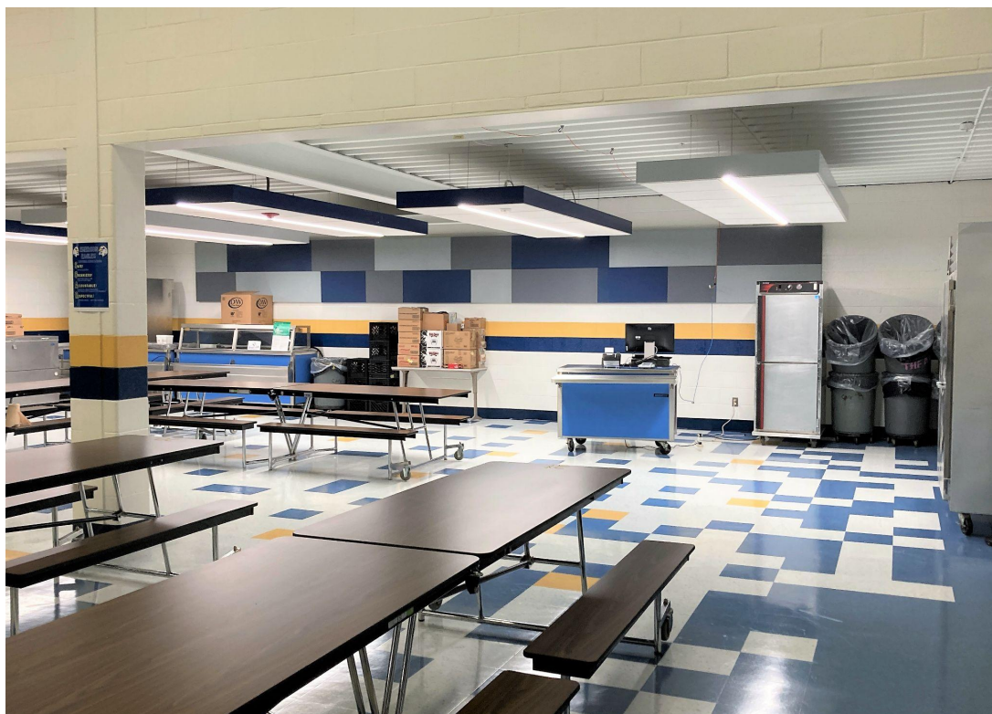
Cafeteria expansion and flooring replaced
