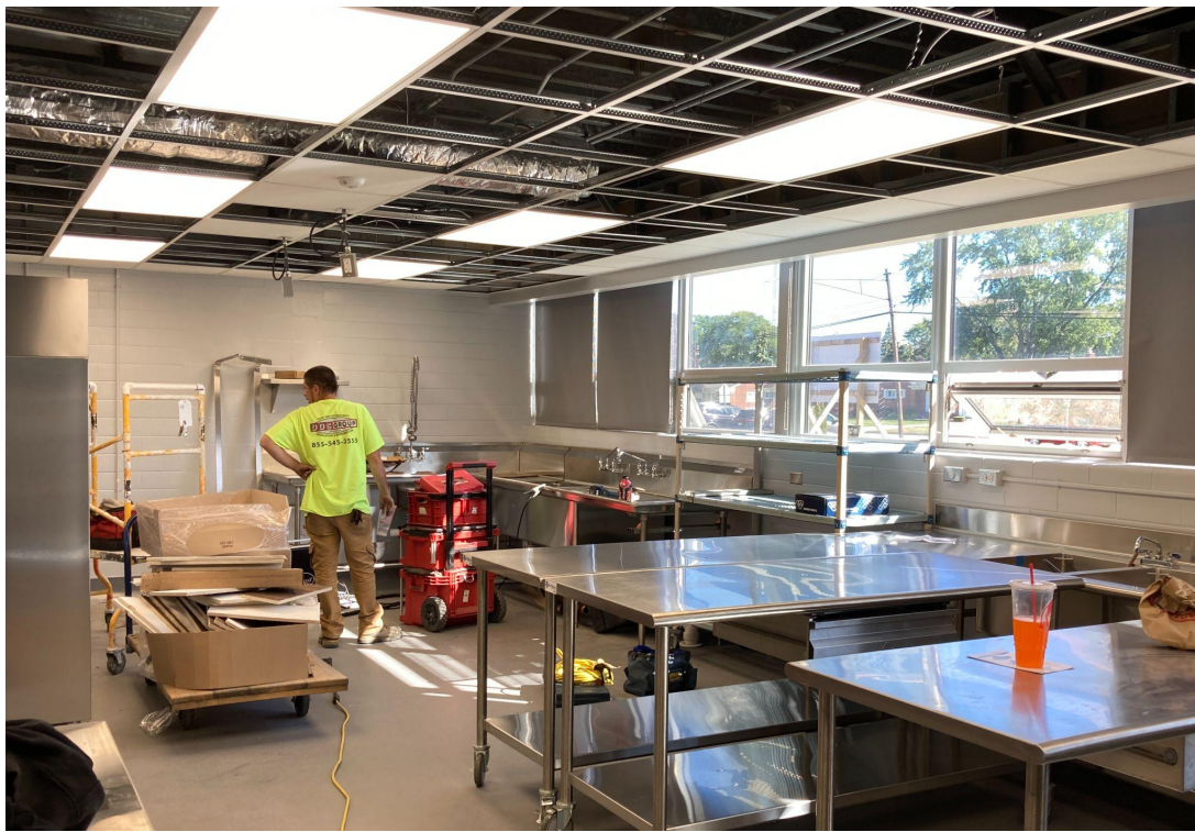
Kitchen renovation and new equipment
