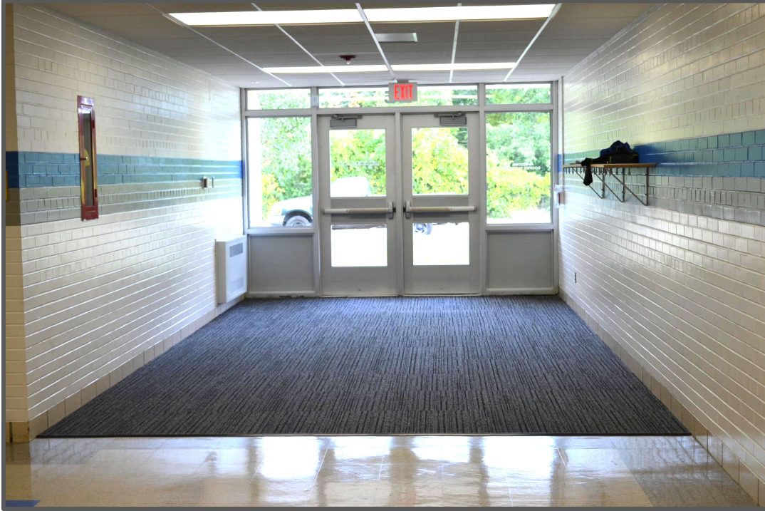
New walk-off carpet areas at doors; tiles around fountains at Cooper.
