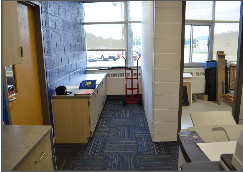
Paint, new casework in Main Office at Cooper. Clinic area is currently being remodeled.
