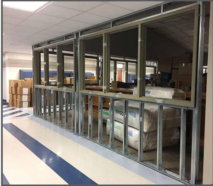
Enclosure of the learning lab at Randolph
