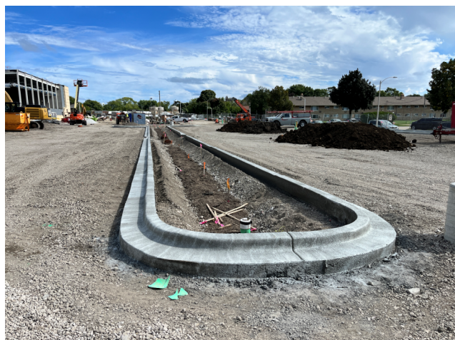
Curb Installed – Site West Parking Lot
