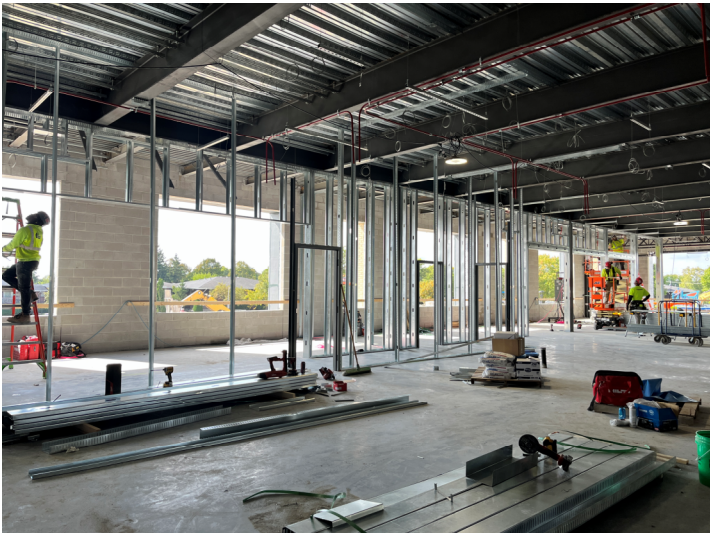
Light Gauge Framing – Area C1 1 st Level Offices
