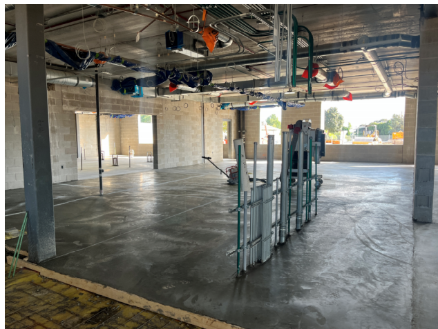
Concrete Poured – Area C1 Vocational Room
