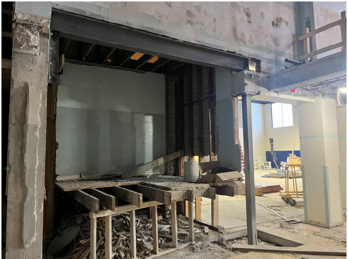
New Structural Steel Elements Installed – Area A1 1 st Level Near Stage
