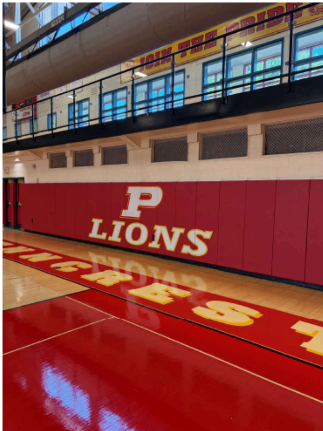
PENNCREST GYM WALL PADS
