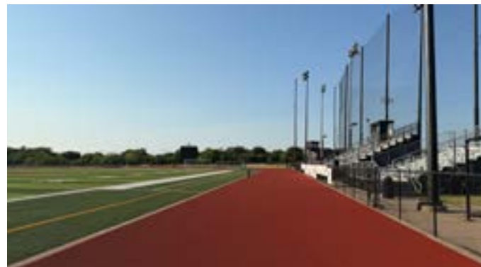
Cardinal Track Resurfacing
