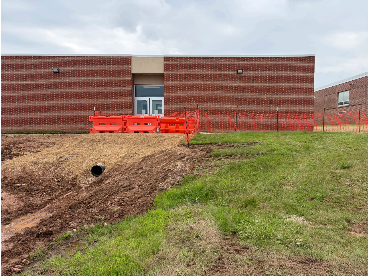
Temporary Egress at Kindergarten Wing
