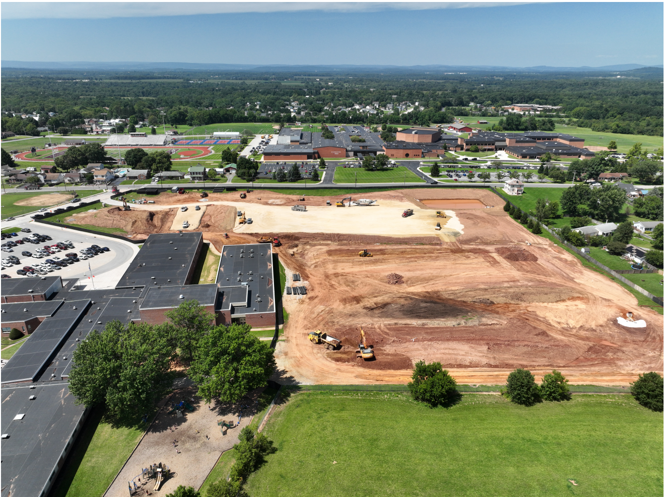
Site Grading in Progress (1)
