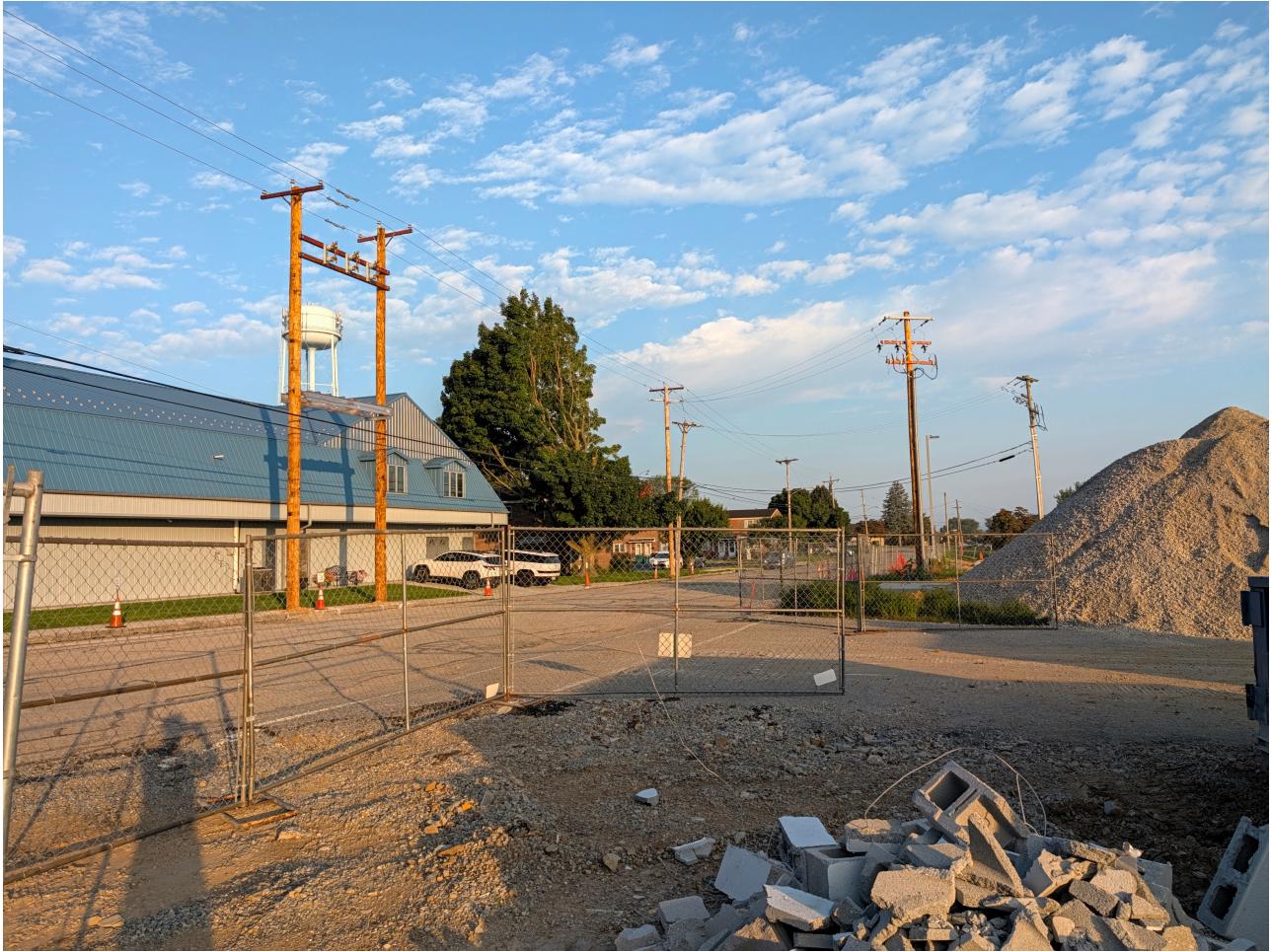
New Electric Service Progress
