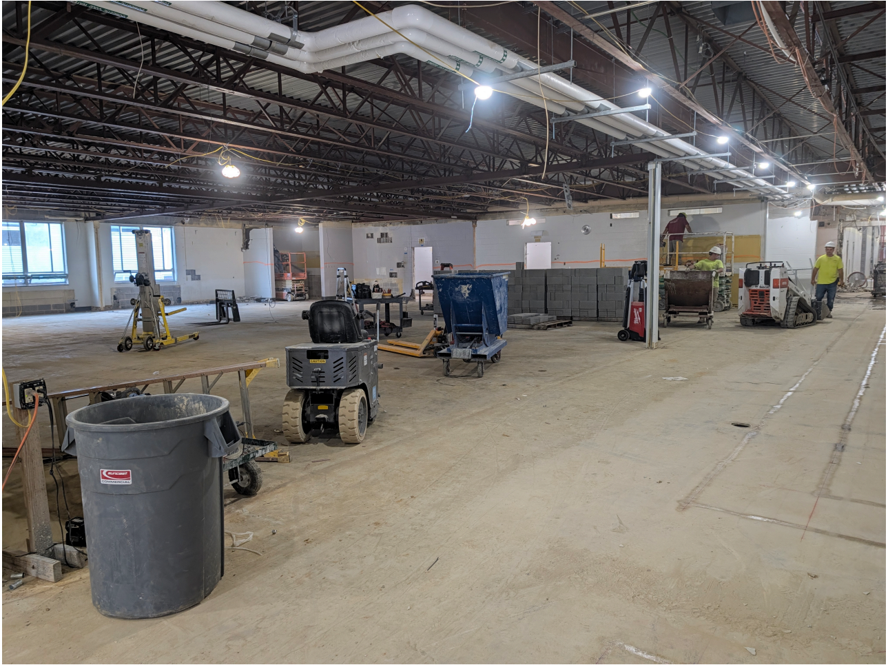
Area C Demo Progress 2
