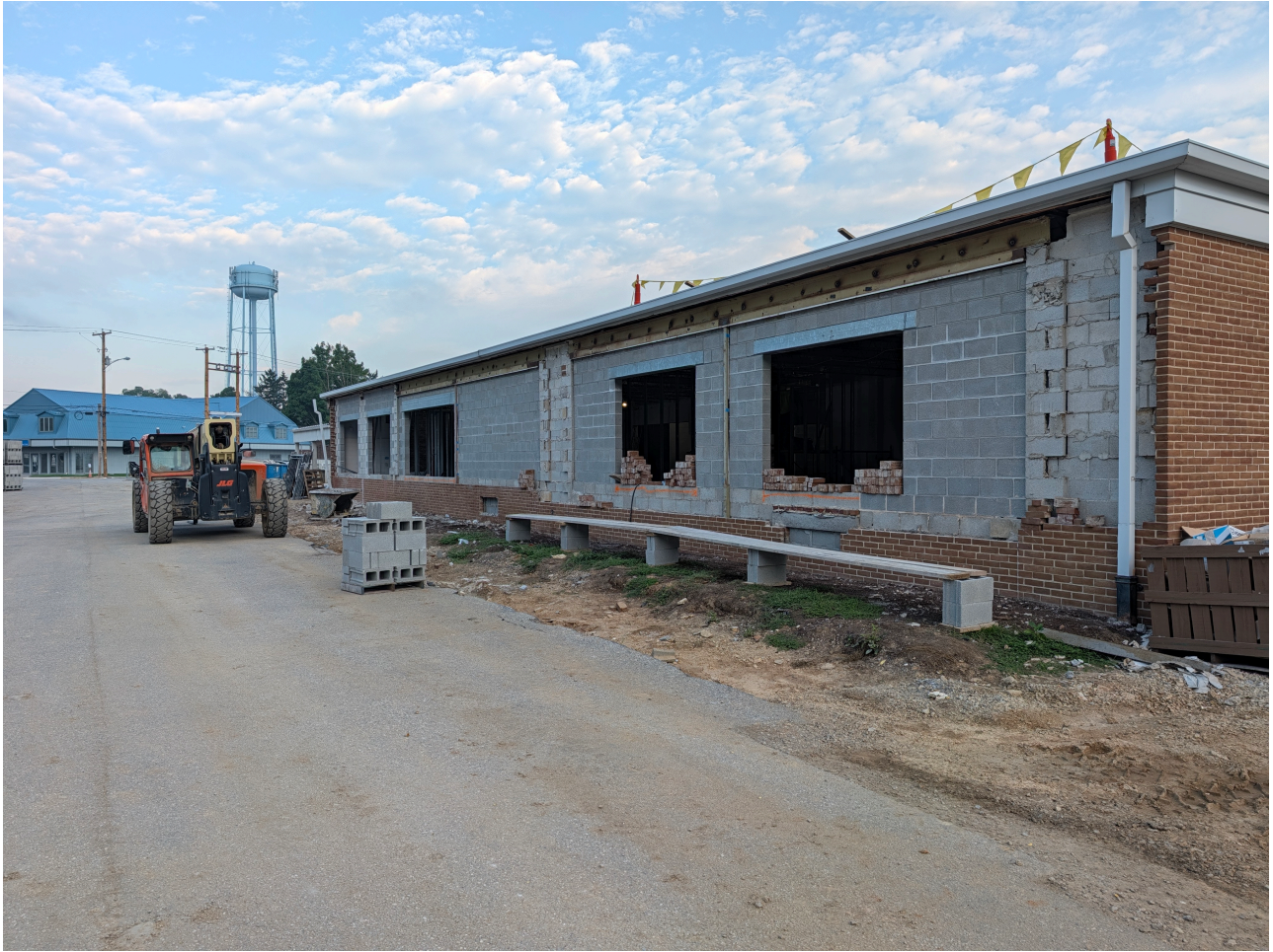
New Window Openings Area A Admin
