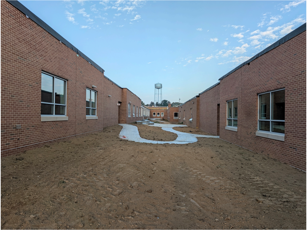
Courtyard Concrete Seating and Sidewalks Complete
