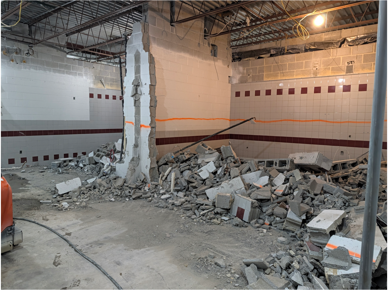
Area C Demo Progress
