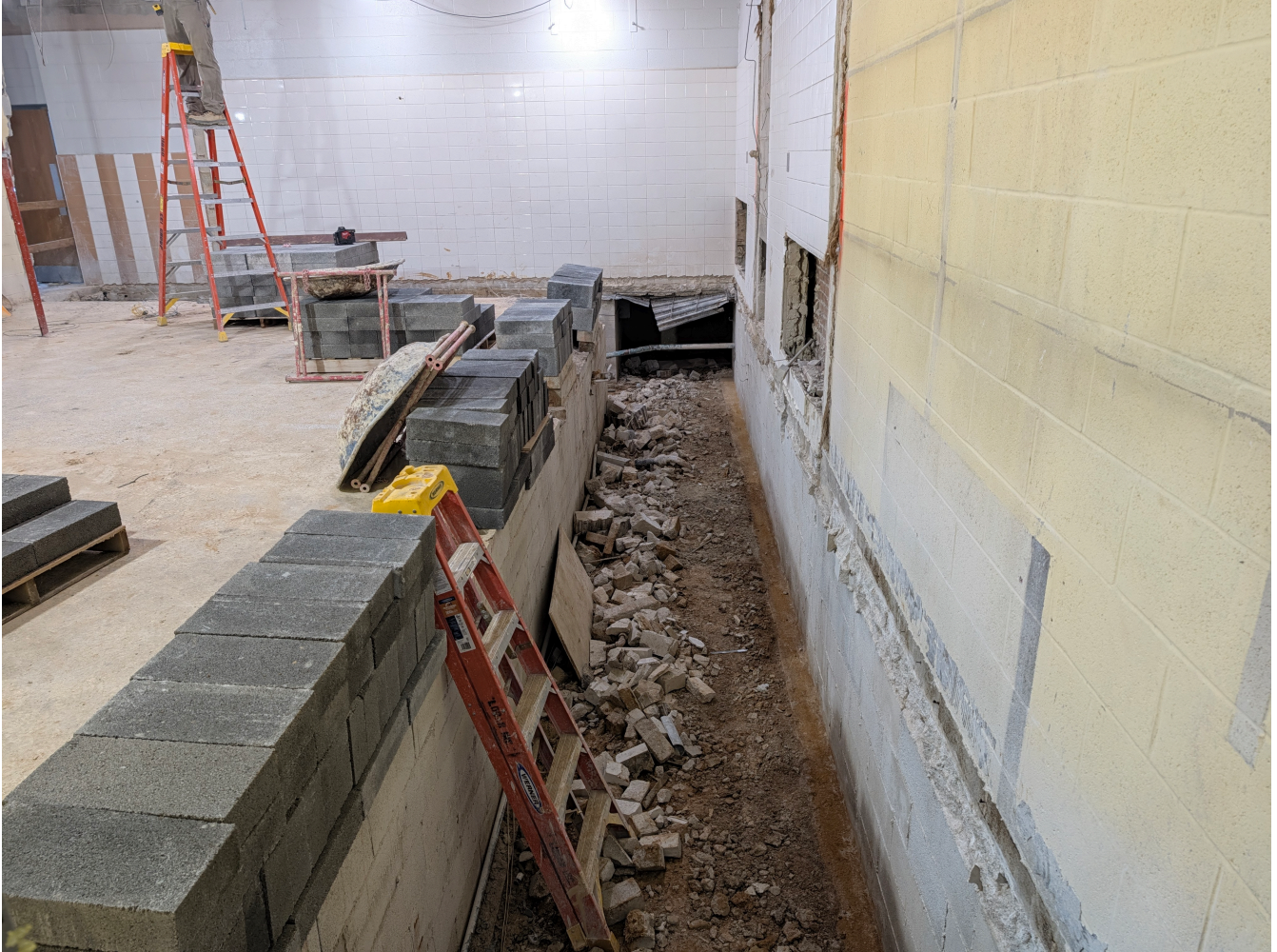
Utility Tunnel Demo Progress
