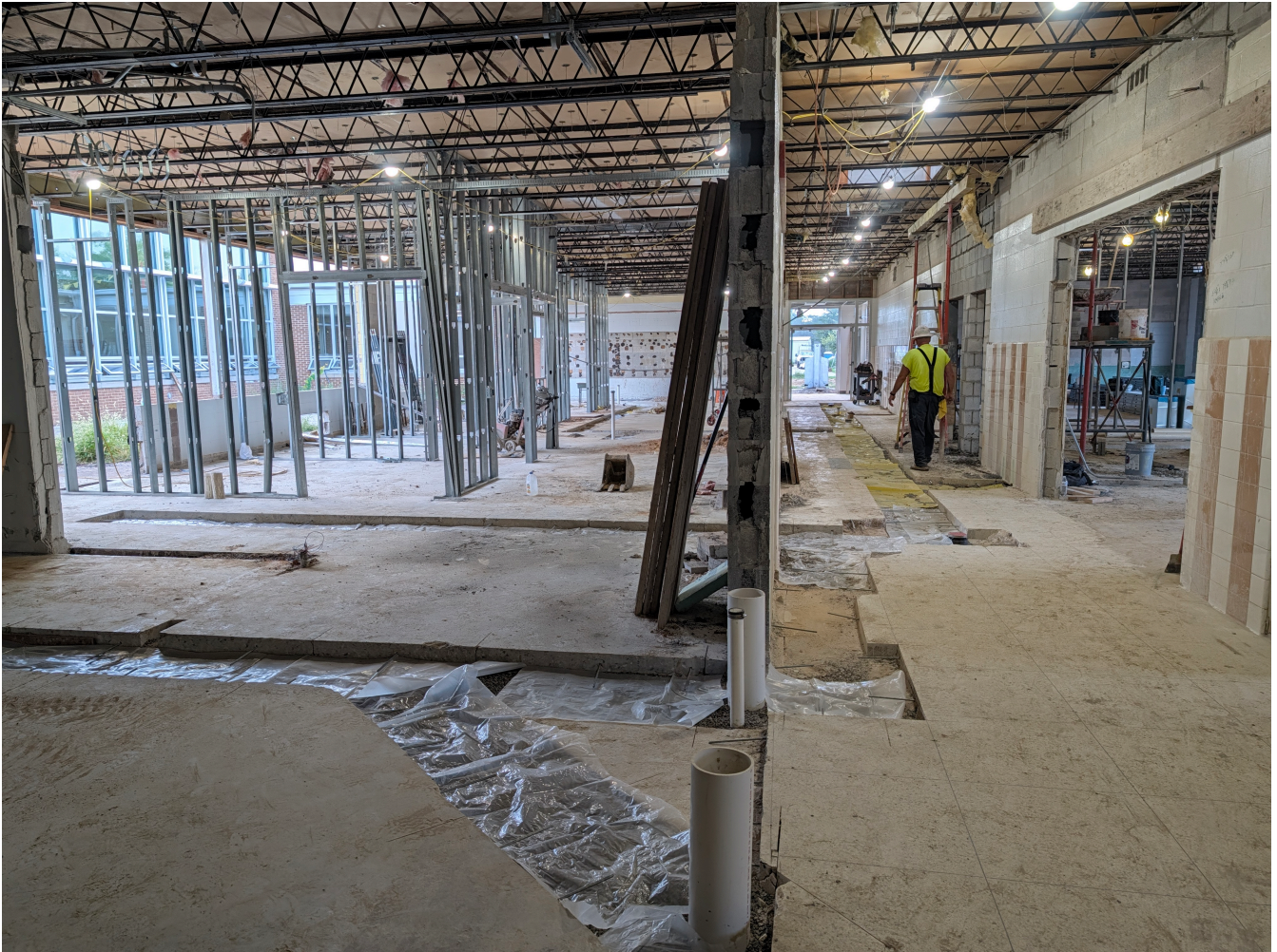
Area A Admin Progress
