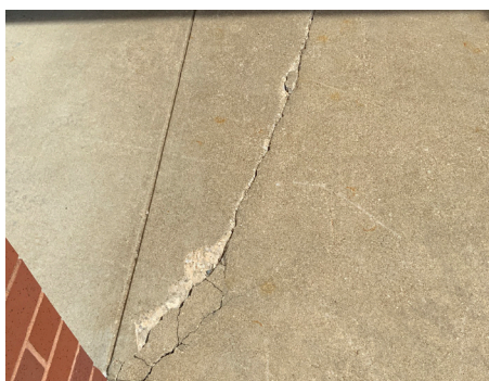
Building Site - Sidewalk
