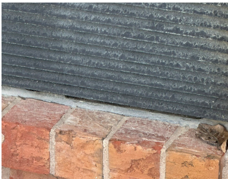
Building Structure / Exterior - Exterior Window
