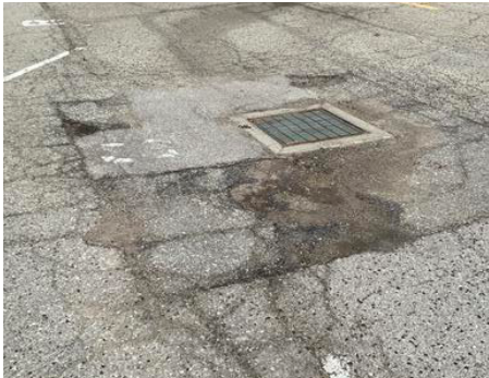
Building Site - Parking Lot
