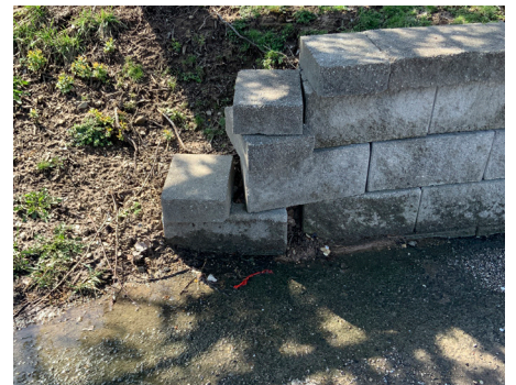
Building Site - Retaining Wall
