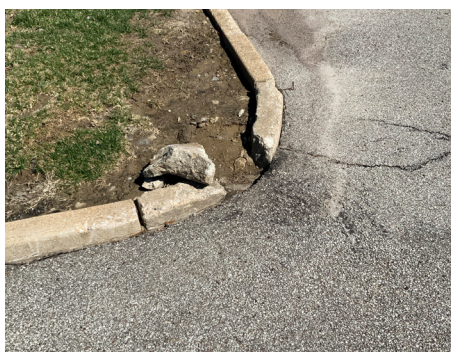
Building Site - Curbs
