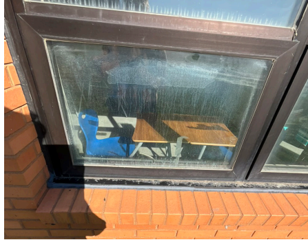
Building Structure / Exterior - Window
