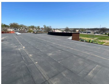
Building Structure / Exterior - Roof
