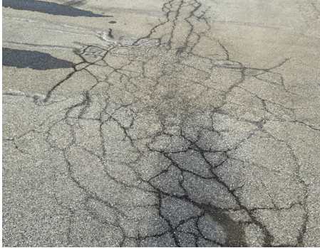
Building Site - Drive Surface
