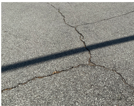
Building Site - Parking Lot
