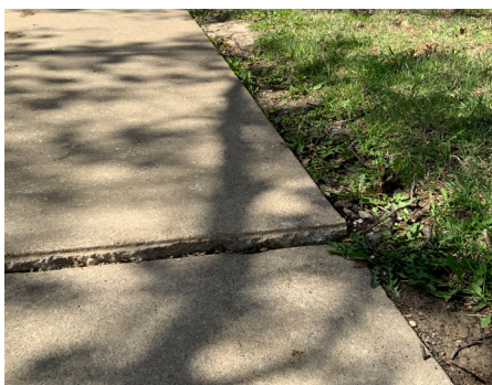
Building Site - Sidewalk
