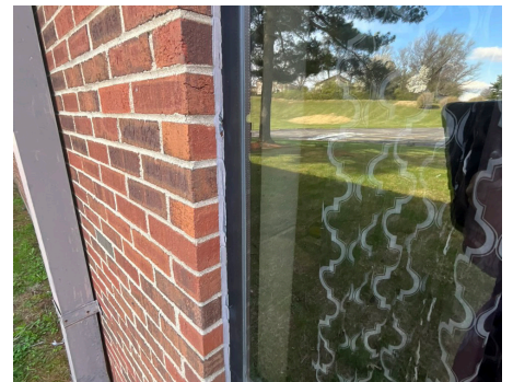
Building Structure / Exterior - Exterior Window
