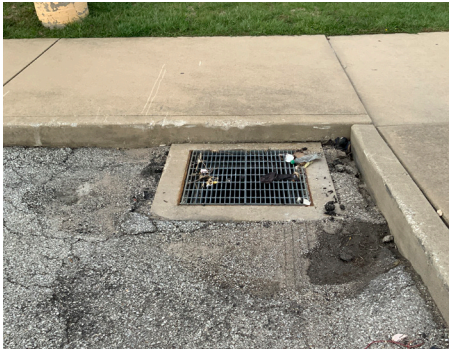
Building Site - Inlets
