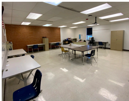
Building Systems - Interior Lighting (Classrooms)
