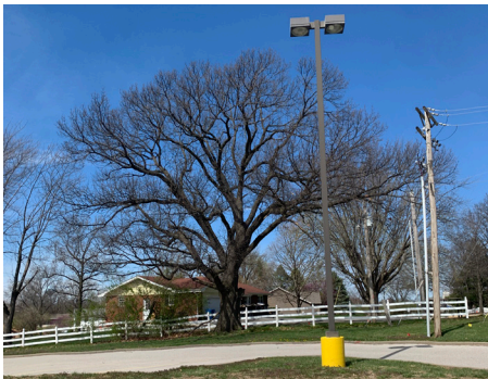
Building Site - Site Lighting
