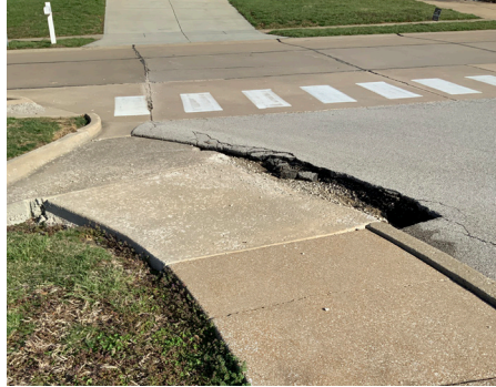
Building Site - Drive Surface
