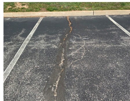
Building Site - Parking Lot
