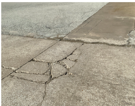
Building Site - Parking Lot
