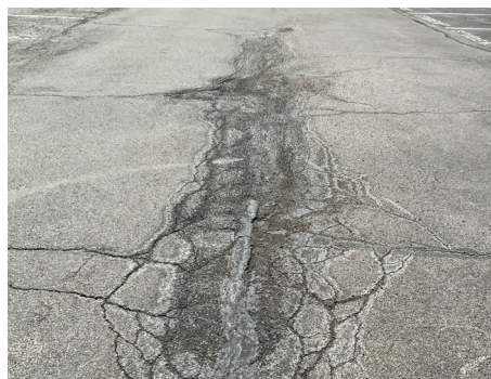
Building Site - Drive Surface
