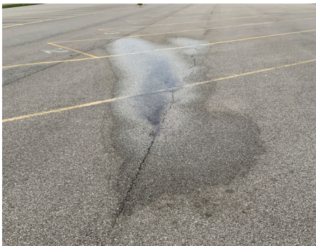
Building Site - Parking Lot
