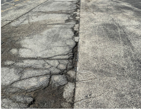
Building Site - Drive Surface
