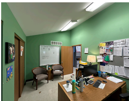
Building Systems - Interior Lighting (Public Areas)
