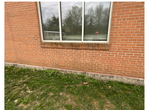
Building Structure / Exterior - Exterior Facade
