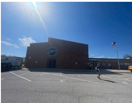
Building Site - Site Lighting
