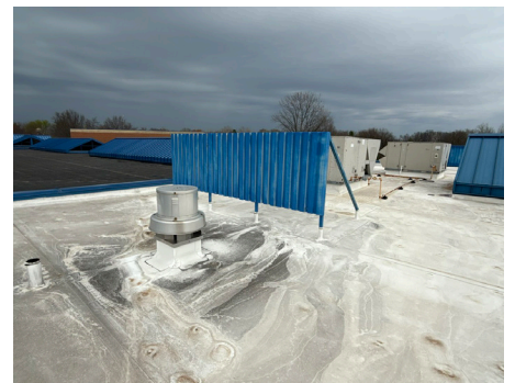
Building Structure / Exterior - Roof Screen
