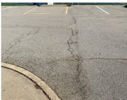
Building Site - Parking Lot
