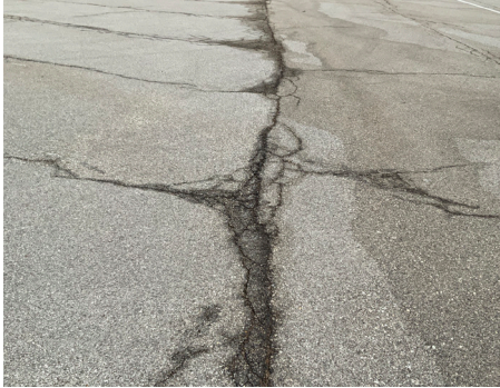
Building Site - Drive Surface
