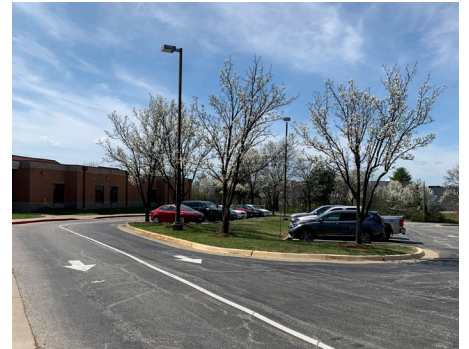
Building Site - Site Lighting
