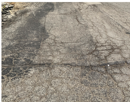
Building Site - Drive Surface
