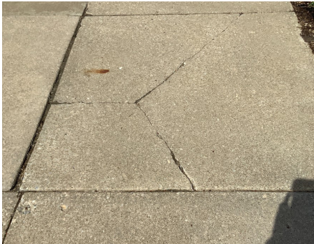
Building Site - Sidewalk
