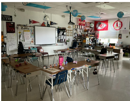
Building Systems - Interior Lighting (Classrooms)
