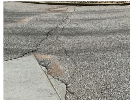
Building Site - Parking Lot
