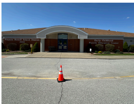
Building Site - Parking Lot
