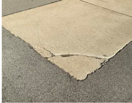
Building Site - Sidewalk
