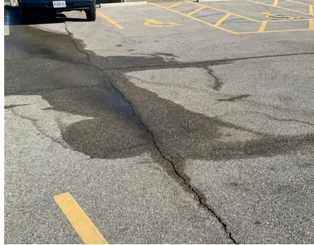
Building Site - Parking Lot
