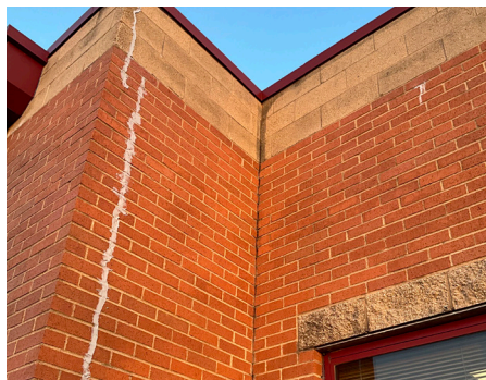
Building Structure / Exterior - Structural System
