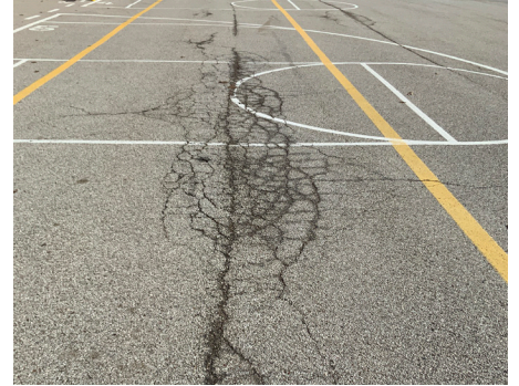
Building Site - Parking Lot
