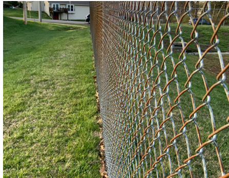
Building Site - Fencing
