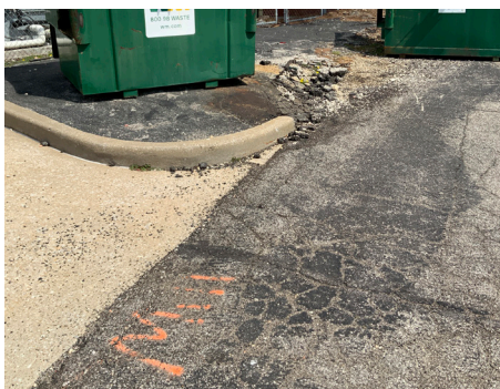
Building Site - Loading Area
