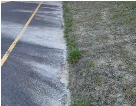
Building Site - Drainage System
