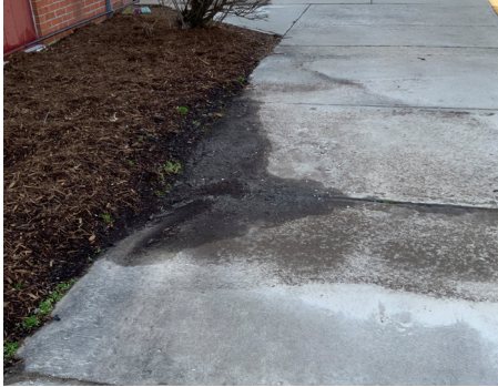
Building Site - Drainage System
