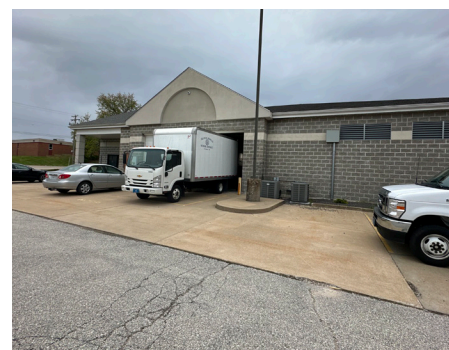
Building Site - Site Lighting
