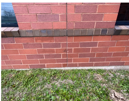
Building Structure / Exterior - Exterior Facade
