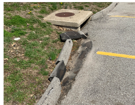
Building Site -Curbs
