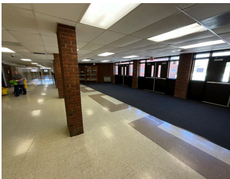
Building Systems - Interior Lighting (Public Areas)
