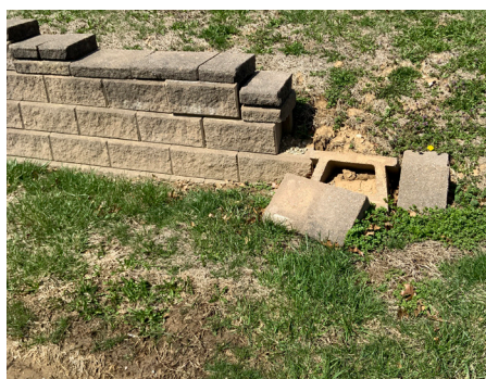
Building Site - Retaining Wall
