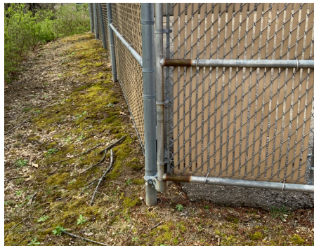
Building Site - Fencing
