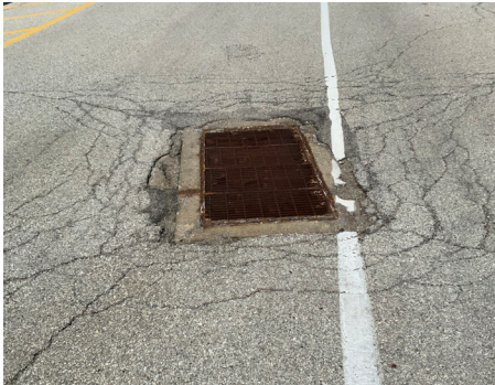
Building Site - Inlets
