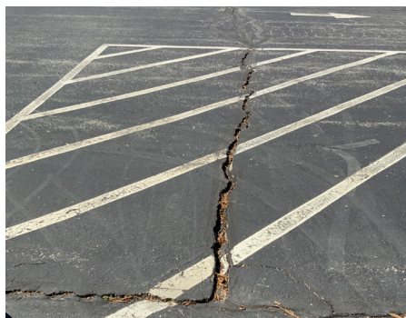
Building Site - Drive Surface
