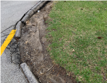
Building Site - Curbs
