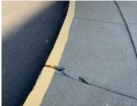
Building Site - Sidewalk
