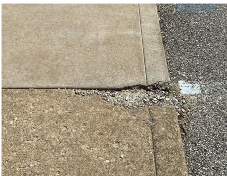
Building Site - Curbs
