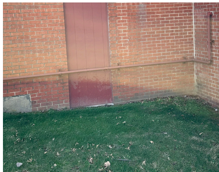
Building Site - Turf Grass
