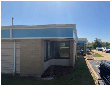
Building Structure / Exterior - Exterior Facade
