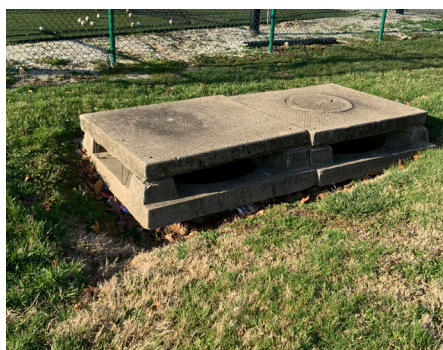
Building Site - Inlets
