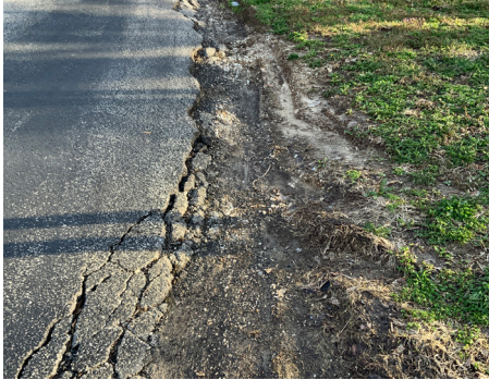
Building Site - Drive Surface
