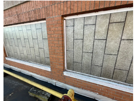
Building Structure / Exterior - Exterior Window
