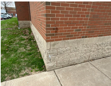
Building Structure / Exterior - Structural System
