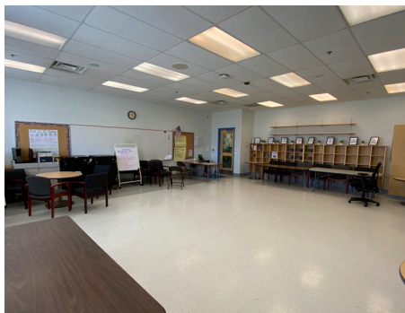
Building Systems - Interior Lighting (Classrooms)
