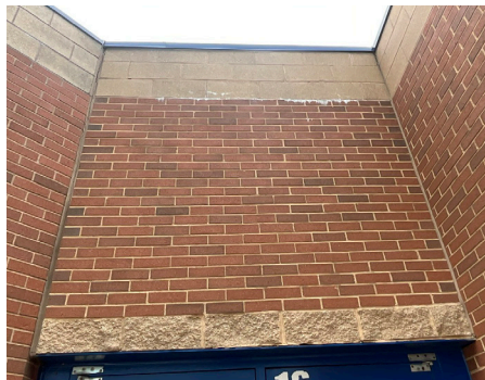
Building Structure / Exterior - Exterior Facade
