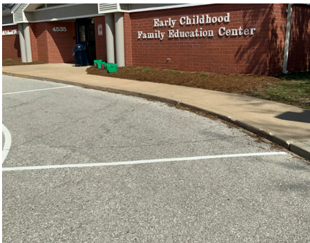
Building Site - Curbs
