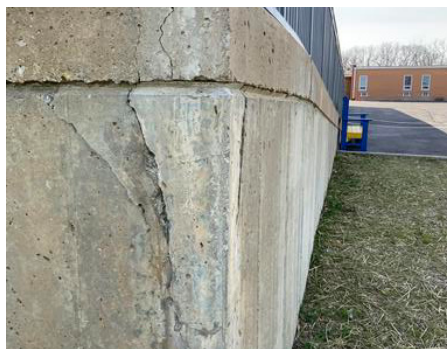
Building Site - Retaining Wall
