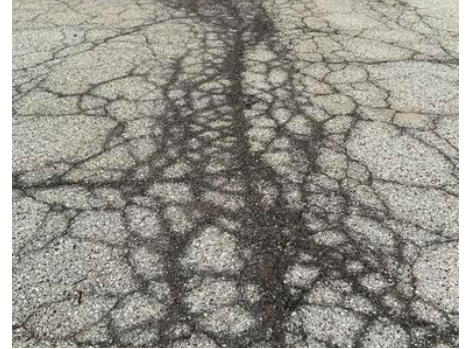
Building Site - Parking Lot
