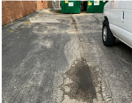
Building Site - Loading Area
