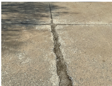
Building Site - Sidewalk
