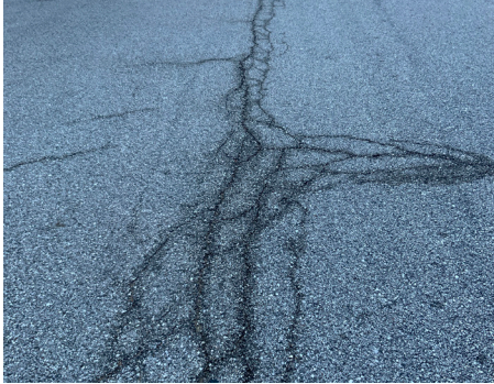
Building Site - Drive Surface
