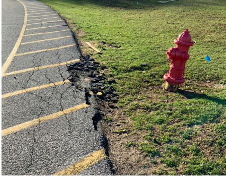
Building Site - Drive Surface
