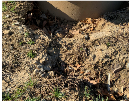
Building Site - Inlets
