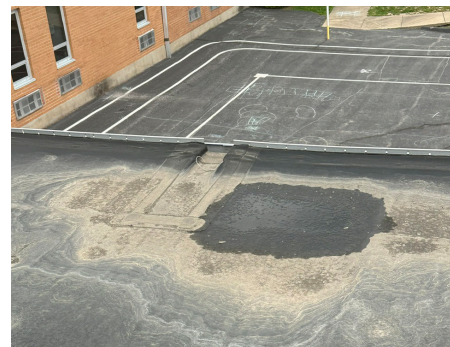
Building Structure / Exterior - Roof
