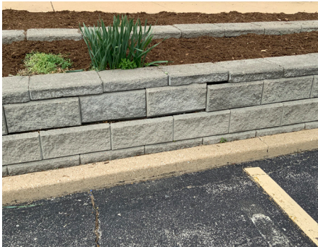
Building Site - Retaining Wall
