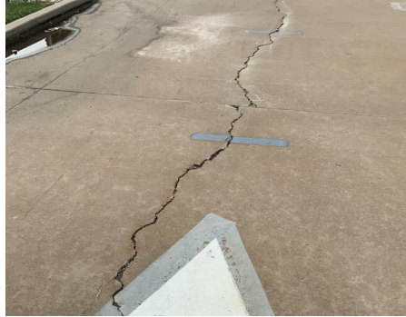
Building Site - Drive Surface
