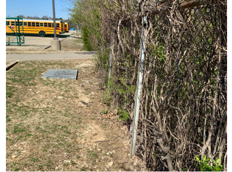
Building Site - Fencing
