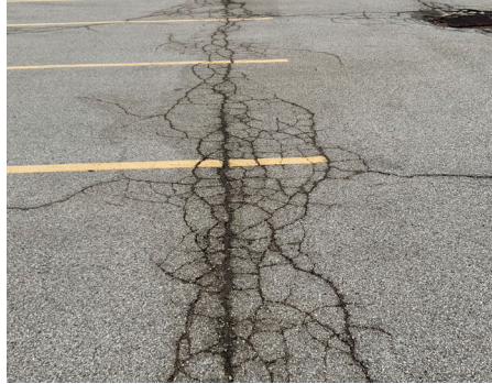
Building Site - Parking Lot
