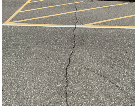
Building Site - Drive Surface
