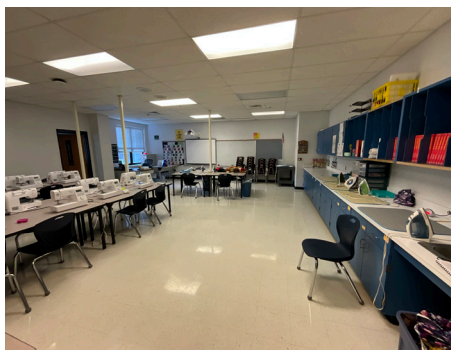
Building Systems - Interior Lighting (Classrooms)
