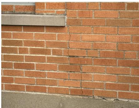
Building Structure / Exterior - Exterior Facade
