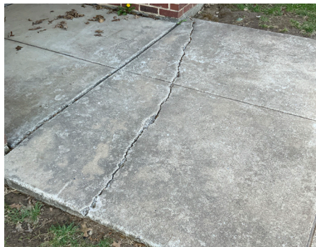
Building Site - Sidewalks
