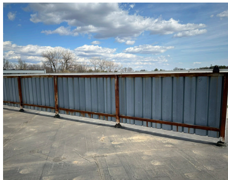
Building Structure / Exterior - Roof Screen
