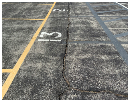
Building Site - Parking Lot
