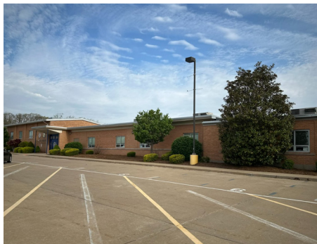
Building Site - Site Lighting
