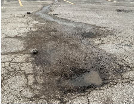
Building Site - Parking Lot
