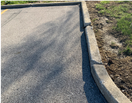
Building Site - Curbs
