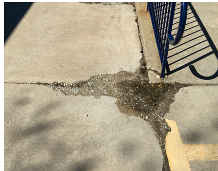
Building Site - Sidewalk
