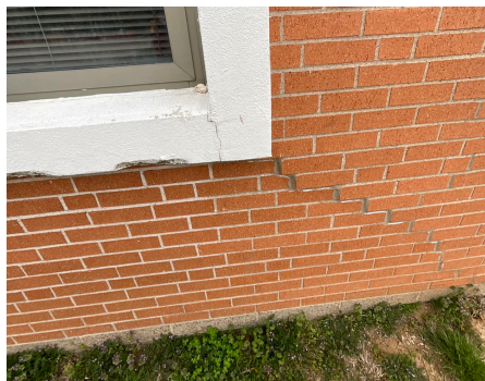
Building Structure / Exterior - Structural System
