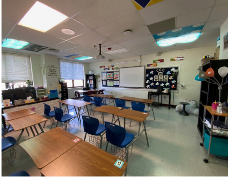
Building Systems - Interior Lighting (Classrooms)
