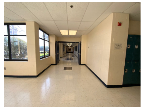
Building Systems - Interior Lighting (Public Areas)
