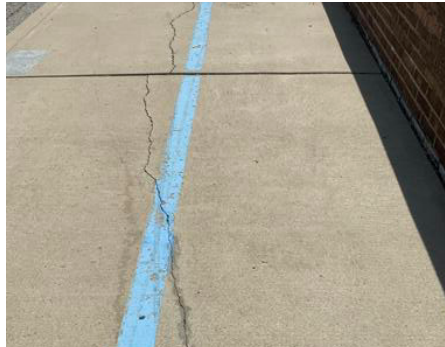
Building Site - Sidewalk
