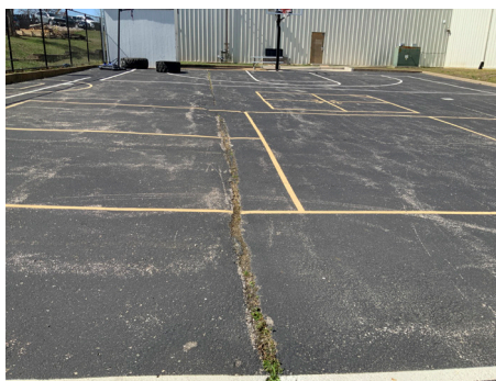
Building Site - Hardscape Play
