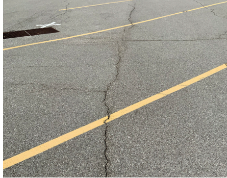
Building Site - Parking Lot
