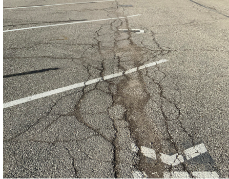
Building Site - Parking Lot
