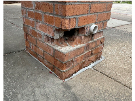
Building Structure / Exterior - Structural System
