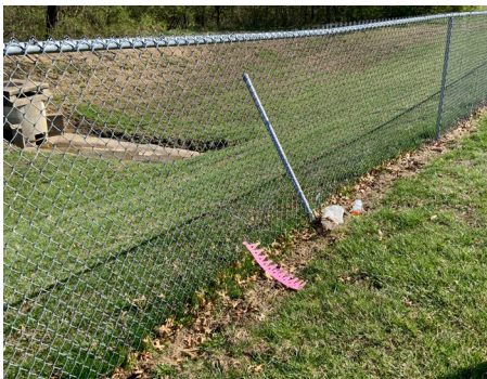
Building Site - Fencing
