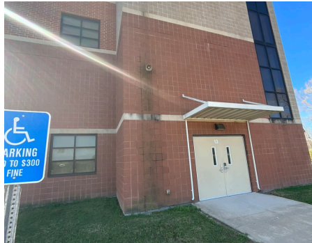
Building Structure / Exterior - Exterior Facade
