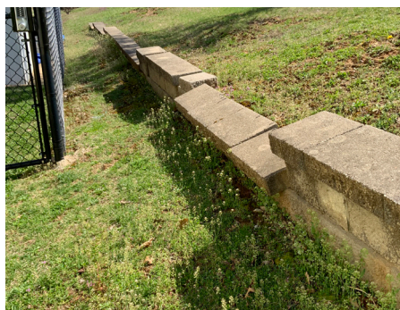
Building Site - Retaining Wall
