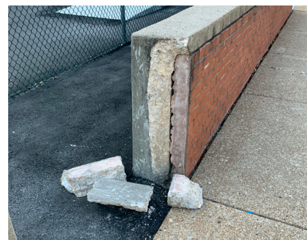
Building Site - Retaining Wall
