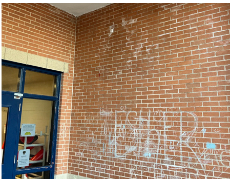
Building Structure / Exterior - Exterior Facade
