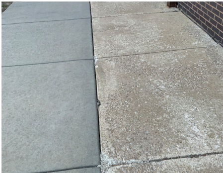
Building Site - Sidewalk
