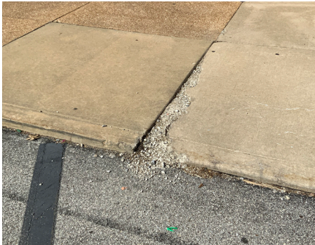
Building Site - Sidewalk
