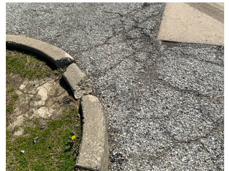
Building Site - Curbs
