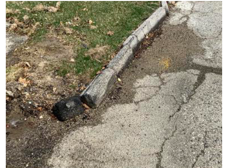
Building Site - Curbs
