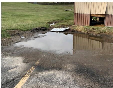
Building Site - Drainage System
