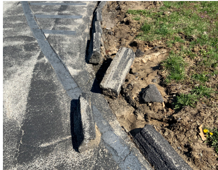
Building Site - Curbs
