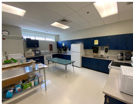
Building Systems - Interior Lighting (Classrooms)
