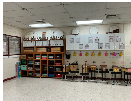
Building Systems - Interior Lighting (Classrooms)
