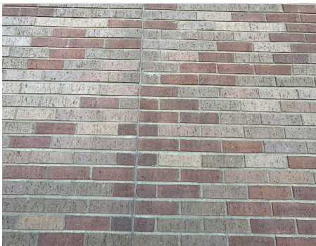
Building Structure / Exterior - Exterior Facade
