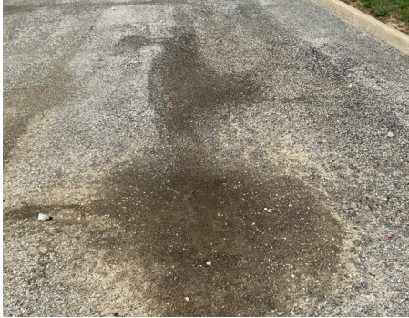
Building Site - Drive Surface
