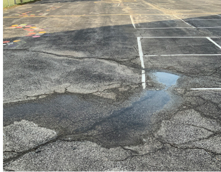
Building Site - Parking Lot
