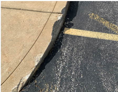
Building Site - Curbs
