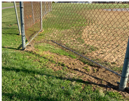
Building Site - Fencing
