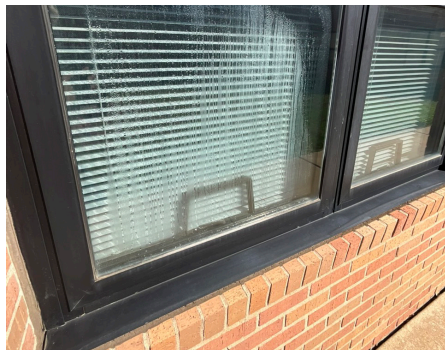
Building Structure / Exterior - Exterior Window
