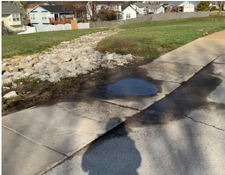
Building Site - Sidewalk
