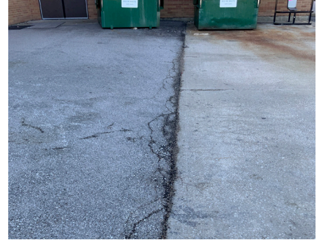
Building Site - Loading Area
