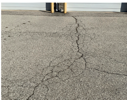
Building Site - Loading Area
