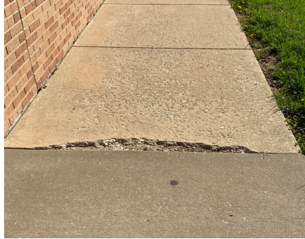
Building Site - Sidewalk
