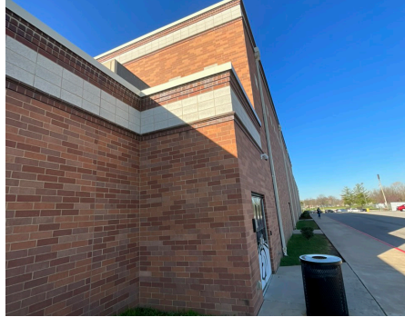
Building Structure / Exterior - Exterior Facade
