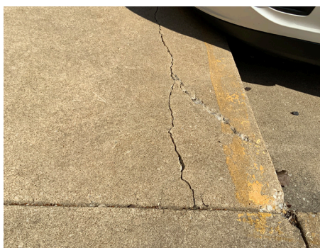
Building Site - Sidewalk
