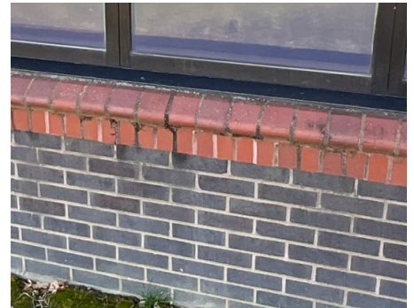
Building Structure / Exterior - Exterior Facade
