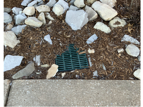
Building Site - Inlets
