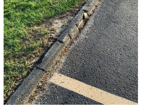
Building Site - Curbs
