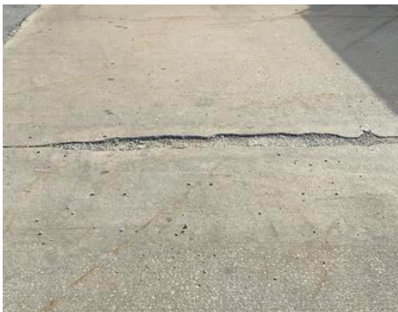
Building Site - Loading Area
