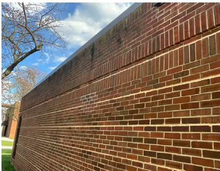
Building Structure / Exterior - Exterior Facade
