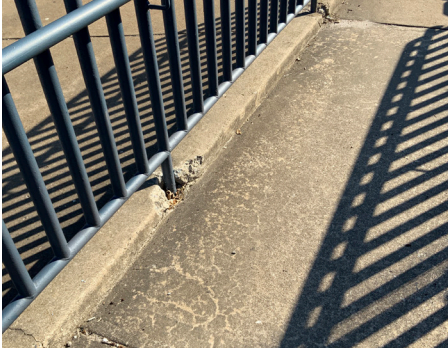
Building Site - Fencing
