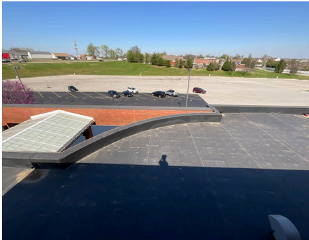
Building Structure / Exterior - Roof
