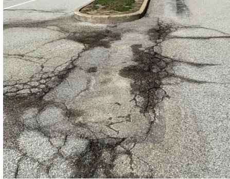
Building Site - Parking Lot
