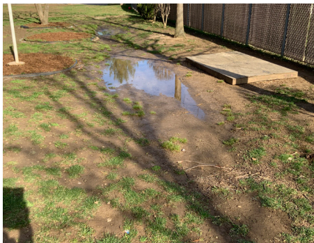
Building Site - Drainage System
