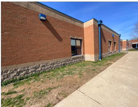
Building Site - Site Lighting
