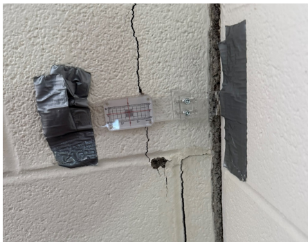
Building Structure / Exterior - Structural System
