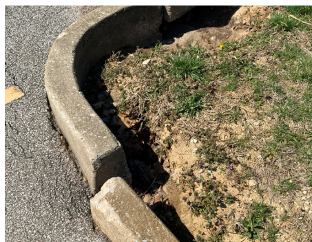
Building Site - Inlets
