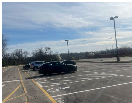
Building Site - Site Lighting
