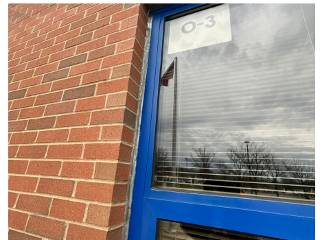
Building Structure / Exterior - Exterior Window
