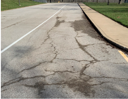
Building Site - Drive Surface
