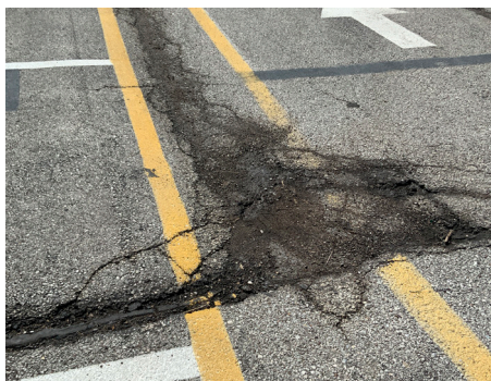
Building Site - Drive Surface
