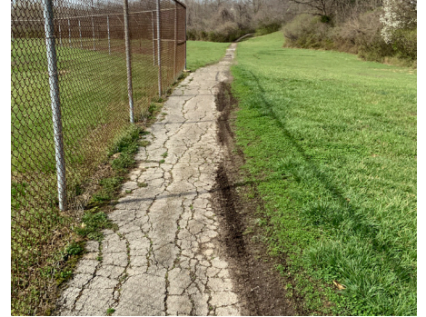
Building Site - Sidewalk
