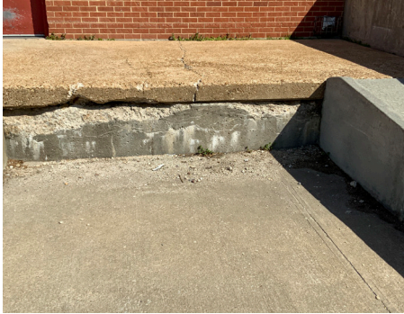
Building Site - Loading Area
