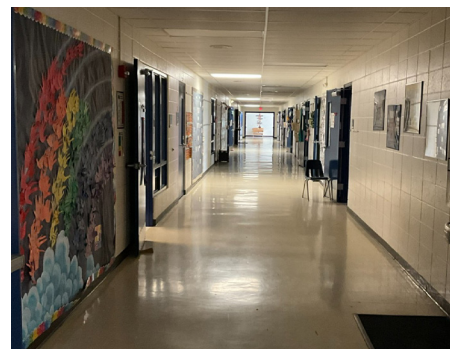
Building Systems - Interior Lighting (Public Areas)
