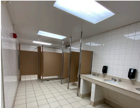
Building Systems - Mechanical System
