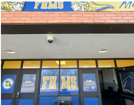
Building Site - Site Lighting
