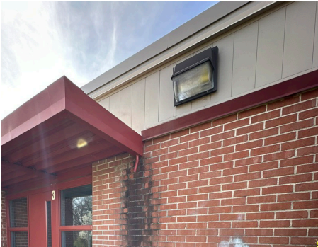
Building Sites - Site Lighting
