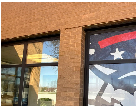
Building Structure / Exterior - Exterior Window
