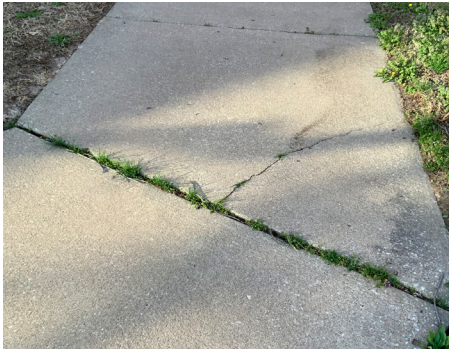
Building Site - Sidewalk
