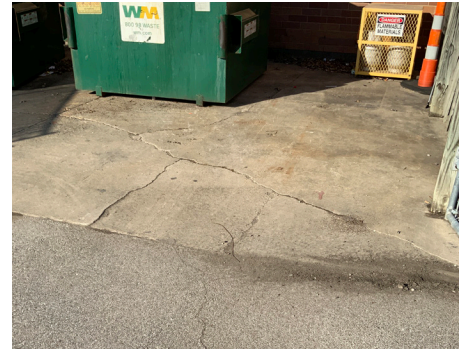
Building Site - Loading Area
