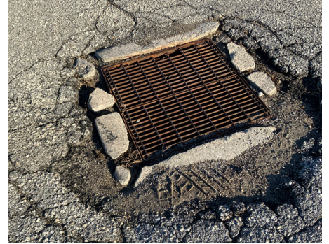
Building Site - Inlets
