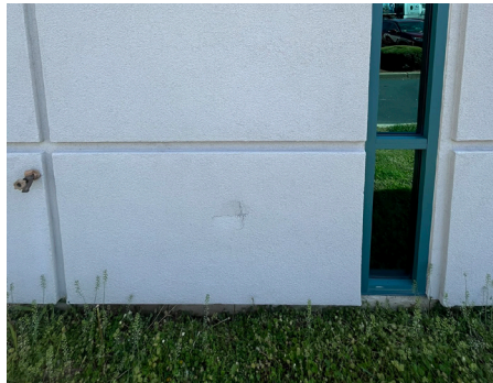
Building Structure / Exterior - Exterior Facade
