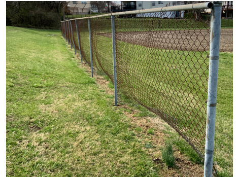
Building Site - Fencing
