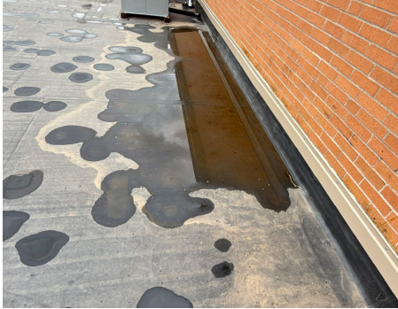
Building Structure / Exterior - Roof
