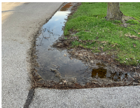
Building Site - Drainage System
