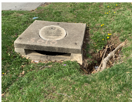
Building Site - Inlets
