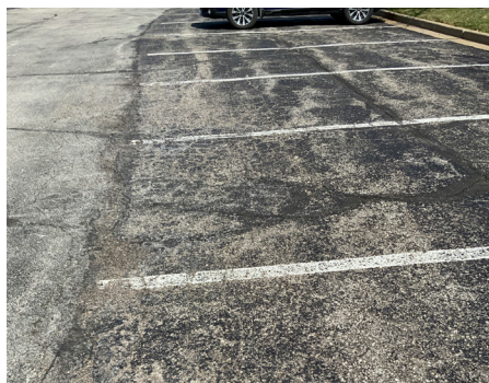
Building Site - Parking Lot
