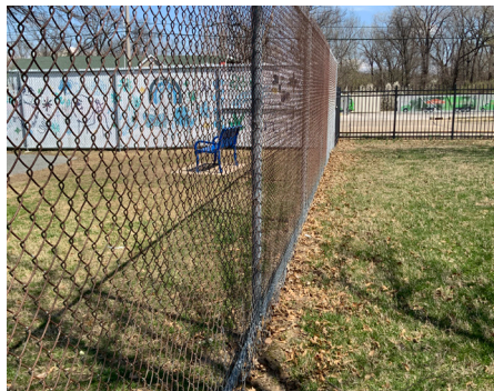
Building Site - Fencing
