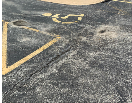
Building Site - Parking Lot
