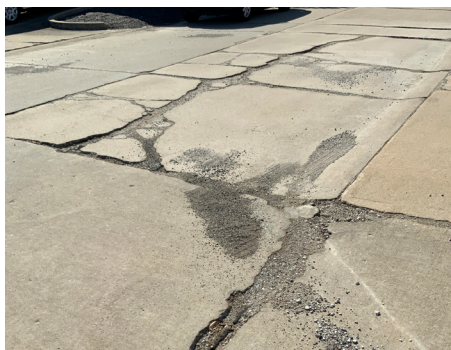
Building Site - Drive Surface
