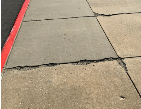
Building Site - Sidewalk
