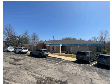
Building Site - Site Lighting
