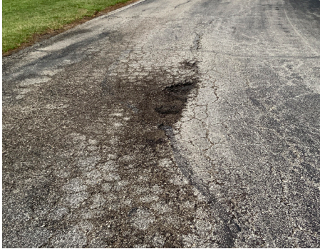
Building Site - Drive Surface
