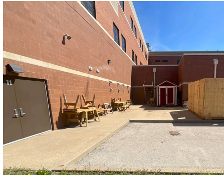
Building Site - Site Lighting
