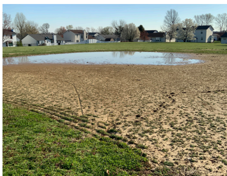
Building Site - Drainage System
