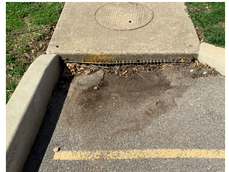
Building Site - Inlets
