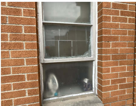
Building Structure / Exterior - Exterior Window
