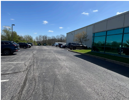
Building Site - Site Lighting
