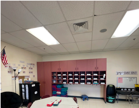
Building Systems - Interior Lighting (Classrooms)
