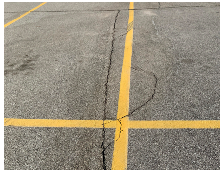
Building Site - Parking Lot
