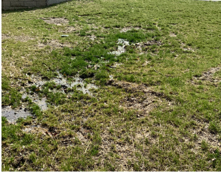
Building Site - Drainage System
