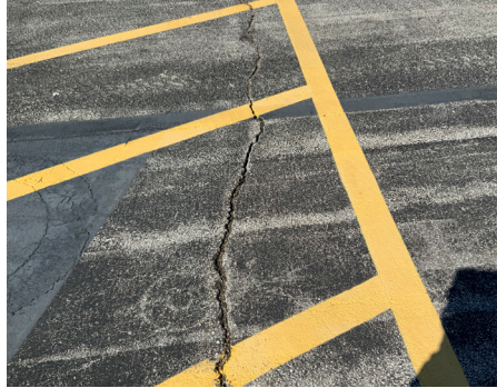
Building Site - Drive Surface
