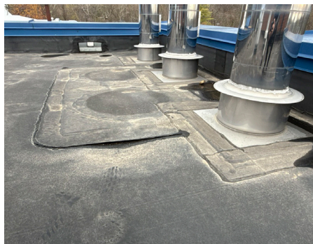
Building Structure / Exterior - Roof
