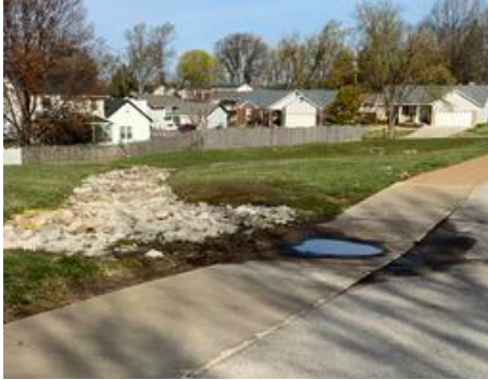
Building Site - Drainage System
