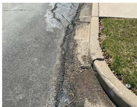
Building Site - Curbs
