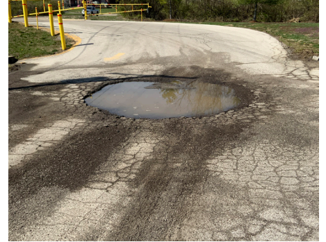
Building Site - Parking Lot
