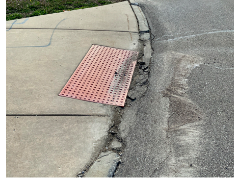
Building Site - Curbs
