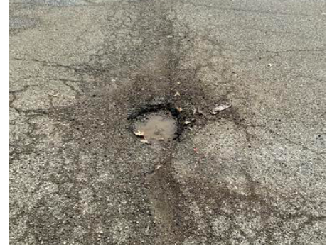
Building Site - Drive Surface
