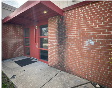
Building Structure / Exterior - Exterior Facade
