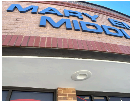
Building Site - Site Lighting
