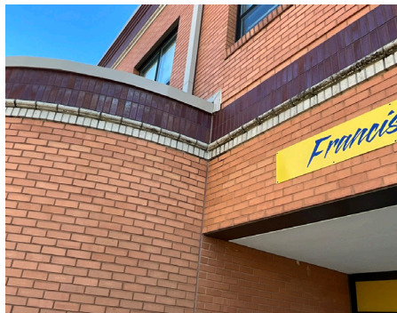
Building Structure / Exterior - Exterior Facade
