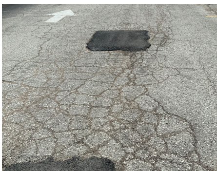
Building Site - Entrance to ROW
