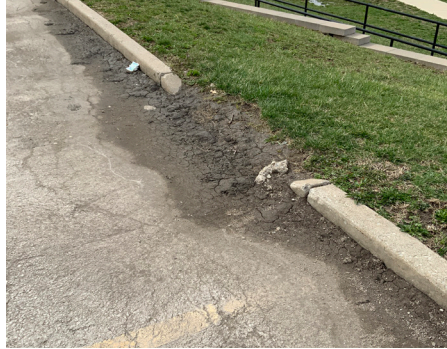
Building Site - Curbs
