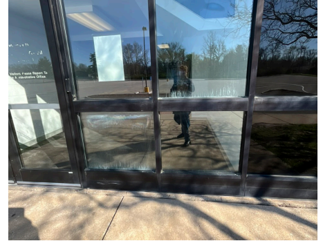
Building Structure / Exterior - Exterior Window
