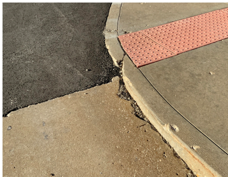
Building Site - Curbs
