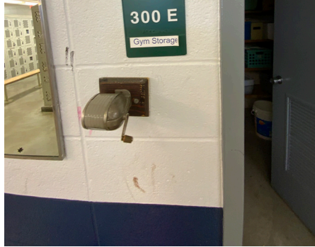
Interior Environment - Interior Wall
