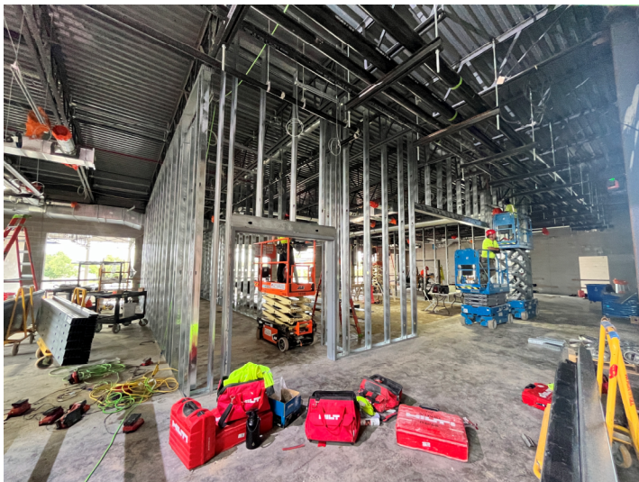
Metal Stud Framing – Area B1 1 st Level
