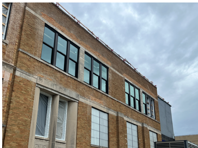
Windows Installed – Area A1 North Elevation
