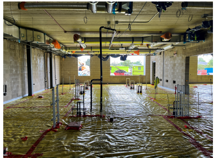
Prepped For Concrete Pour – Area C1 Ground Level Corridor & Vocational Training Rooms
