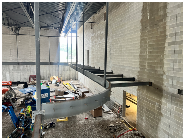
Walking Steel In Progress – Area C2 New Gymnasium
