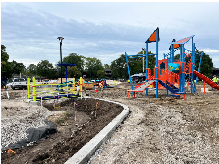
Playground Progress – Site
