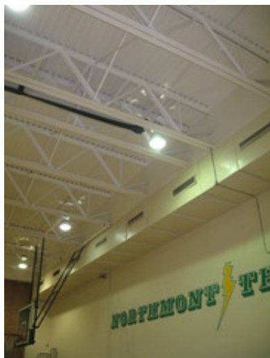
Roof Structure Over Gymnasium
