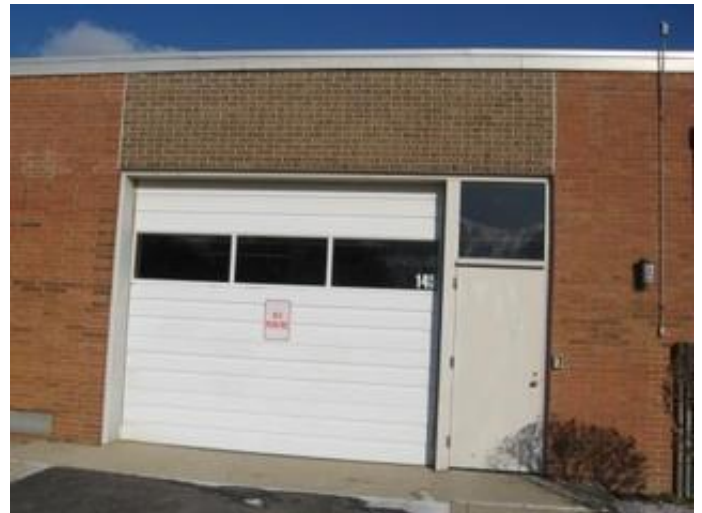
Overhead Door and Typical Exterior Door
