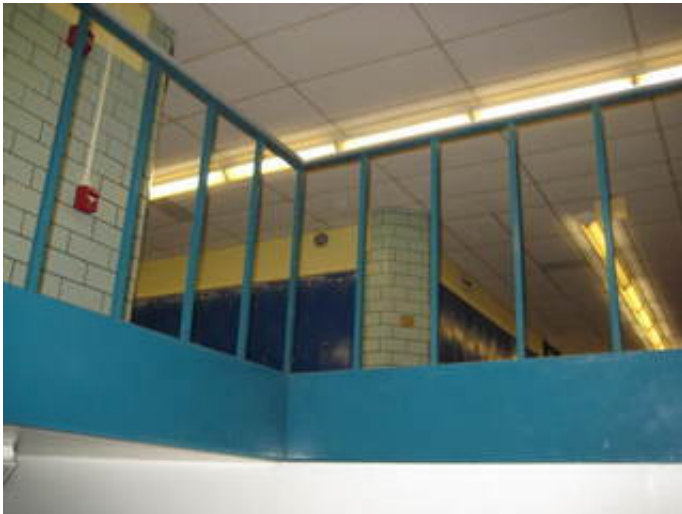
Non-compliant Guardrail
