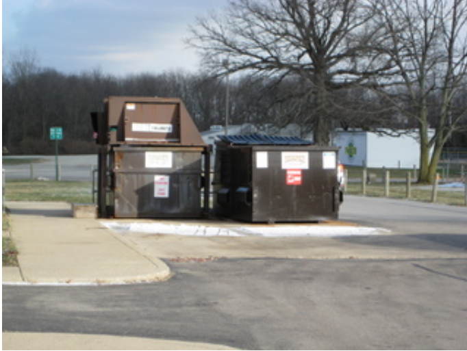
Concrete Dumpster Pad
