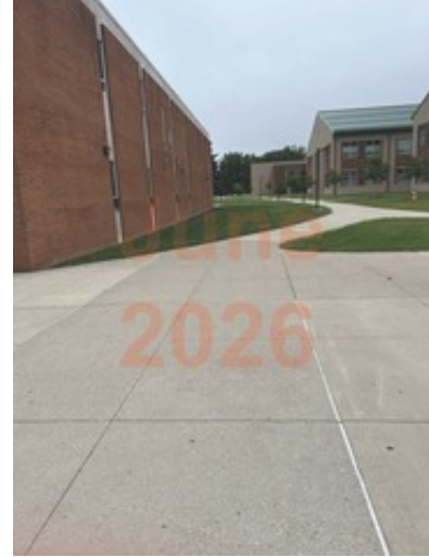
Concrete Sidewalk Conditions (2026 Photo)
