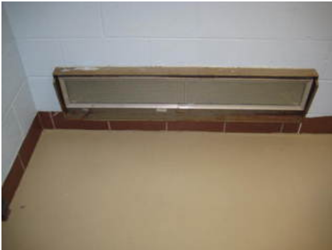
Electric Fired Radiant Glass Heater
