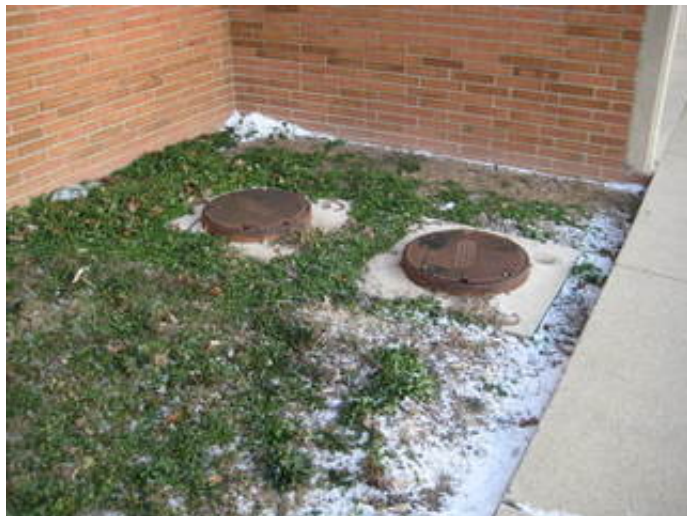
Kitchen Grease Trap Interceptor
