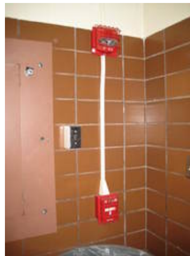
Fire Alarm System Manual Pull Station and Strobe Indicating Device
