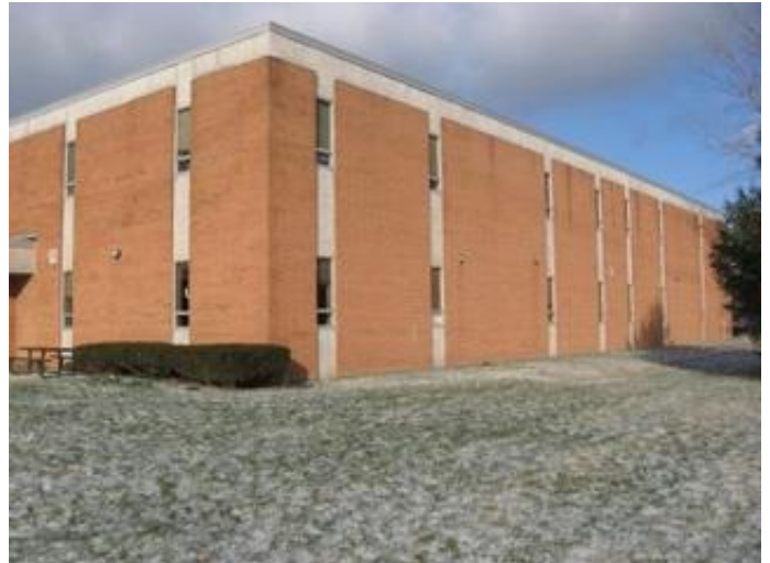
1967 Original Construction Classroom Windows
