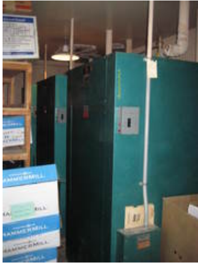
Electric Fired Domestic Water Heaters
