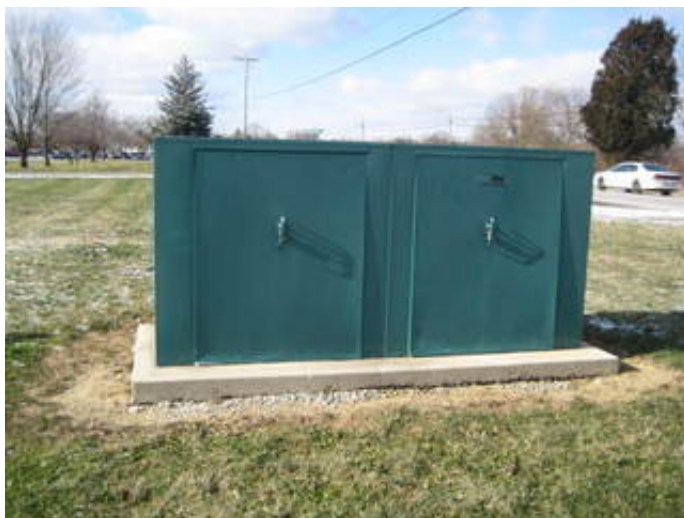
Incoming Domestic Water Service Line Shed
