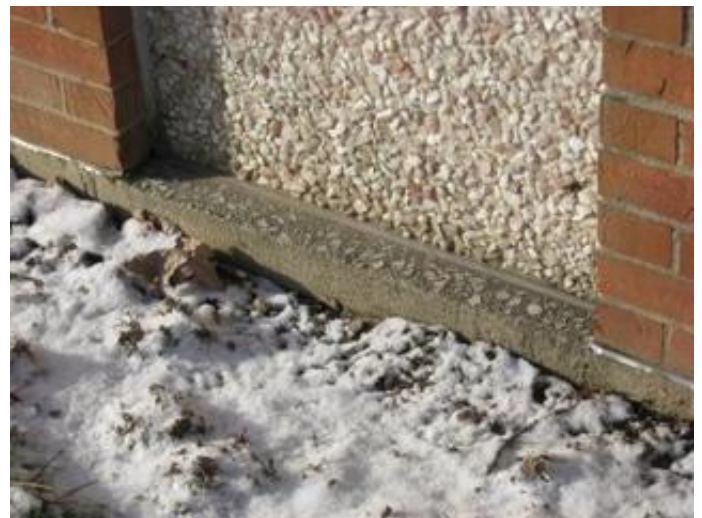
Exposed Concrete Foundation at Window Location
