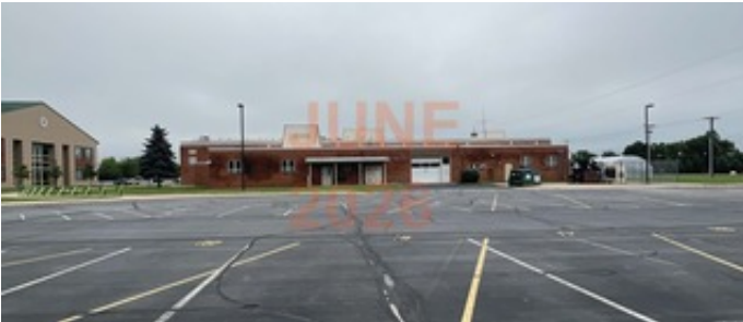
South elevation photo:
