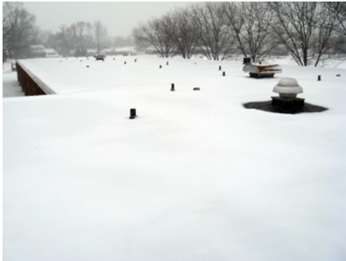
Roof Over Classroom Wing Of The 1965 Original Construction
