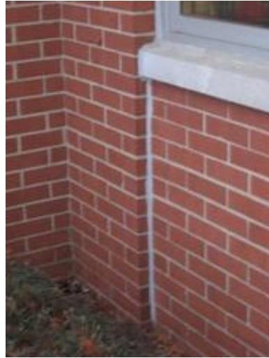
Typical Control Joint at Window Sill
