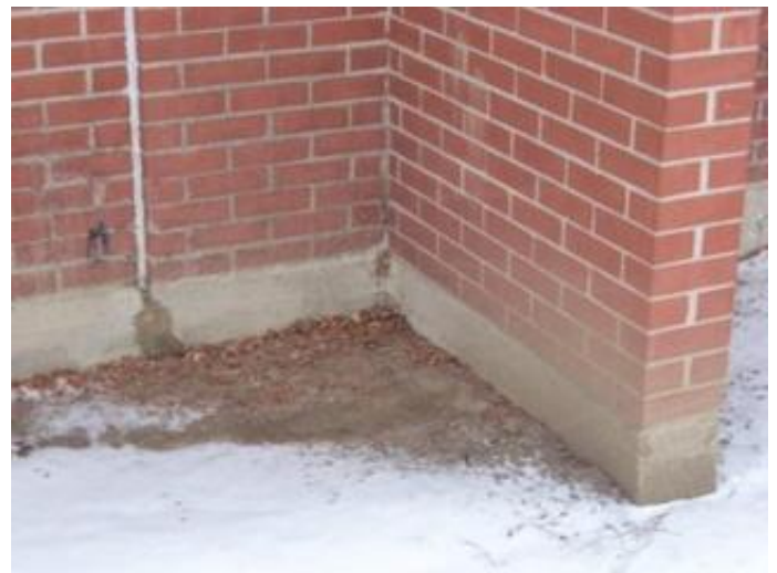
Exposed Concrete Foundation at Control Joint and Wing Wall
