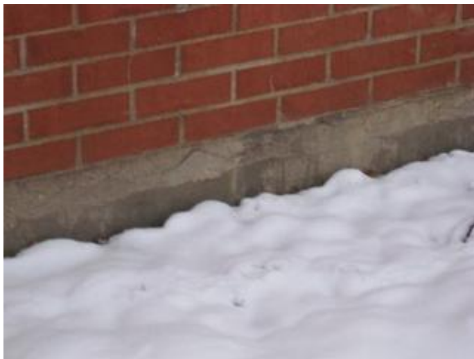
Typical Exposed Concrete Foundation Wall Condition
