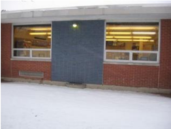
Typical Classroom Windows
