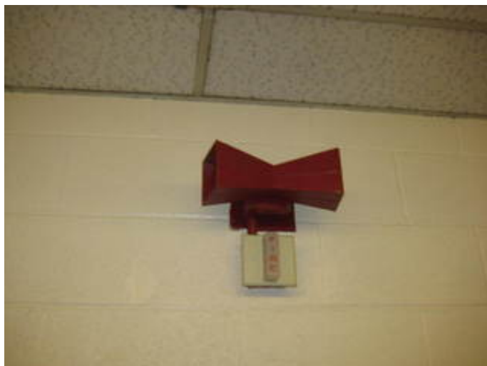
Fire Alarm System Horn and Strobe Indicating Device
