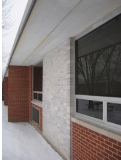
Typical Exterior Soffit Condition
