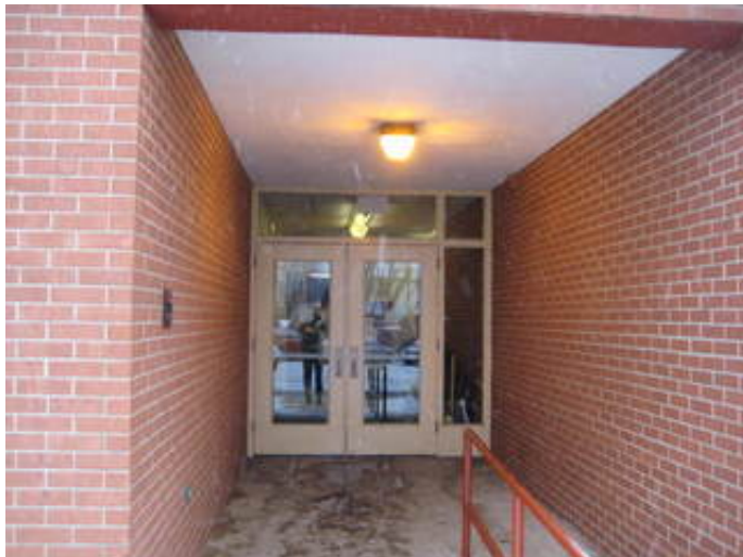
Typical Surface Mounted Light Fixture
