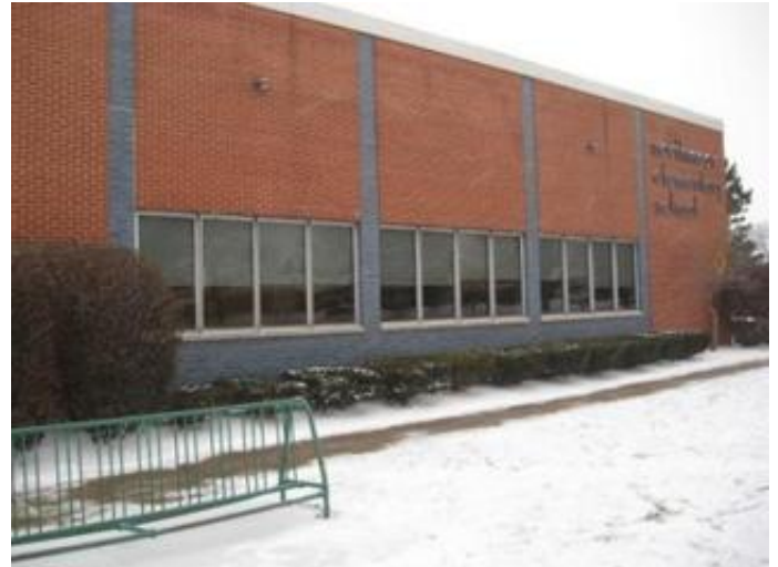
1965 Original Construction Multi Purpose Room Windows
