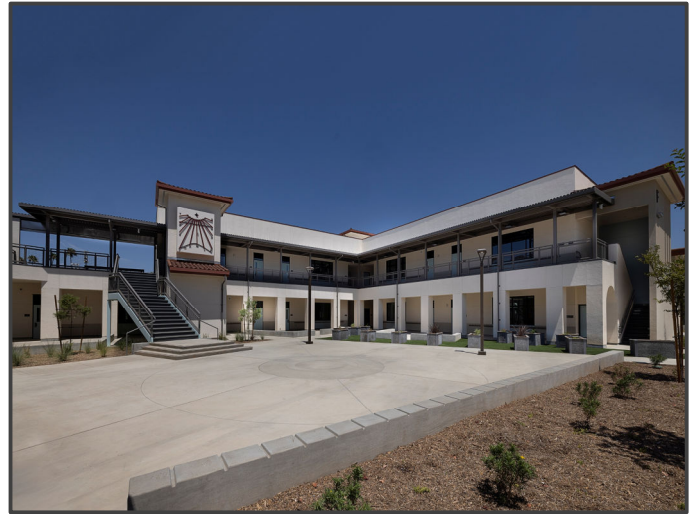
Building F – 2 Story Classroom
