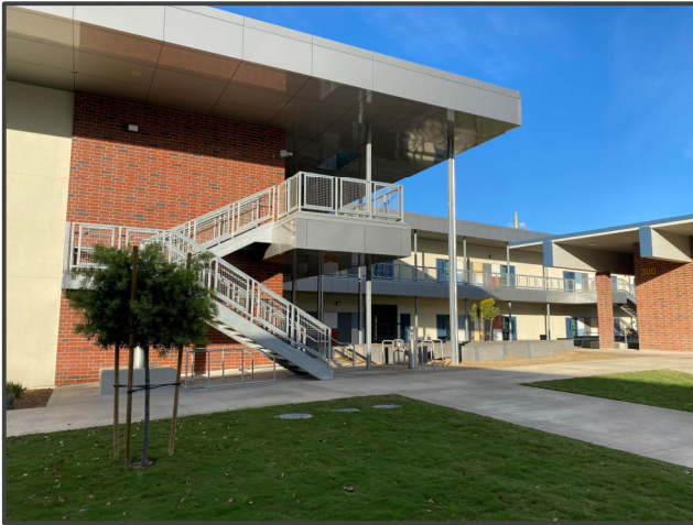
New 2-Story Classroom Building
