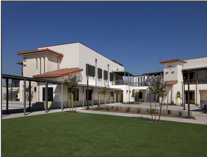
Building D – 2 Story Classroom
