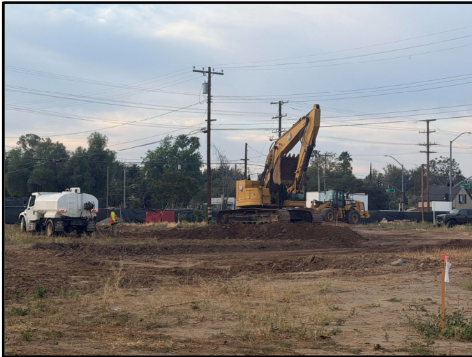
Increment 1 – Soil Mitigation Parcel C Stockpiling
