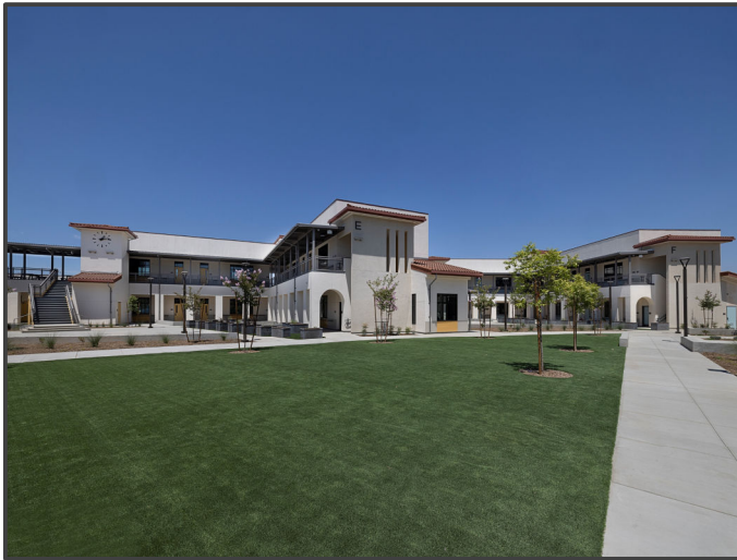
Building A & F – 2 Story Classroom
