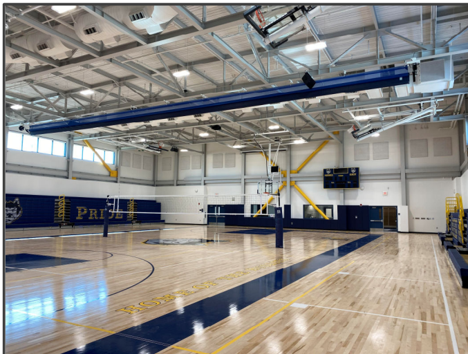
New Gym Building – Volleyball Court Set Up
