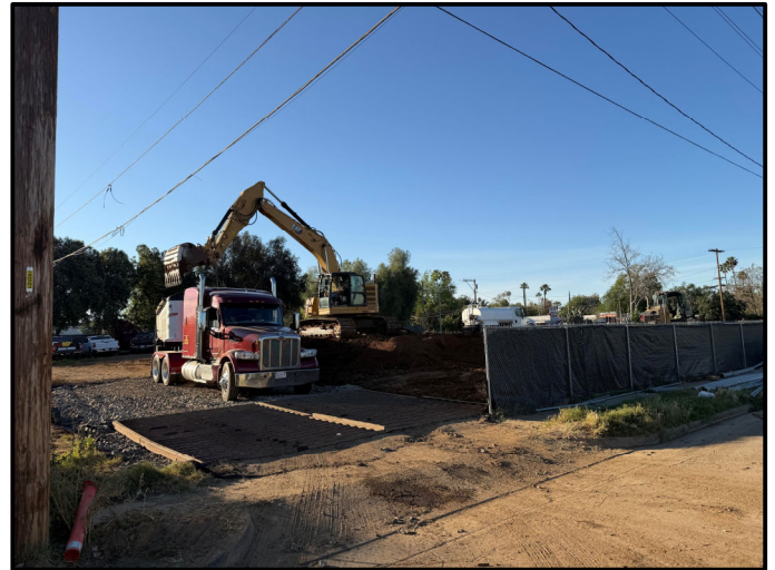
Increment 1 – Soil Mitigation Truck Loading Work
