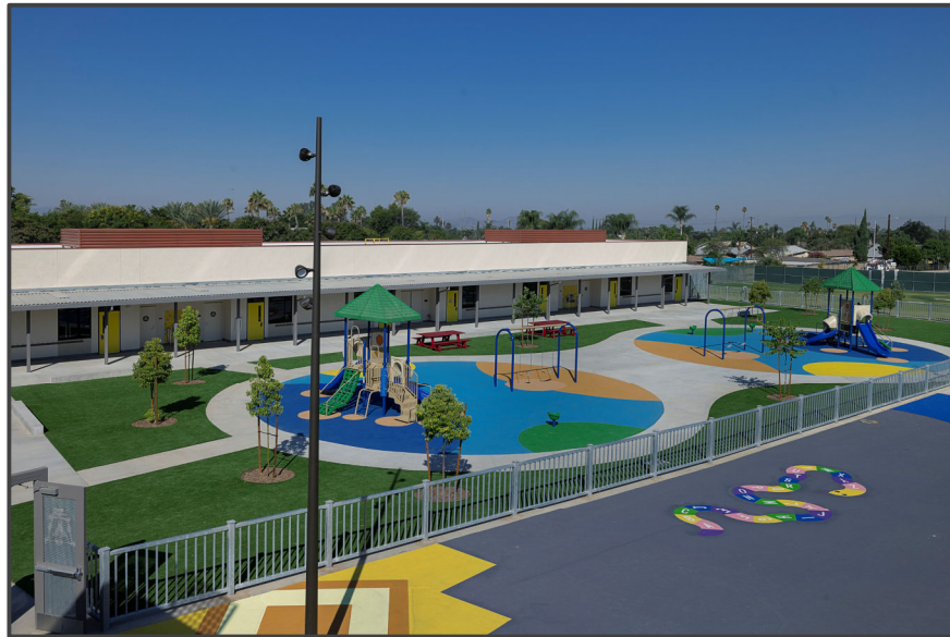
Building C – Kindergarten & Playground
