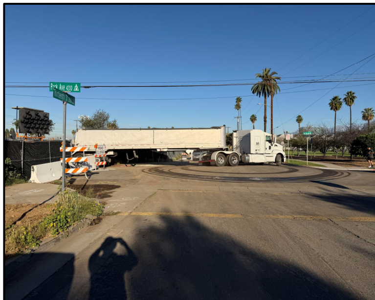
Increment 1 – Soil Mitigation Work Truck Haul Off
