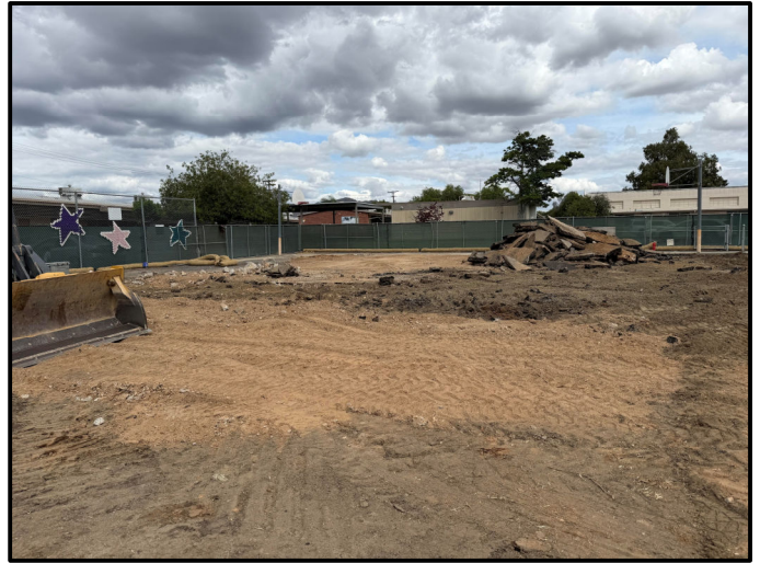
Increment 3 - Lincoln High School Asphalt Demolition
