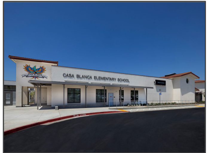
Building A - Administration Building
