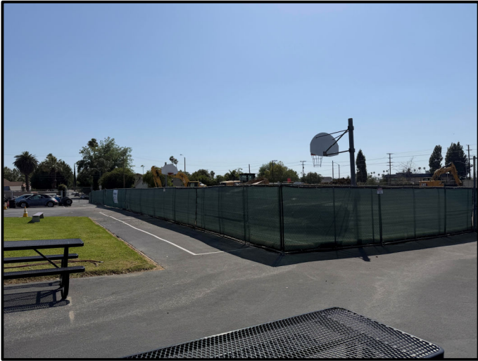
Increment 3 - Lincoln High School Temporary Fence
