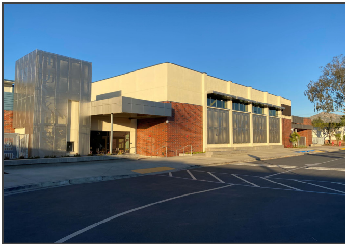
New Gym Building – Lobby Entry
