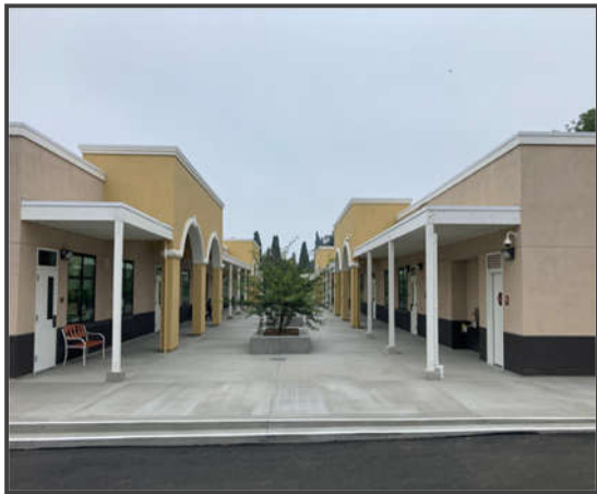
New Classroom Buildings
