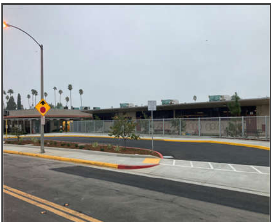
New Drop Off Area
