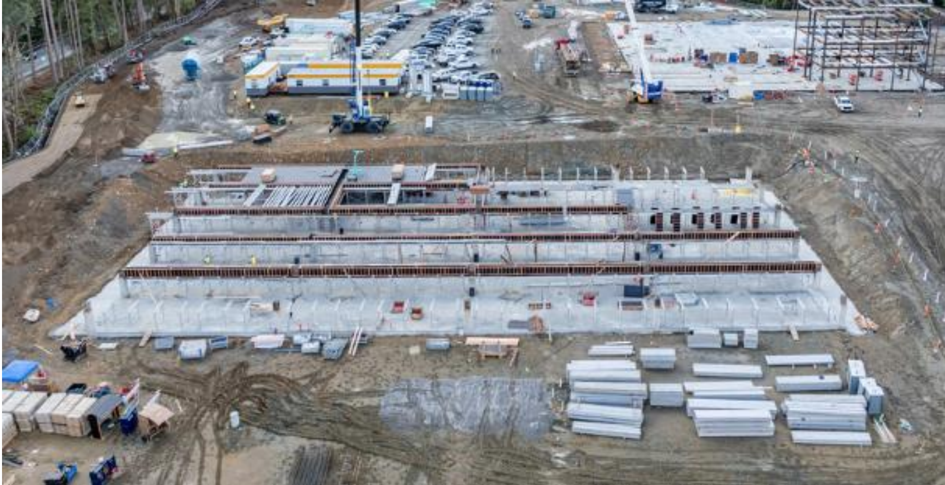
View of the parking garage slab and post-tension slab preparation underway (drone photo taken 9/14/26)
