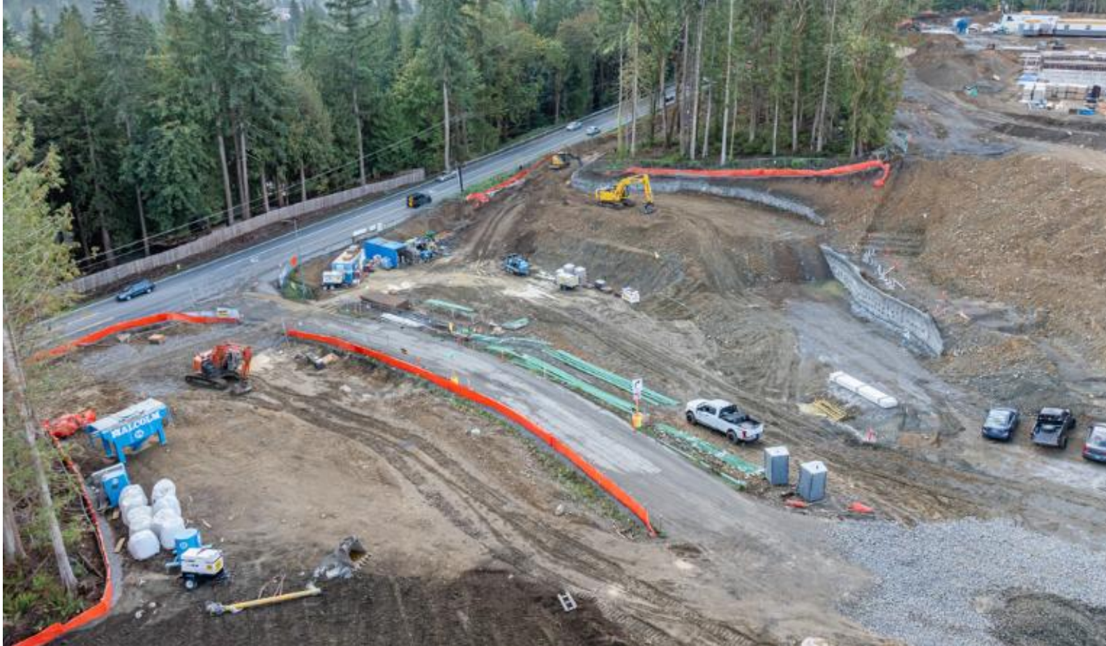
View of the main entrance being graded and retaining walls installed (drone photo taken 9/14/26)
