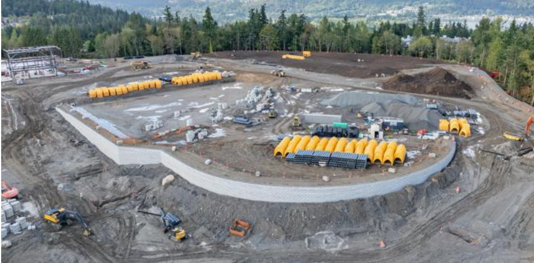
Aerial view of the future sports field area with retaining wall completed and underground storm water system being prepared (drone photo taken 9/14/26)
