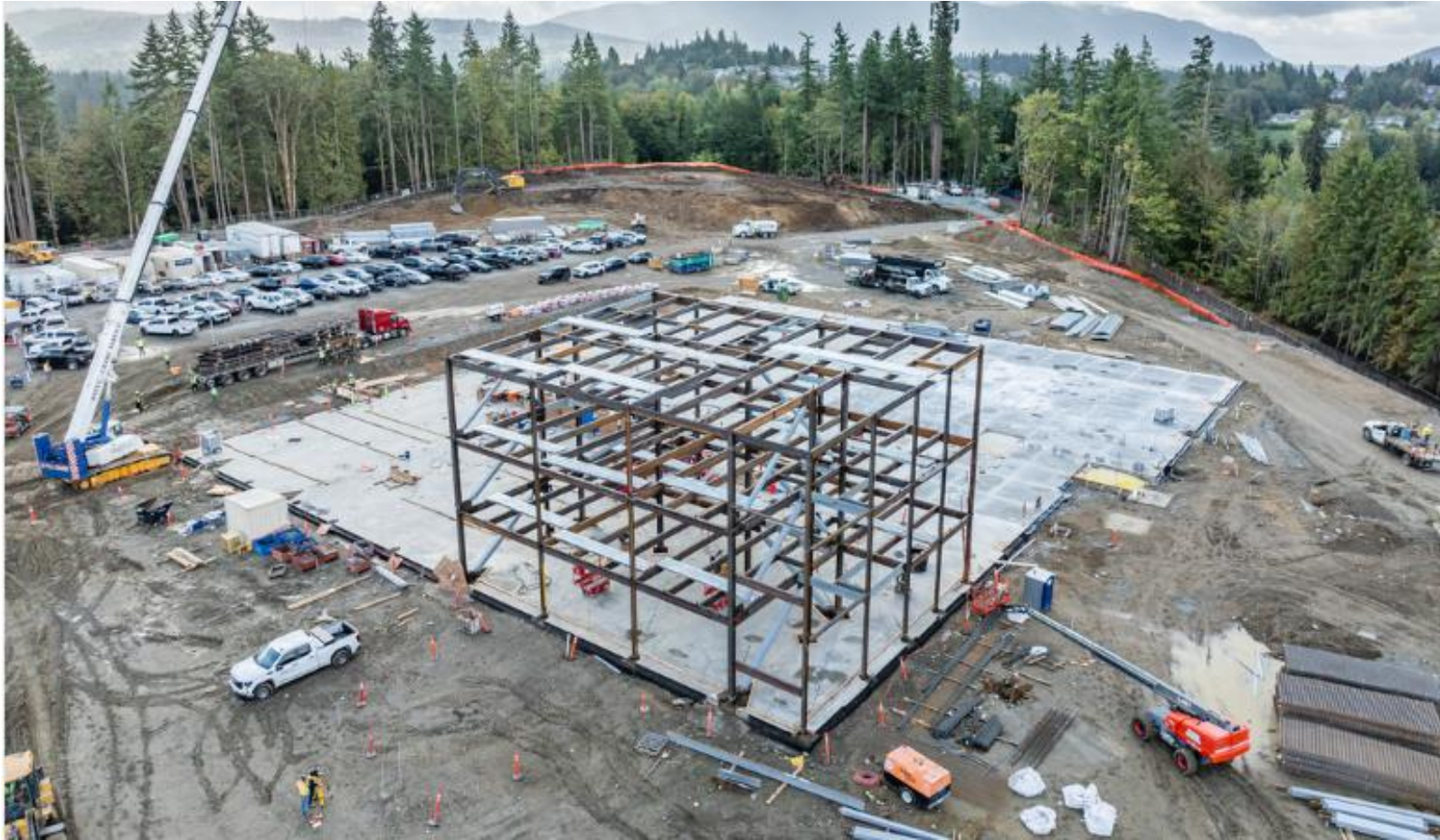
View of the main building with steel erection well underway (drone photo taken 9/14/26)
