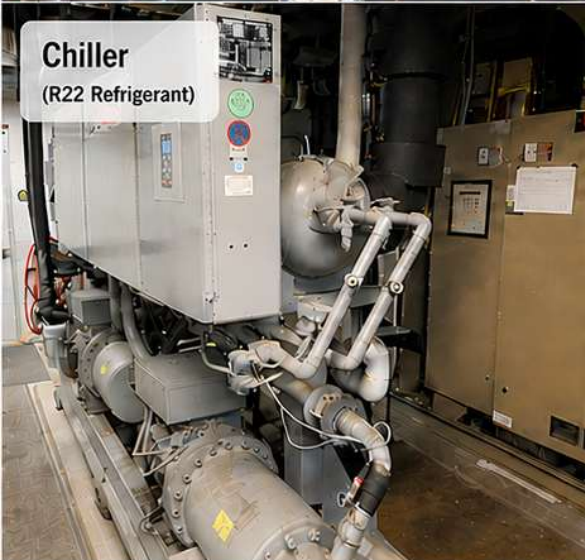
Chiller Condensing Unit
