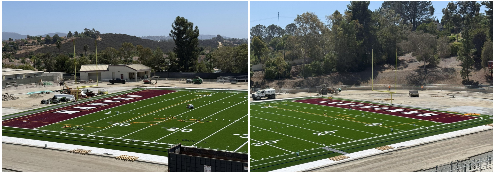
Turf Installation - Endzones
