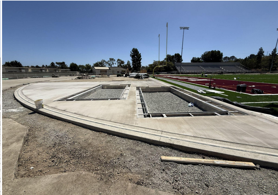
Jump Pit Installation
