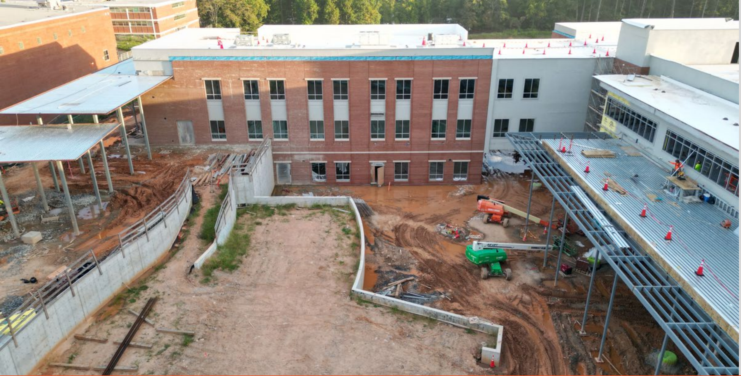
Area 2/3- Breezeway- Exterior Brick work
