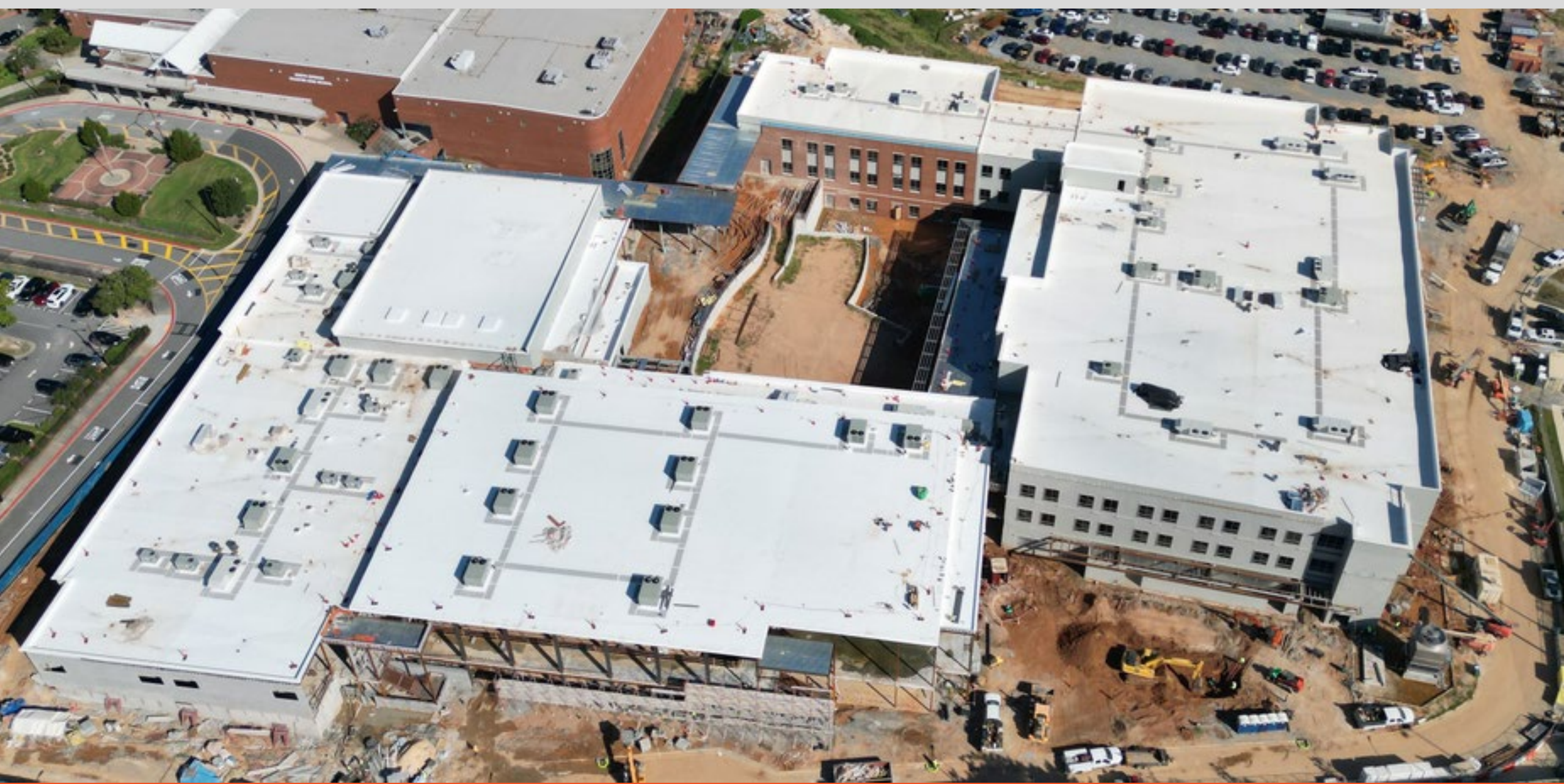
TPO Roofing complete at the new building
