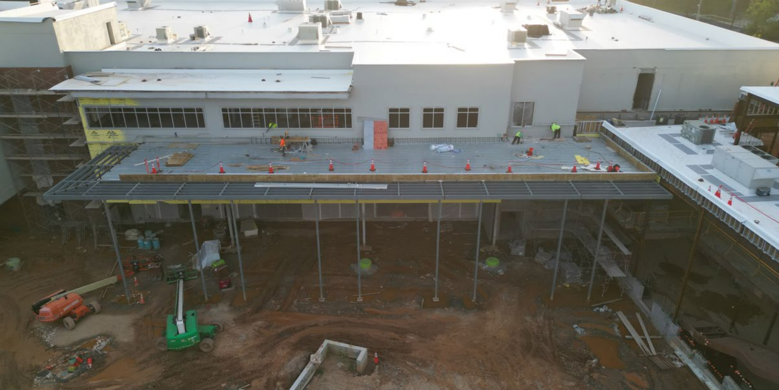
Courtyard East- Steel Canopies
