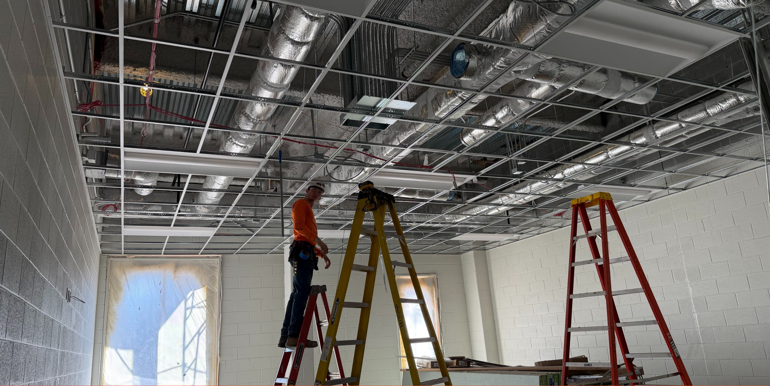
Area 3 and 4- Level 1- Ceiling Grids and Lights installation
