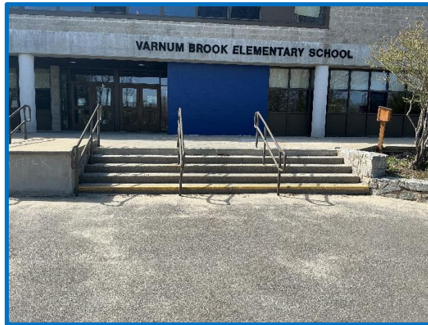
Figure 6 Varnum Brook Elementary School
