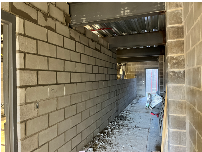
CMU Partitions Built – Area A2 Ground Level
