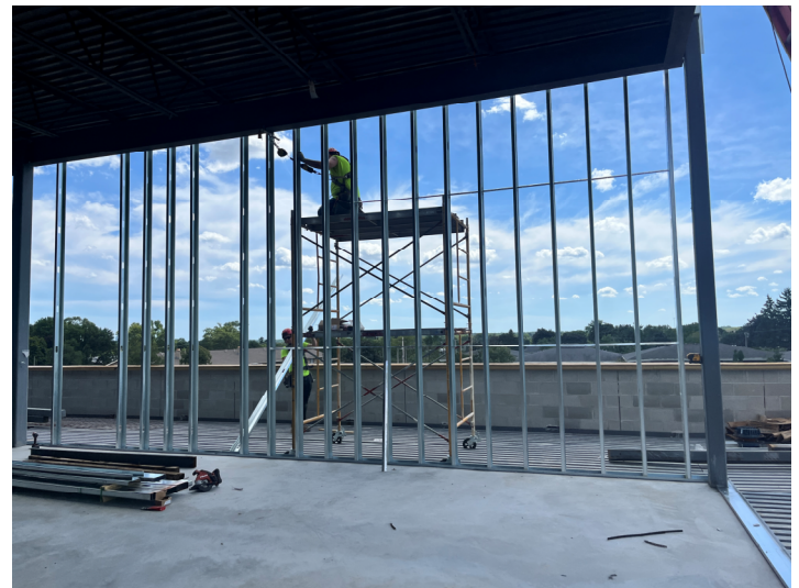
Metal Stud Framing – Area C1 2 nd Level
