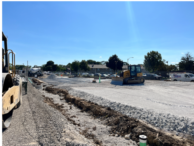
Grading Underway – Site
