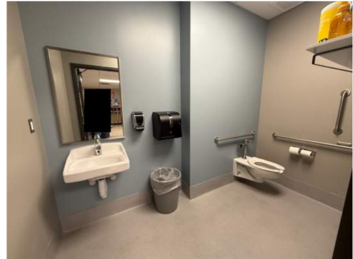
Restrooms 164a / 165a
