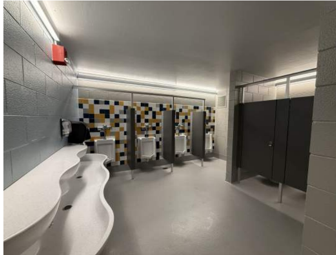
Boys 150 Restroom / Girls 151 Restroom
