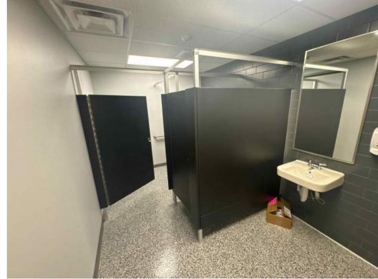
PR03 Womens Restroom
