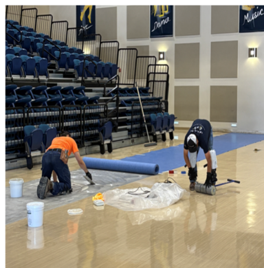
Hillview PAC Flooring Replacement
