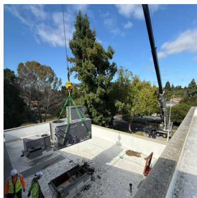
Laurel Upper HVAC Electrification
