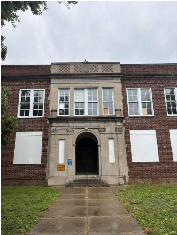
South elevation - detail of main entrance
