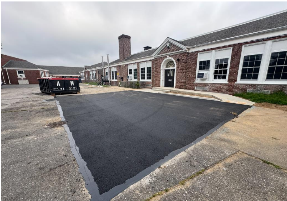
Hempstead McNeil ES – Ramp and Asphalt
