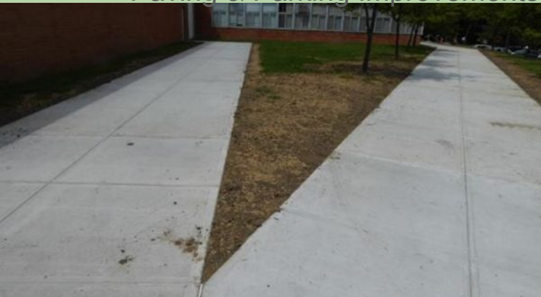
Paving & Parking Improvements
