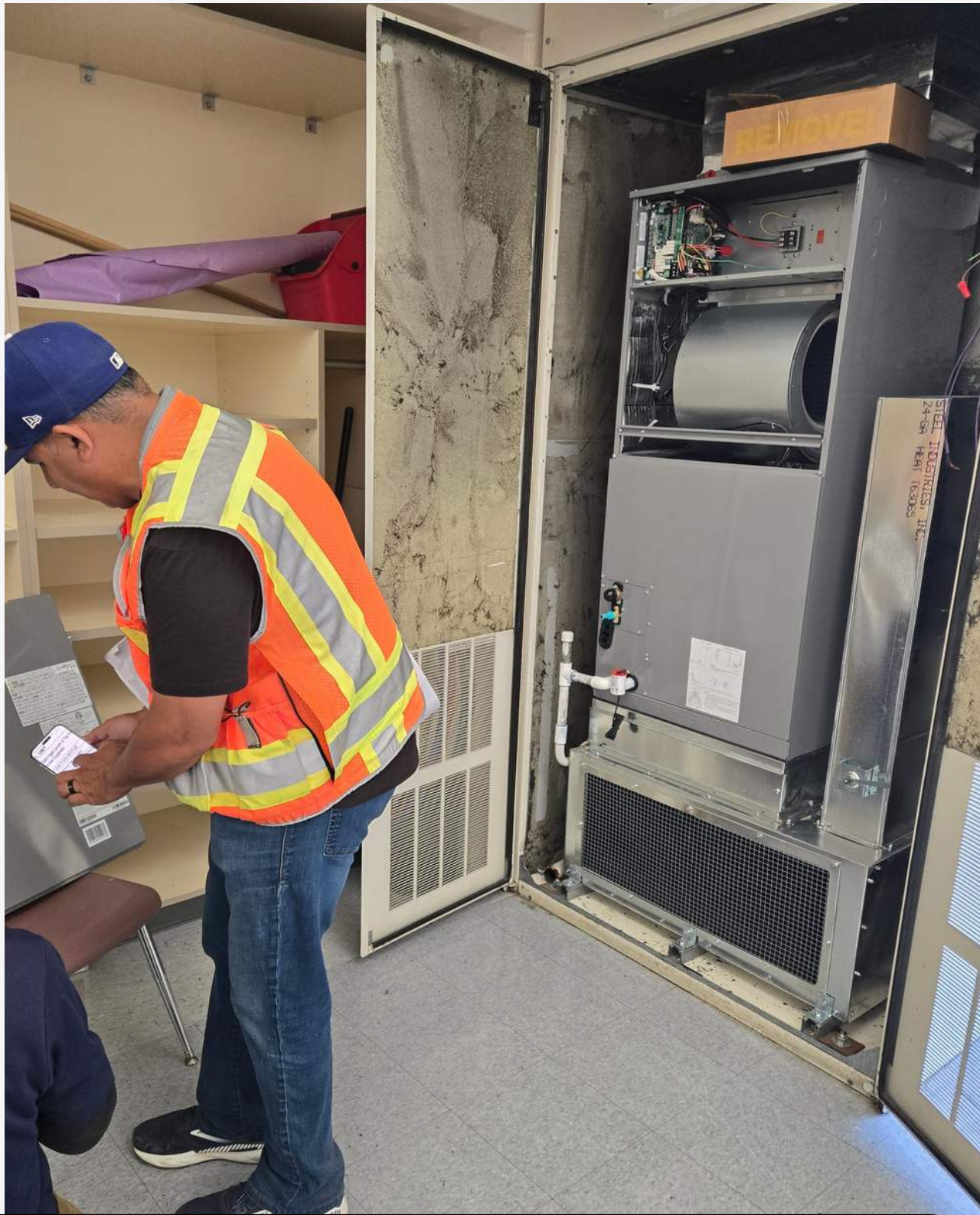
HVAC Replacement & Roofing
