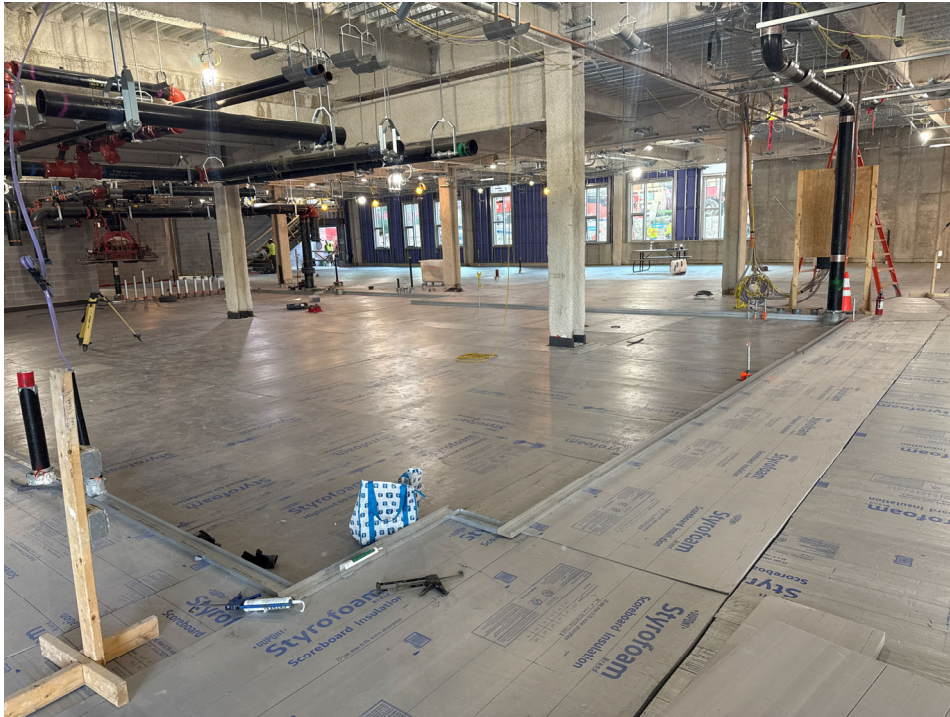
Rigid insulation for topping slab in place, Level 1
