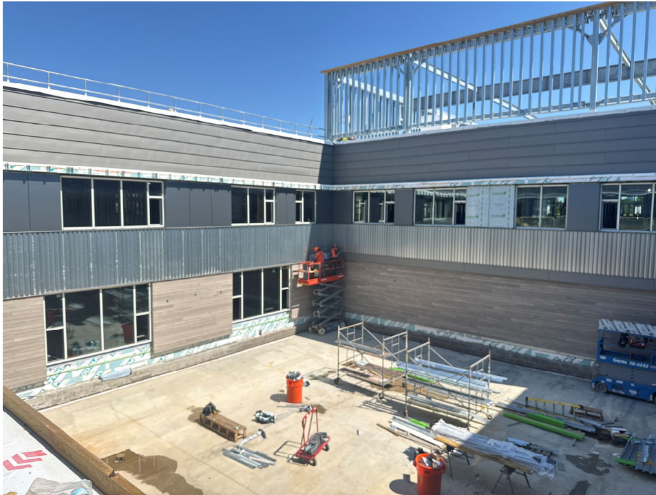
View of courtyard progress – Accoya wood, zinc panels
