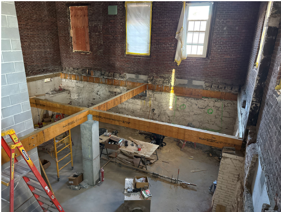
Framing for new floor at Historic Building elevator area
