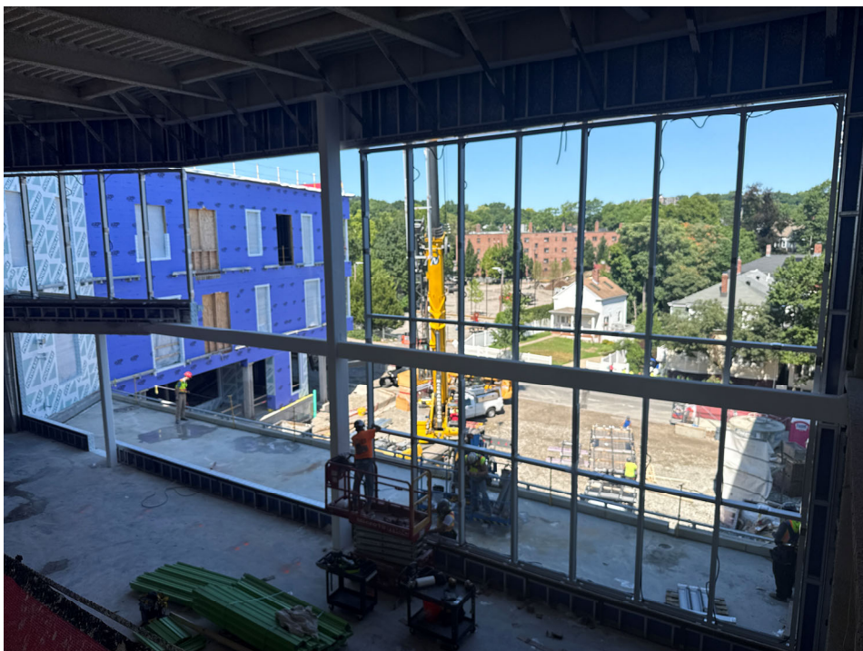
Curtainwall installation, West (Library) elevation
