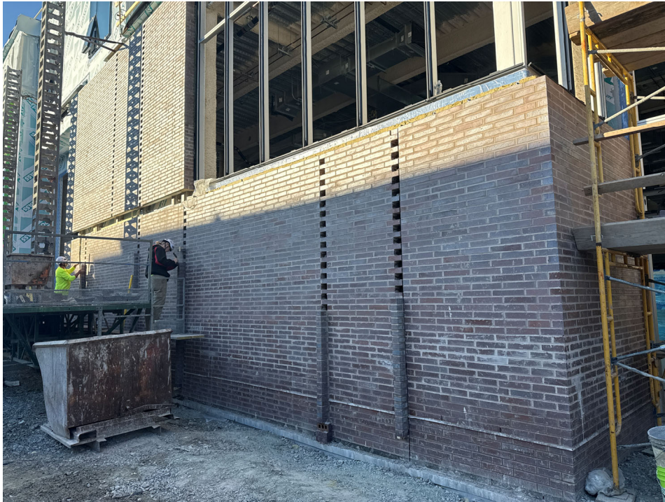
North elevation brick, including fins
