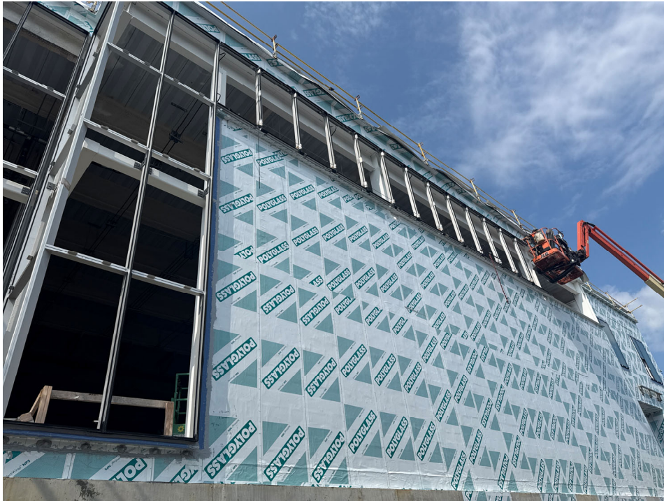
Curtainwall progress, North elevation
