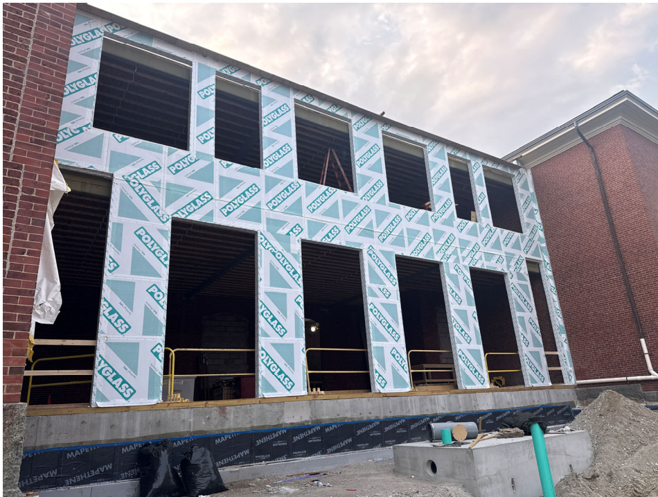
Exterior of Historic Building addition
