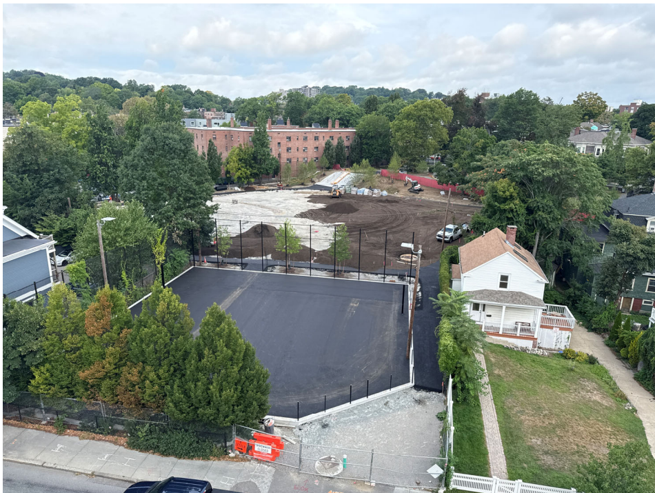
Pierce Park – loam placement in progress.
