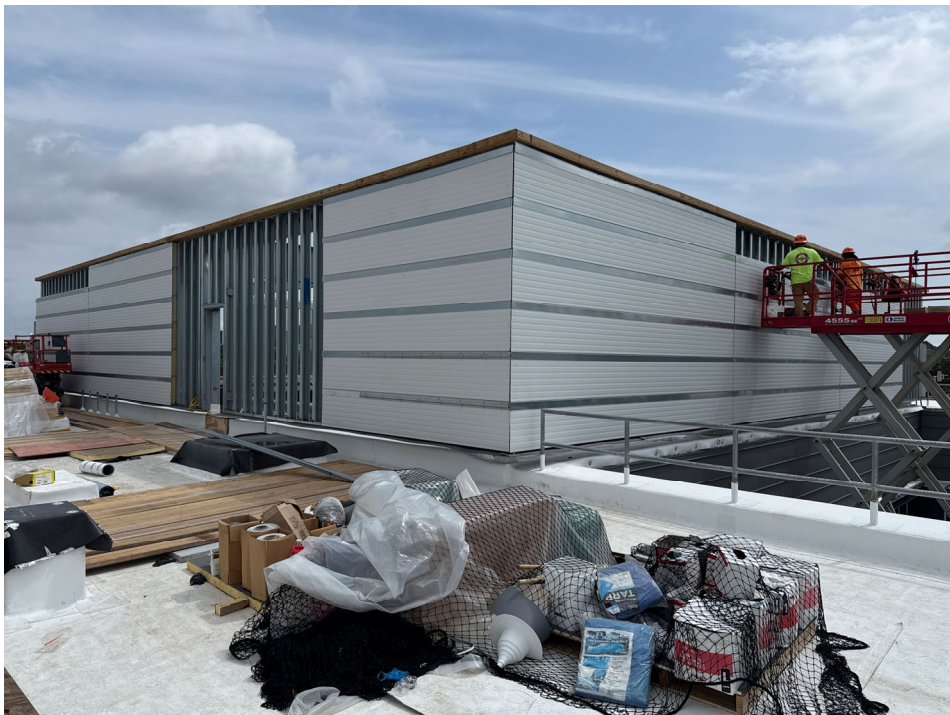
Insulated metal panels at MEP area, Building A roof
