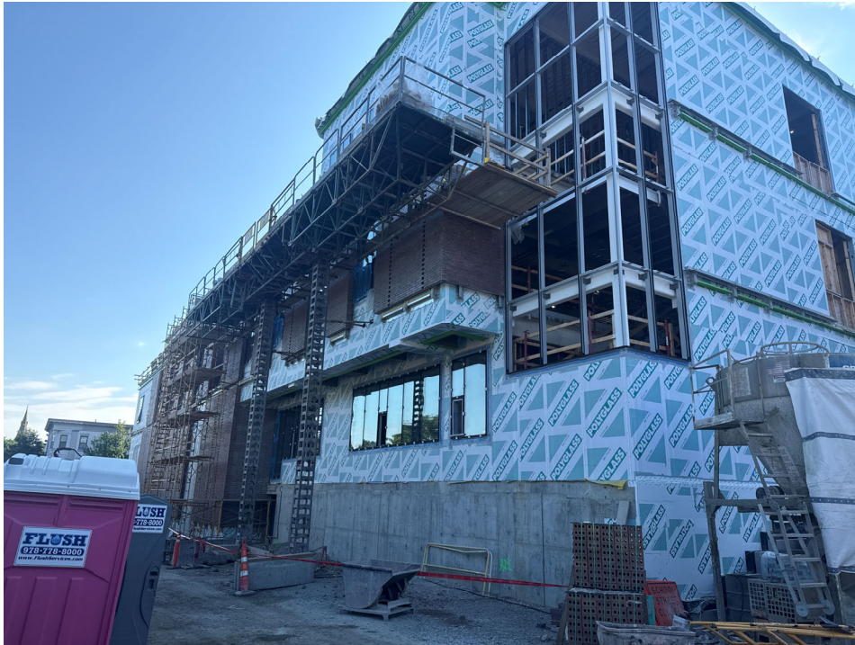
West elevation progress – brick, curtainwall
