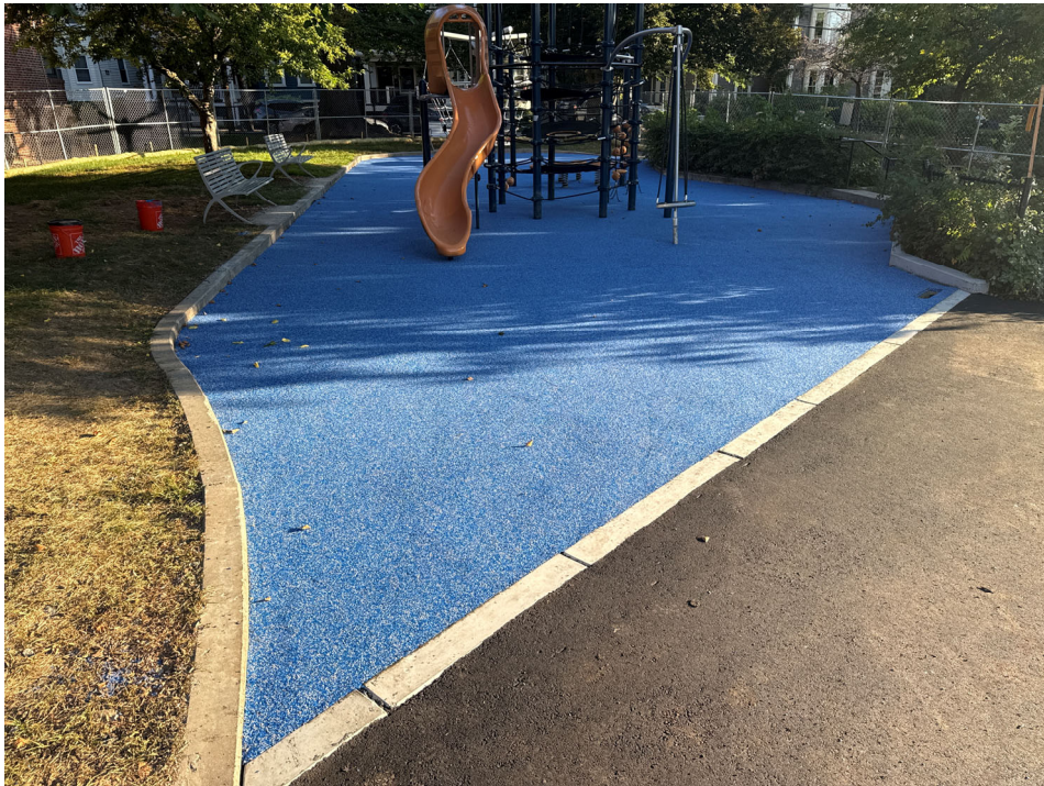
Upper playground, play surface completed.
