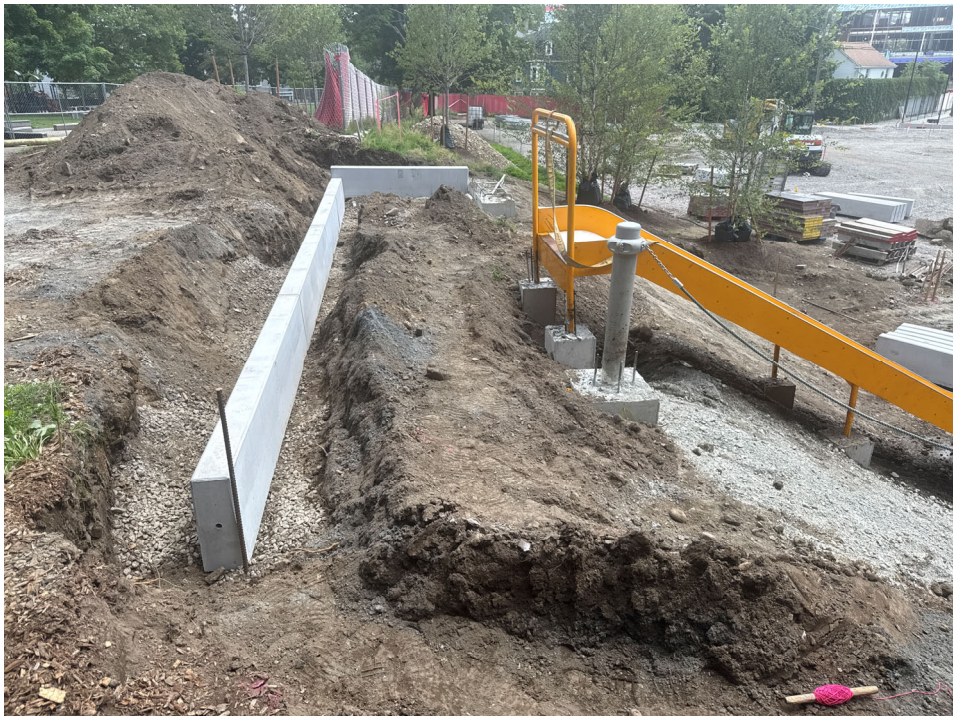
Precast concrete curb at top of slide, Pierce Park.
