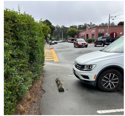
Figure 3. ADA accessibility issues behind the perpendicular parking on Miramontes St.
