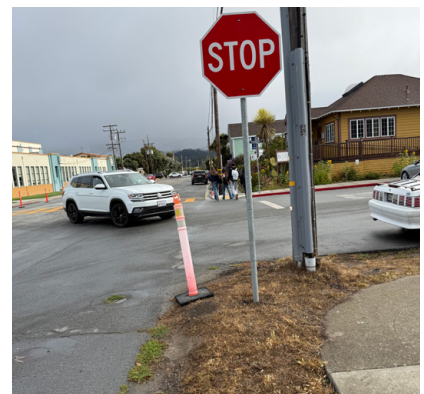
Figure 9. Missing curb ramp at the southeast corner of Church St/ Miramontes St.
