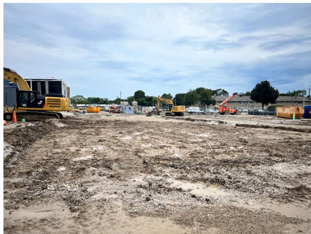
Grading Underway – Site
