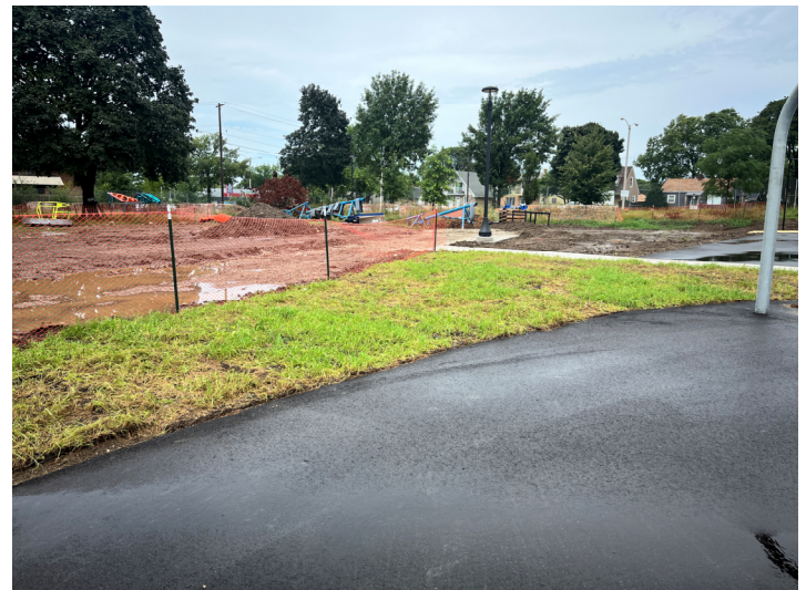
Vegetative Mat Laid – Site
