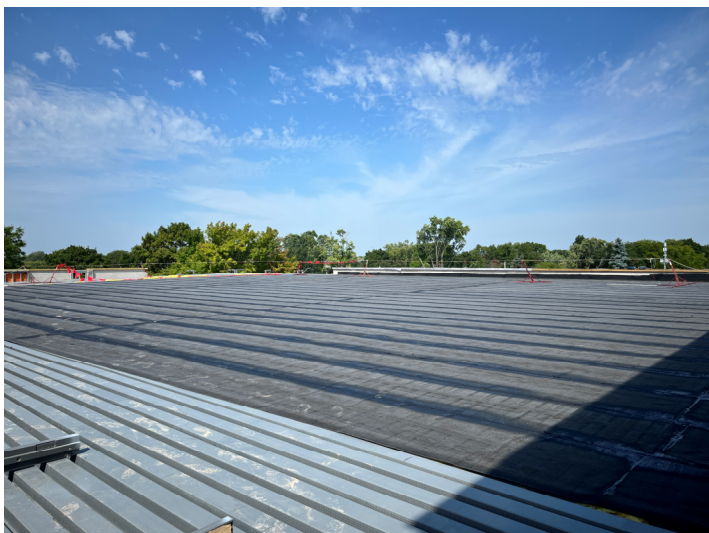
Roofing In Progress – Area C2 Gymnasium
