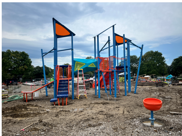
Assembling Playground Equipment – Site
